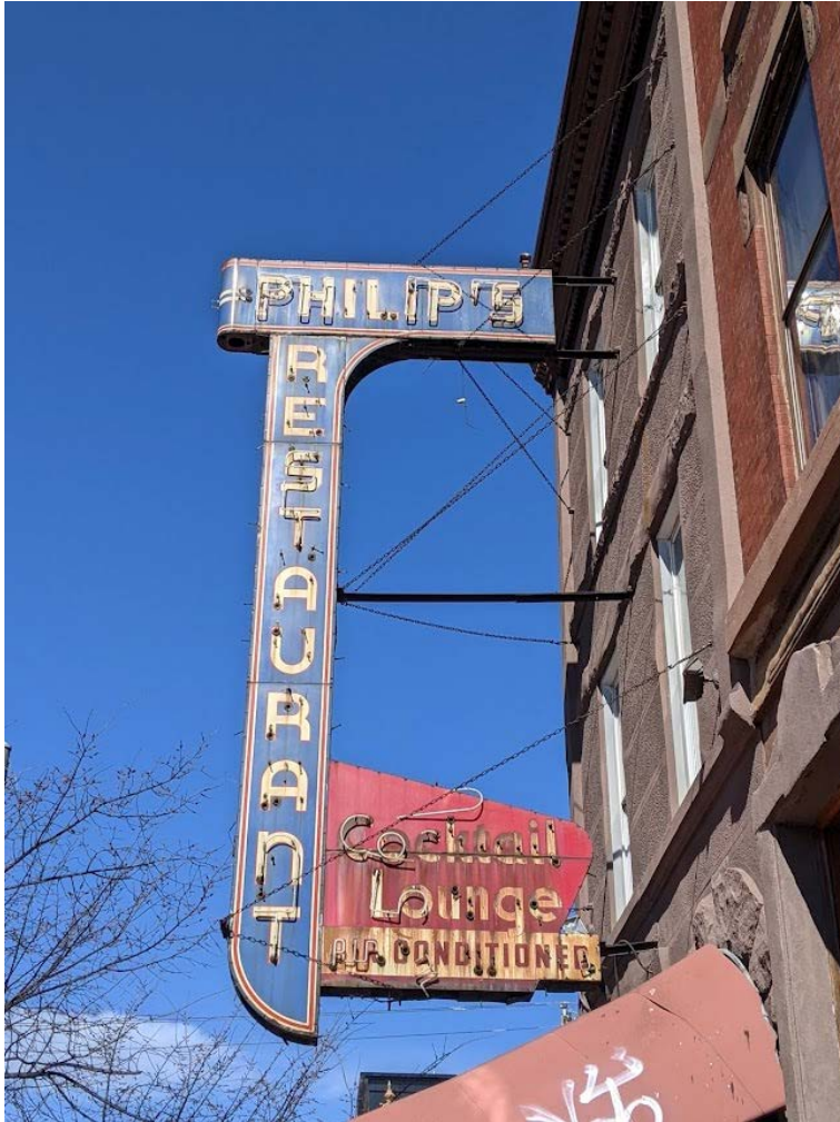
Figure 3. Photograph of the Philips Restaurant neon sign's southern face, at 1145 S. Broad Street, visible from the Boot N Saddle bar across Ellsworth Street. The sign has degraded over time, as clear from the rusting along the painted steel façade.
