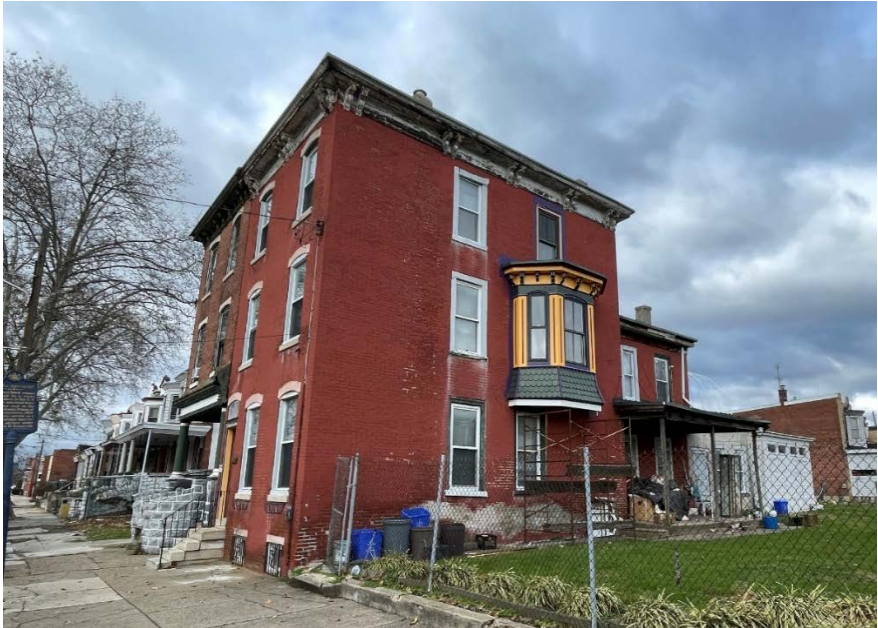
Figure 3. Southeast corner of 5401-03 Vine Street, Philadelphia, December 2022. Photo by Ted Maust.
