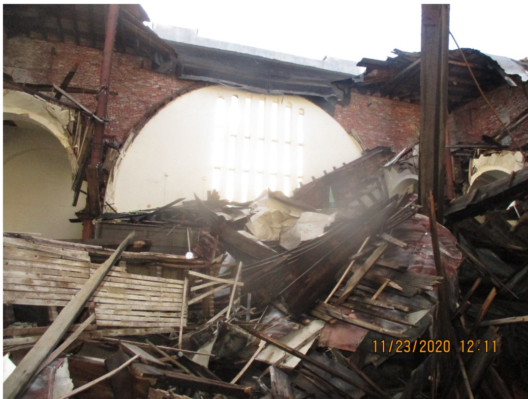
L&I photographs showing dome collapsed into the interior.
