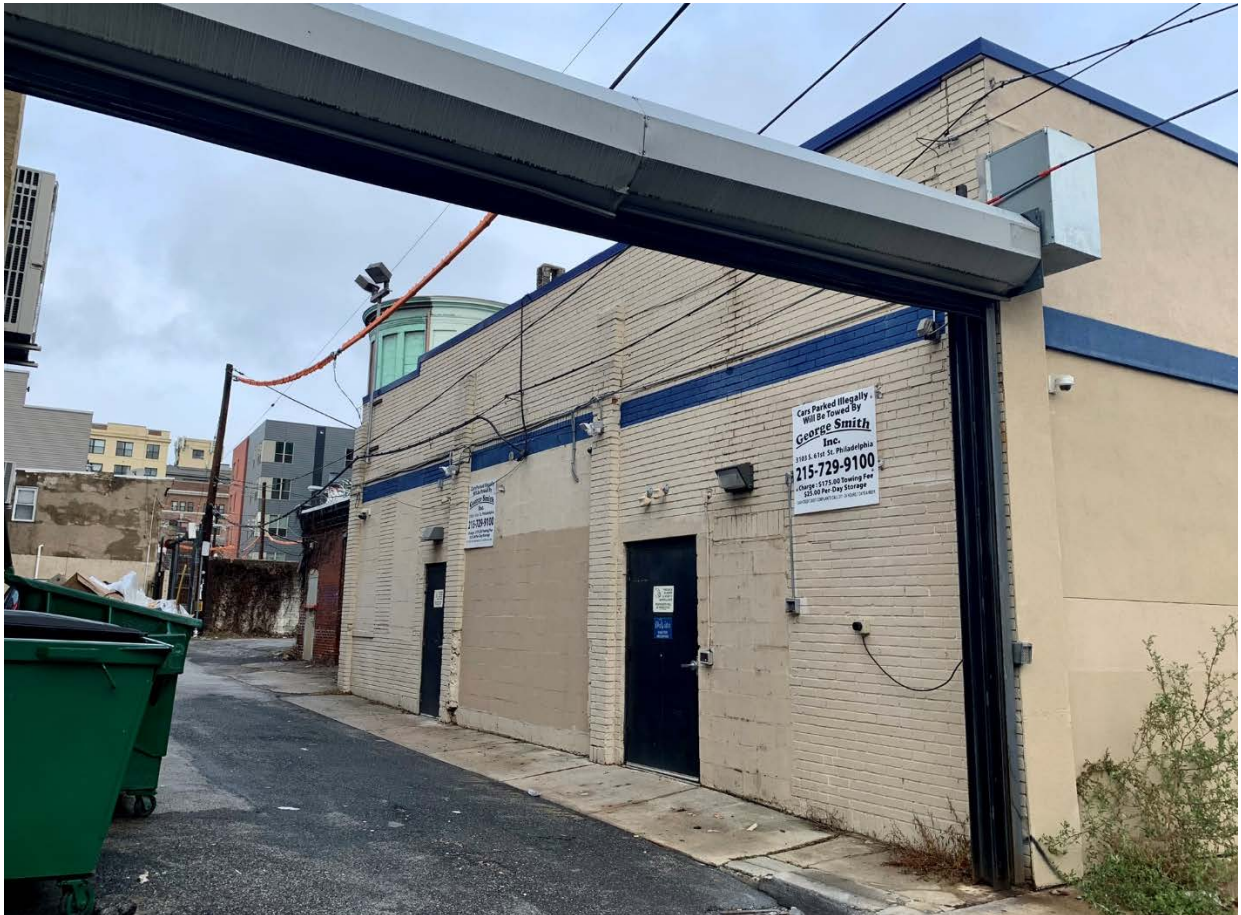
Figure 6. Rear (west) elevation, December 2022.
