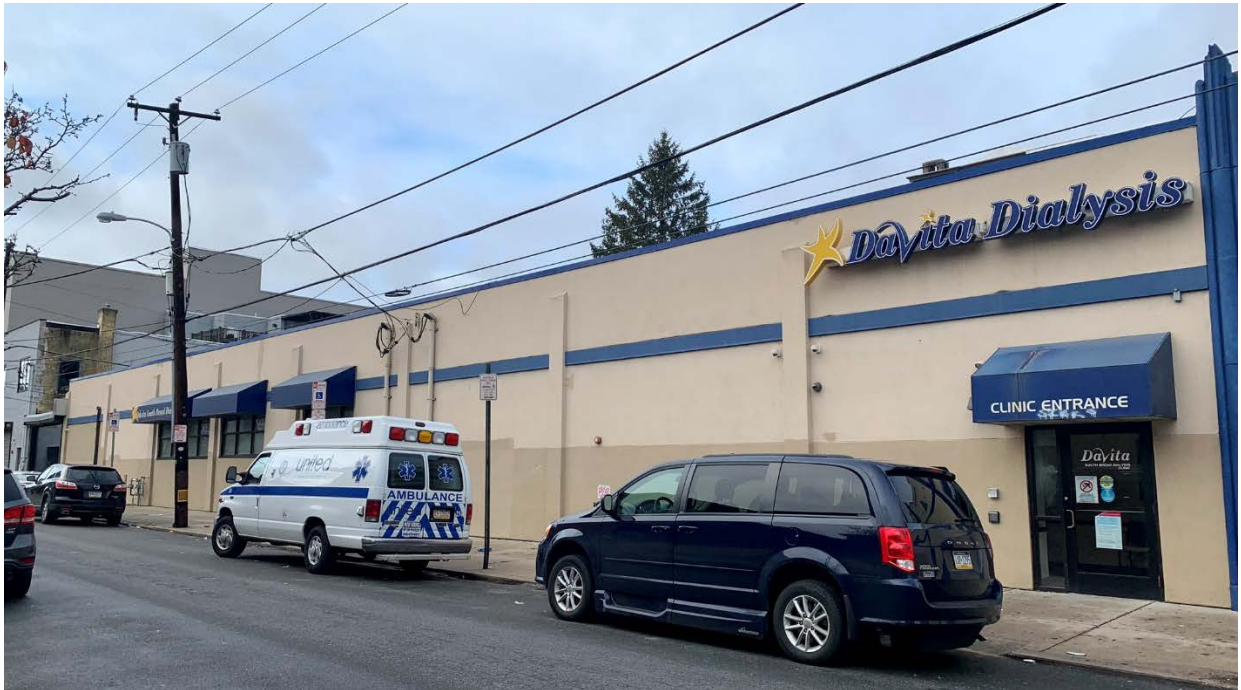
Figure 5. Service department section of the Federal Street elevation, December 2022.
