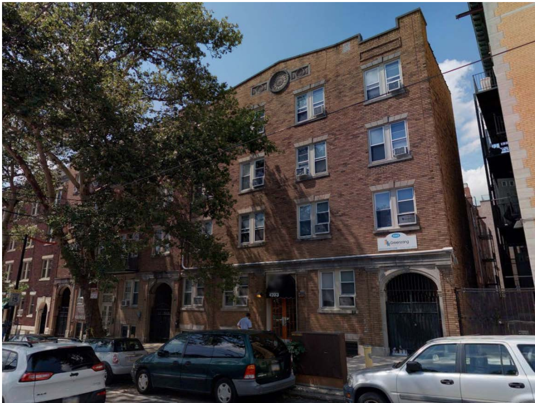
Figure 22. Waltonia Apartments, 4203 Chester Avenue. Source: Cyclomedia, 2019.
