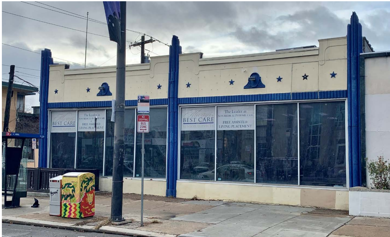
Figure 2. South Broad Street (east) elevation, December 2022.
