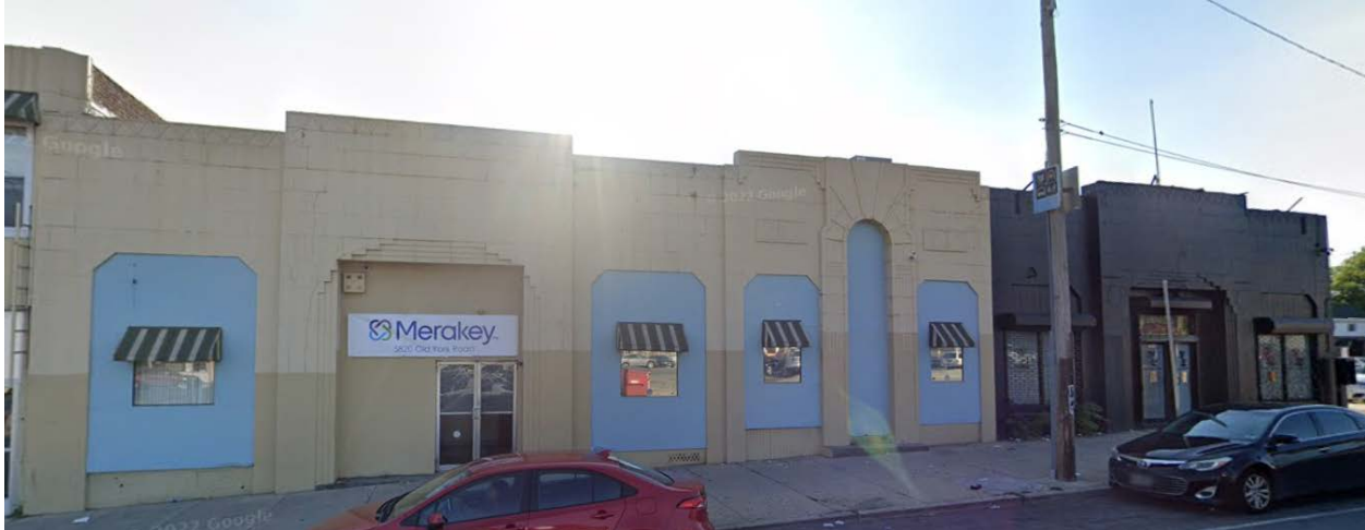
Figure 20. Karl Otto's automobile showroom at 5820-28 and 5830-32 Old York Road, constructed in 1930. Source: Google Street View.
