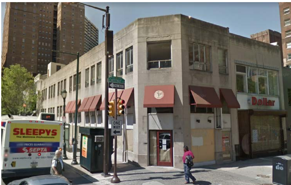
Figure 18. Frank E. Hahn's 1935 store and office for Raymond Pace Alexander, 1900 Chestnut Street. Source: Google Street View.
