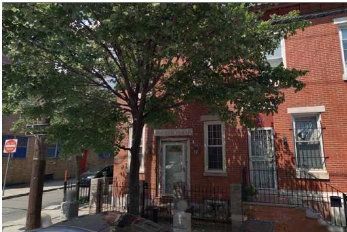
Figure 27. Koharliker Beneficial Association clubhouse, 1824 S 6 th Street. Hebrew text remains above doorway. Source: Cyclomedia, 2019.
