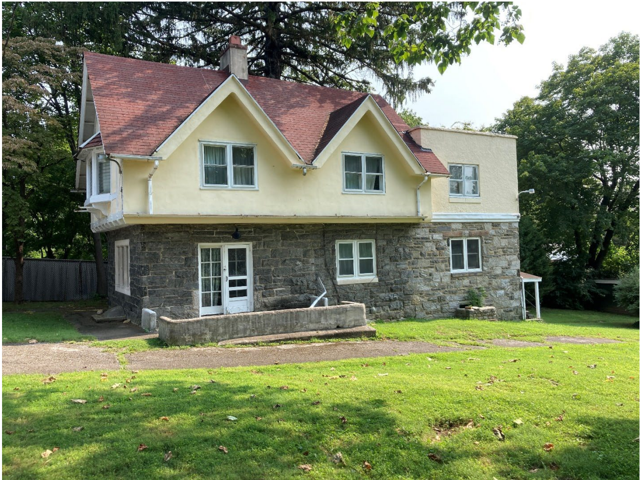
Figure 19: September 2022 photograph showing the existing conditions of the cherry cottage. View looking east.
