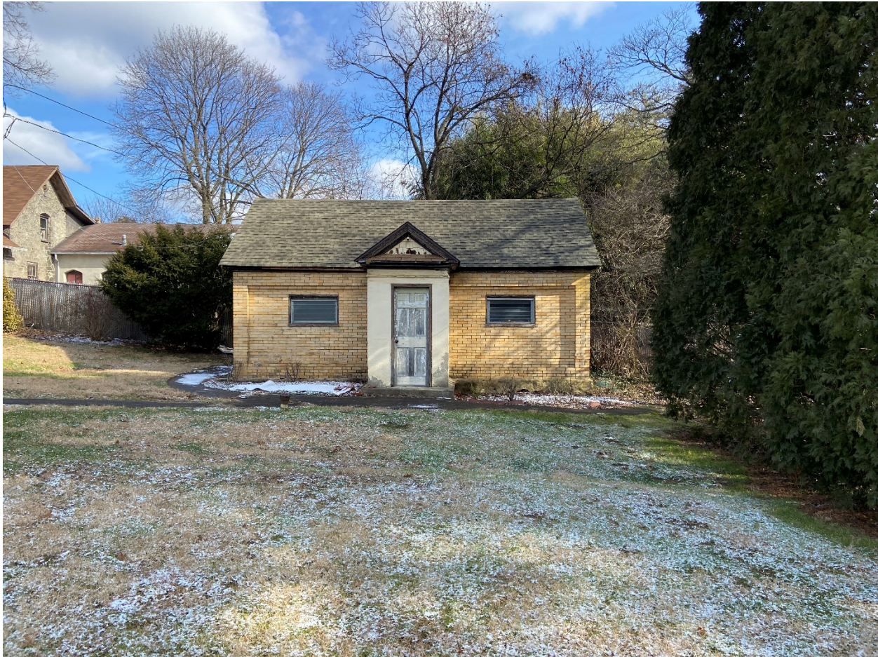
Site visit photograph, Garage/Storage Building (c1900-10)
