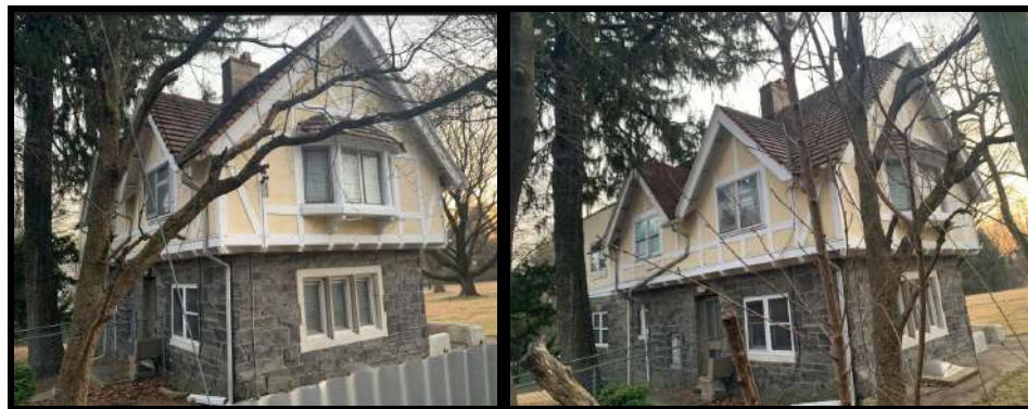
Figure 75. Left: The primary (northeast) and side (northwest) elevations of Cherry Cottage. Figure 76. Right: The primary (northeast) and side (northwest) elevations of Cherry Cottage. Source: Oscar Beisert, 2019.
