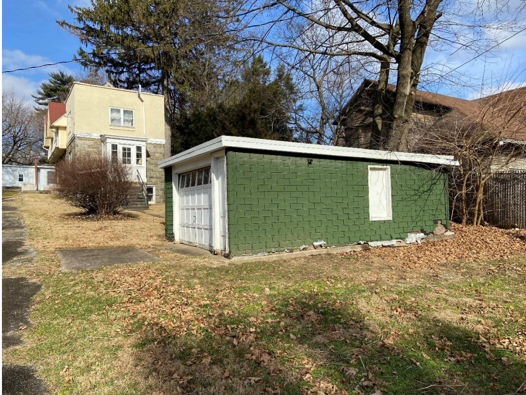
Site visit photograph, Ancillary Building
