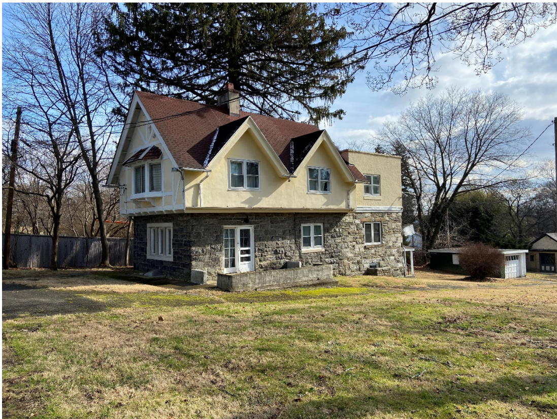
Site visit photograph, the building incorrectly referred to as the Cherry Cottage in the nomination.
