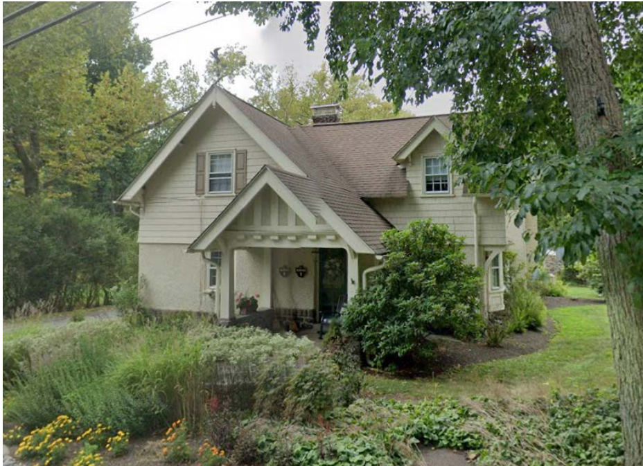
This building at Cherry Cottage in Devon is very much in the style of William Price.
