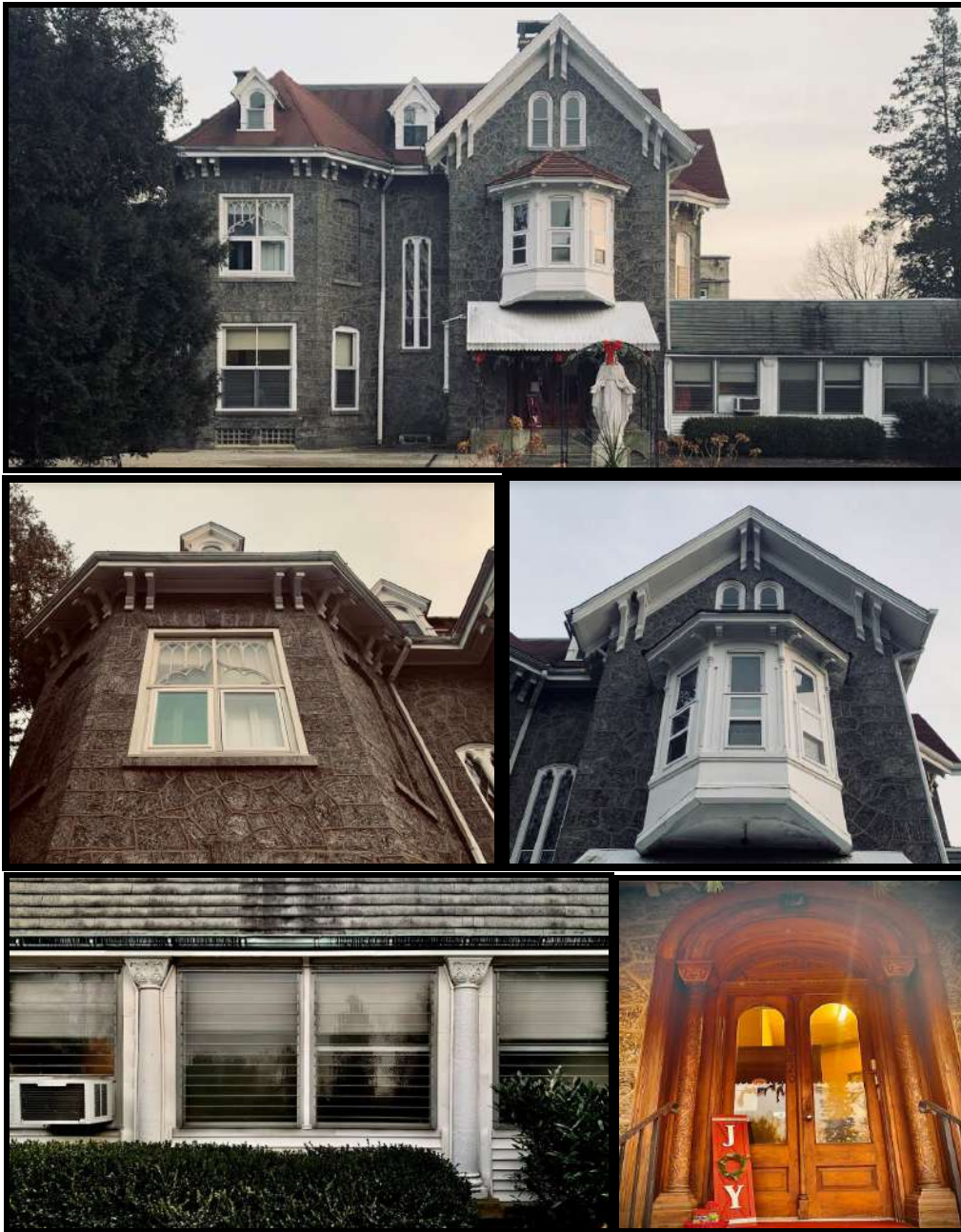
Figure 47. Top: The primary (northwest) elevation of the Main Block. Figure 48. Middle left and Figure 49. right: Details of the primary (northwest) elevation of the Main Block. Source: Oscar Beisert, 2019. Figure 50. Bottom left: The primary (northwest) elevation of the Porch Addition to the Main Block, showing the columns and cushion capitals with Norman architectural details of the porch addition. Figure 51. Bottom right: The primary entrance within the primary (northwest) elevation of the Main Block, showing similar columns and cushion capitals with Norman architectural details to the porch. Source: Oscar Beisert, 2019.
