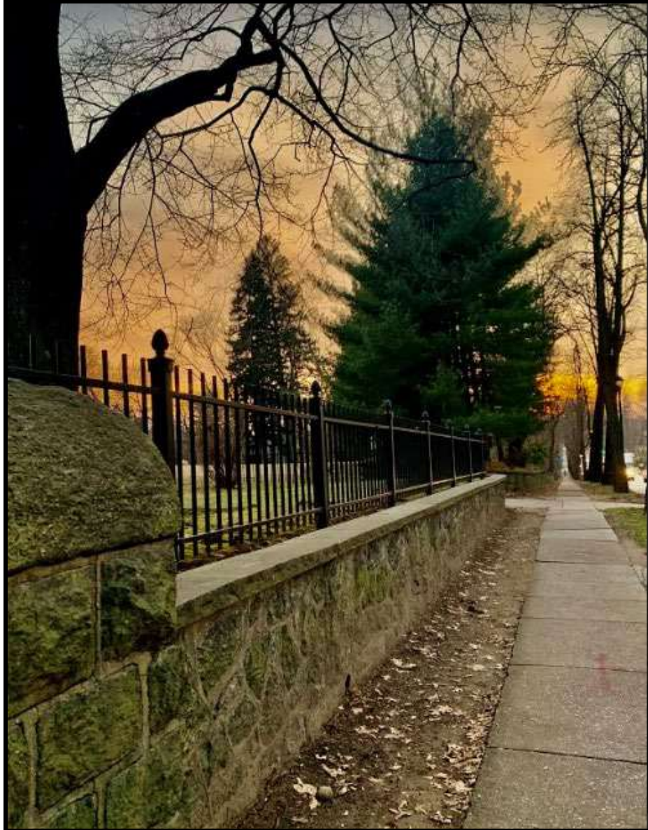
Figure 18. Looking southwest at the stone curbing and wall along City Avenue at the northwest property line of the subject property. Source: Oscar Beisert, 2019.
