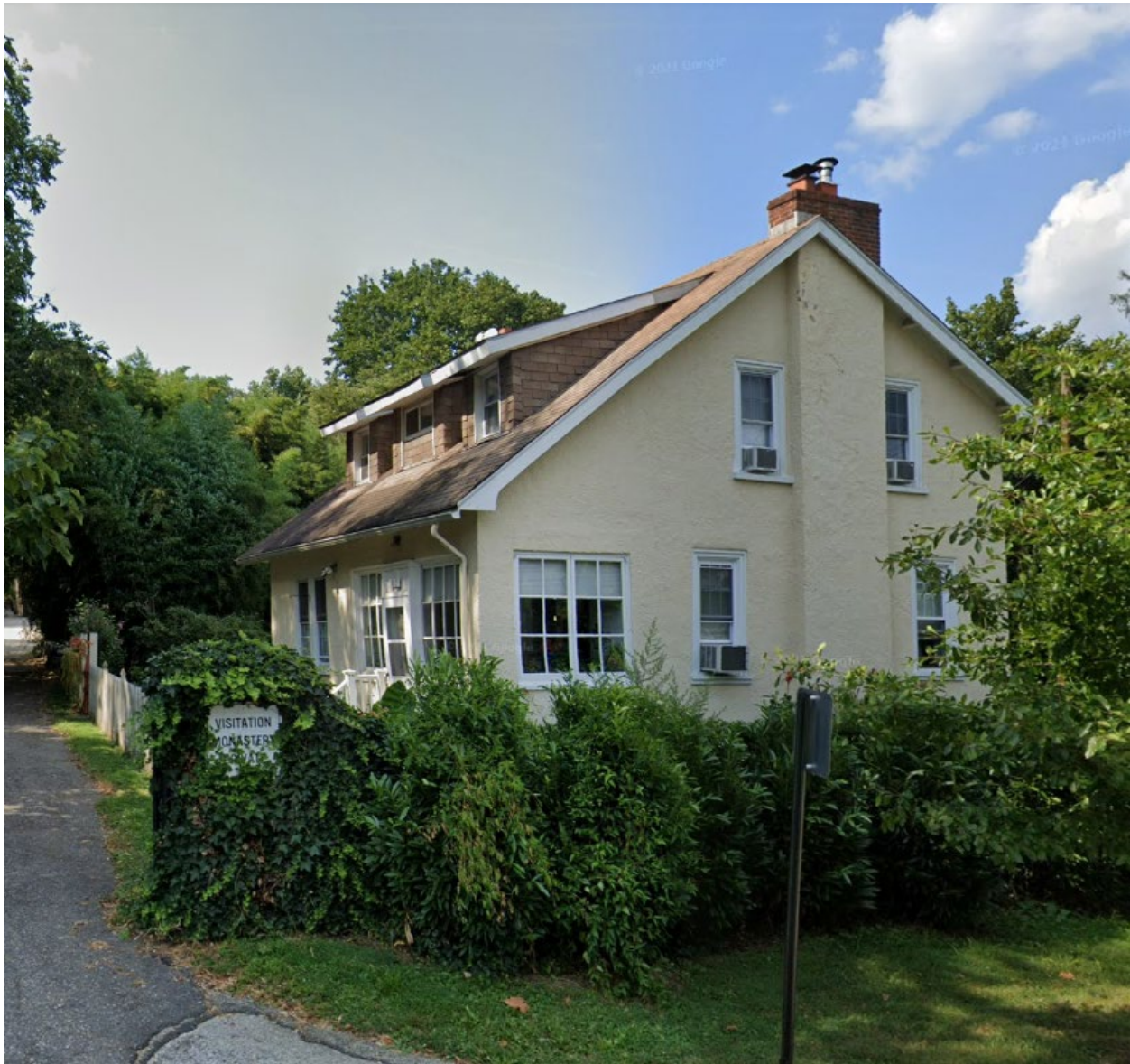
Figure 24: August 2021 image, showing the cottage at the south end of the subject property. View looking north from Overbrook Ave.
