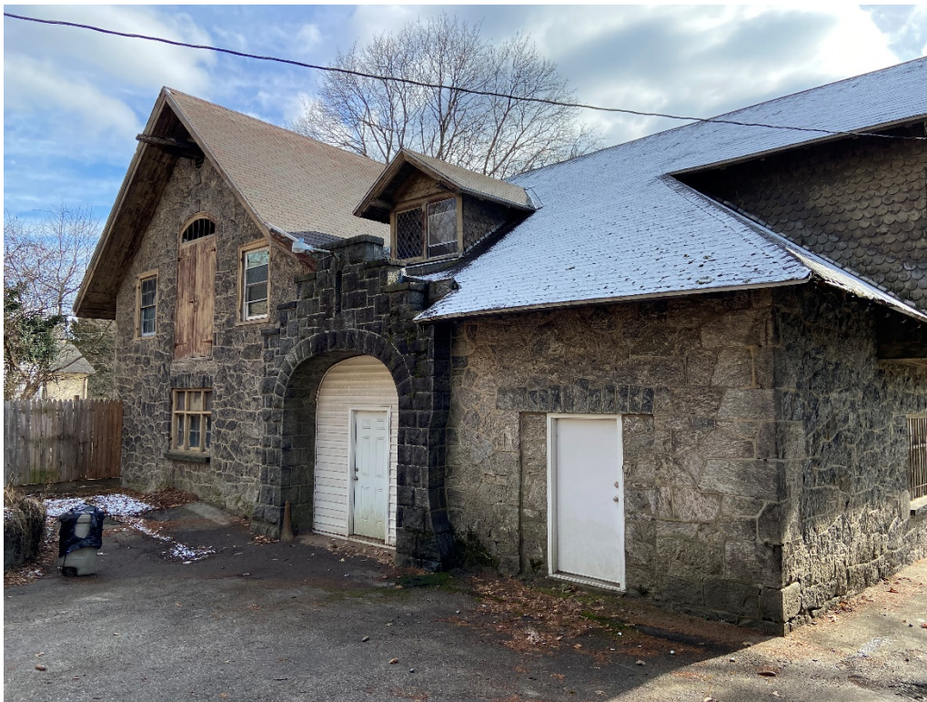
Site visit photograph, front of carriage house.
