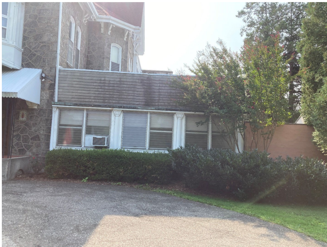
Figure 11: September 2022 photograph showing the porch addition of the mansion house. The nomination dates this building segment to c. 1900-1910. Later alterations to the porch, however, have significantly diminished its ability to convey its date/period of construction and today reads as a mid-century addition. The historic porch, which was a character-defining feature of the 19 th century country estate, no longer exists. View looking west.
