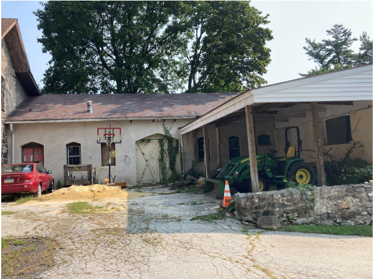
Figure 18: September 2022 photograph showing the existing conditions of the stable. View looking east.
