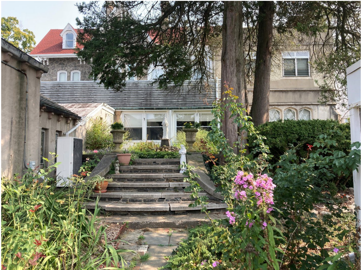
Figure 31: September 2022 photograph showing the existing condition of what was historically the main house’s porch.
