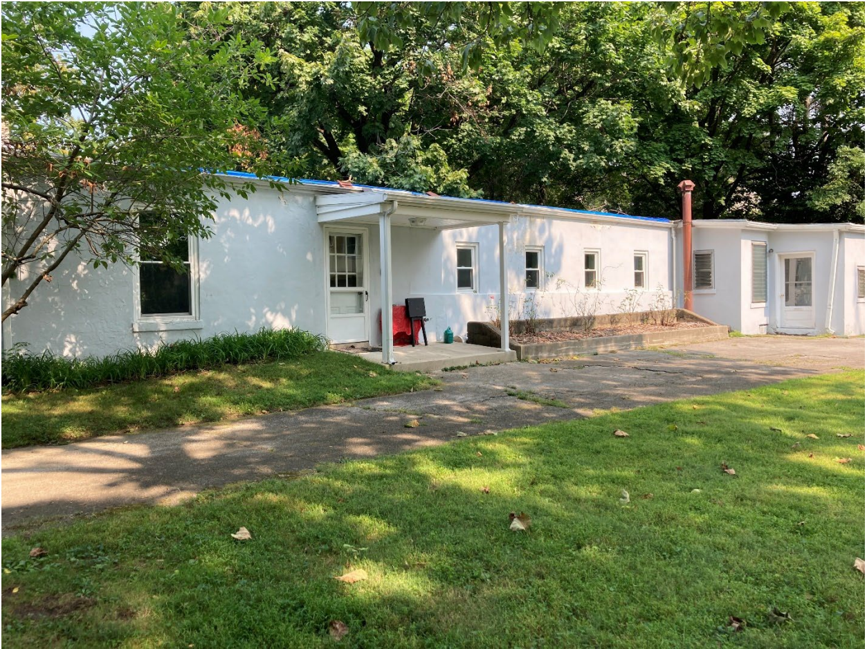
Figure 42: September 2022 photograph showing the modern CMU Block Garden Building B.
