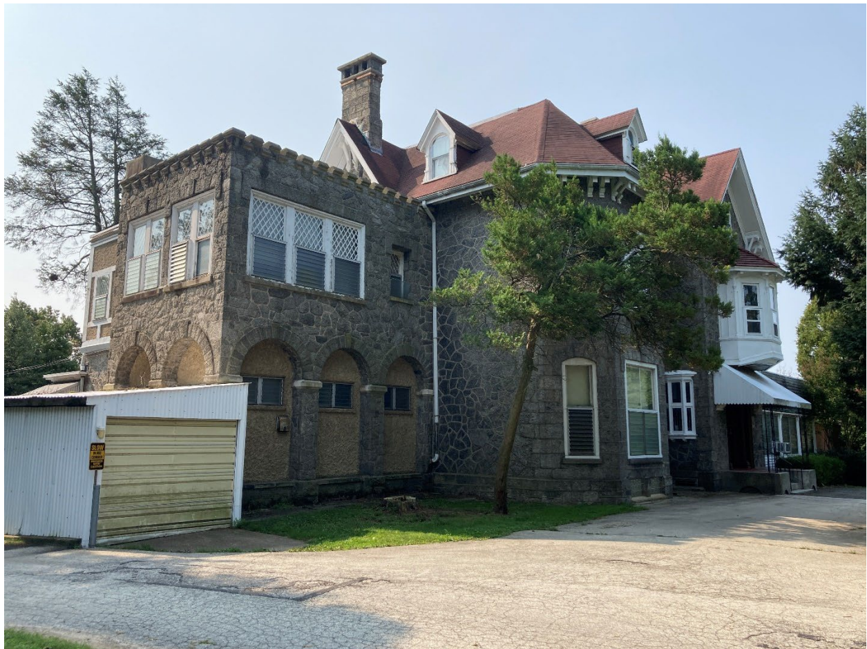
Figure 10: September 2022 photograph showing the arcade addition of the mansion house, located to the south of the main block. View looking south.
