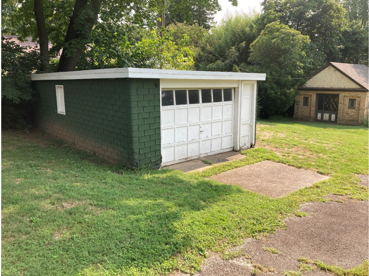
Figure 22: September 2022 photograph showing the ancillary building. View looking east.
