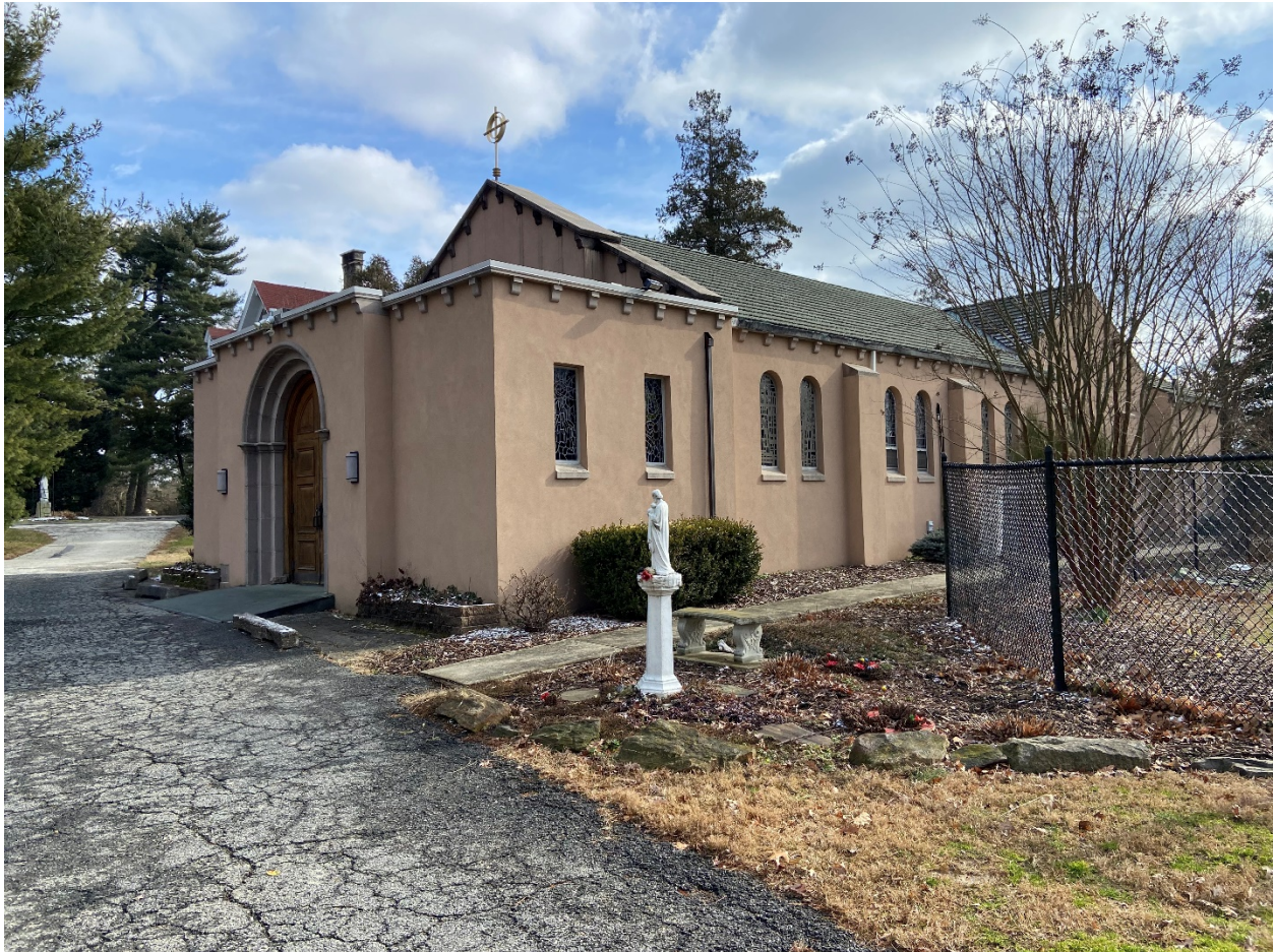
Site visit photograph, Chapel looking from the parking lot to the southeast
