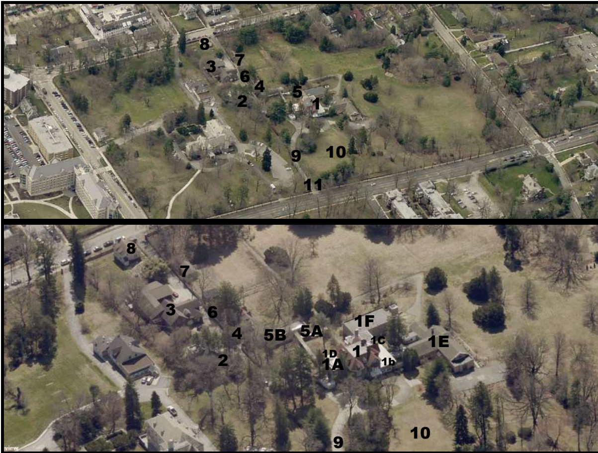
Figure 42. Top: Looking southeast at the subject property in context. Figure 43. Bottom: Looking southeast at the more specific context. Source: Pictometry, Atlas, City of Philadelphia, 2019.
