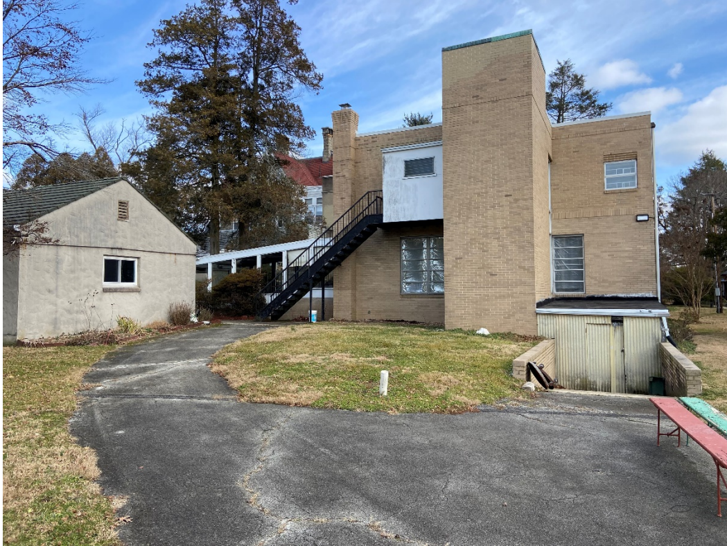
Site visit photograph, rears of the Chapel and Dormitory looking to the east
