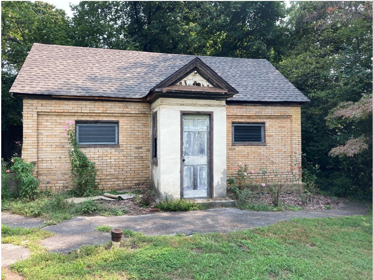
Figure 23: September 2022 photograph showing the garage/storage building. View looking east.
