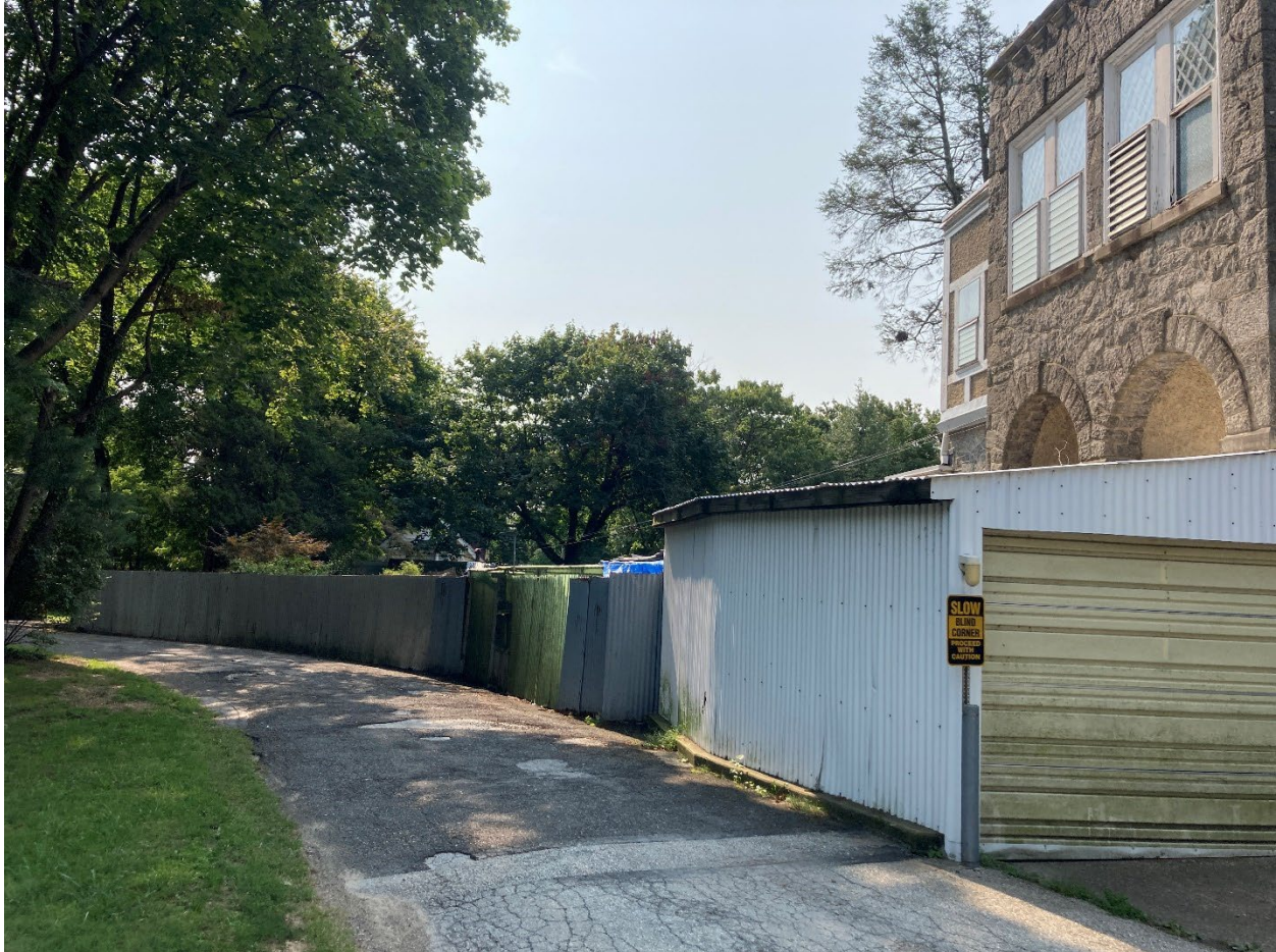
Figure 7: September 2022 photograph showing the current driveway configuration at the east end of the main house. No circular drives remain at this section of the Property.
