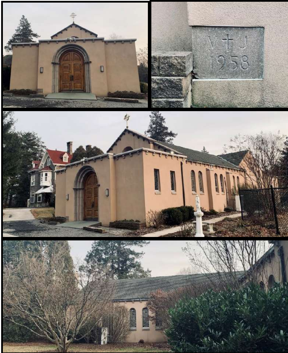
Figure 58. Left: The primary (northwest) elevation of 1e. Chapel Addition. Figure 59. Right: The “1958” cornerstone within primary (northwest) elevation of the 1e. Chapel Addition. Source: Oscar Beisert, 2019. Figure 60. Middle: The primary (northwest) and side (southwest) elevations of the 1e. Figure 61. Bottom: A side component of the primary (northwest) elevation of the 1e. Source: Oscar Beisert, 2019.
