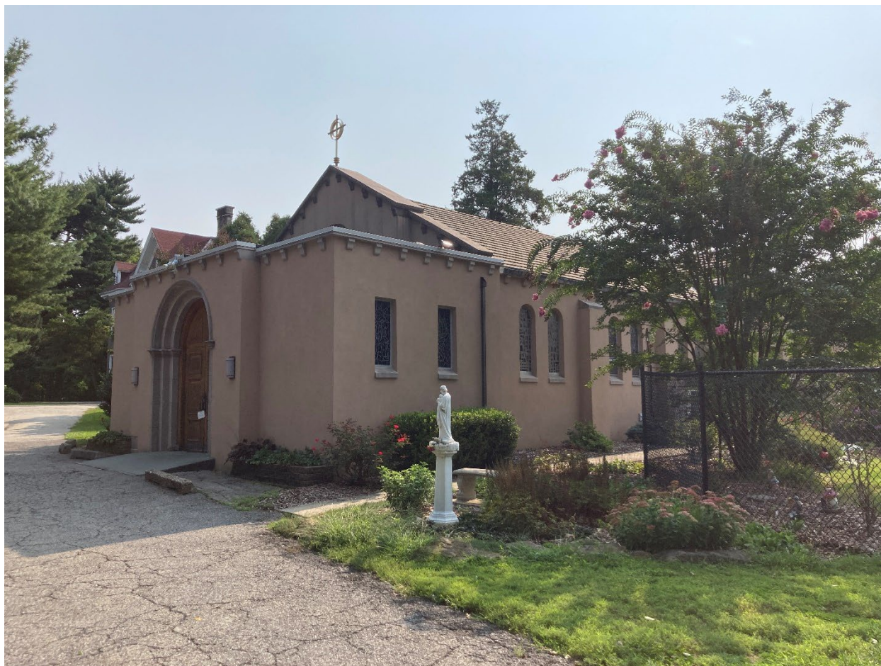
Figure 14: September 2022 photograph showing the chapel addition to the mansion house. The chapel addition is a visual intrusion when compared with the remainder of the main house. The addition eliminated the historic bucolic viewshed from the main house. View looking southeast.
