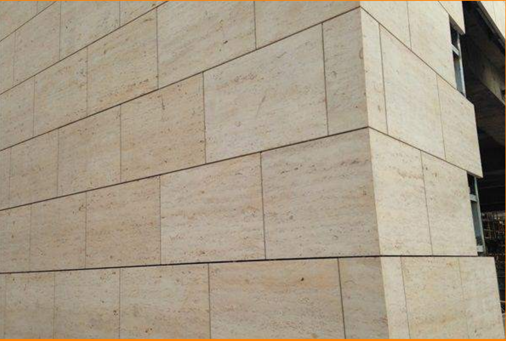
STONE PANELS ON ECO-CLAD FRAMING SYSTEM
