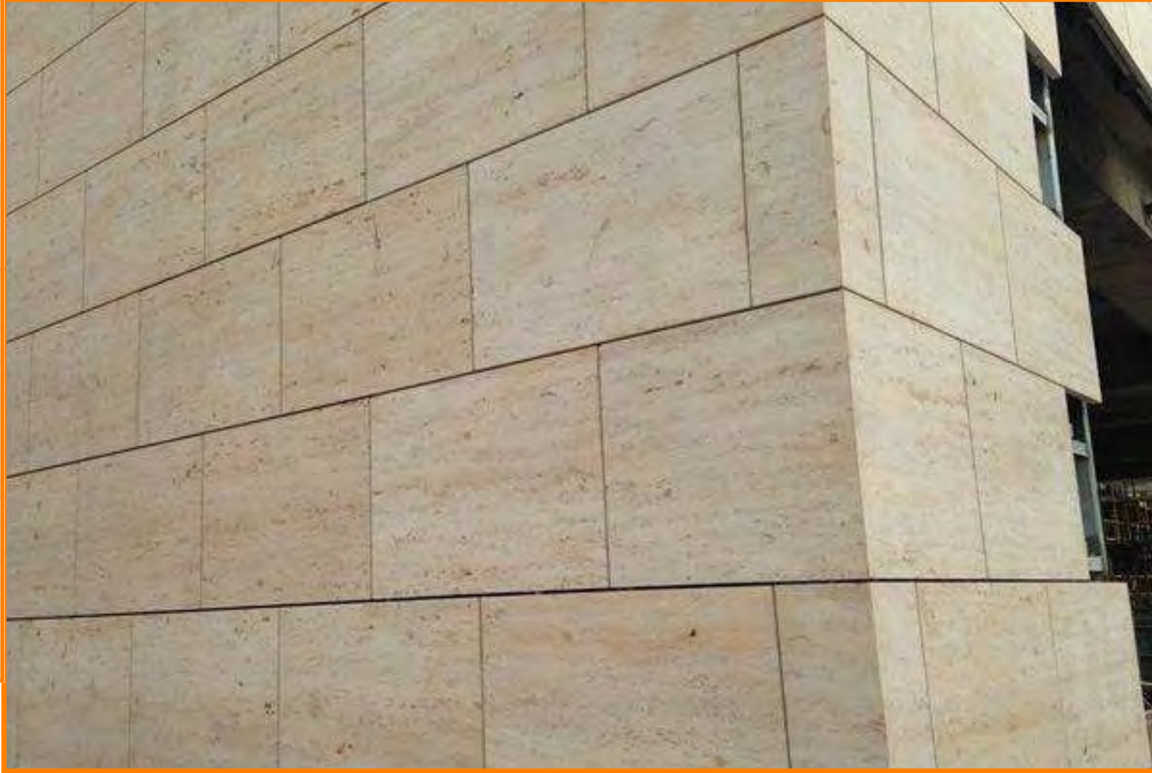
STONE PANELS ON ECO-CLAD FRAMING SYSTEM
