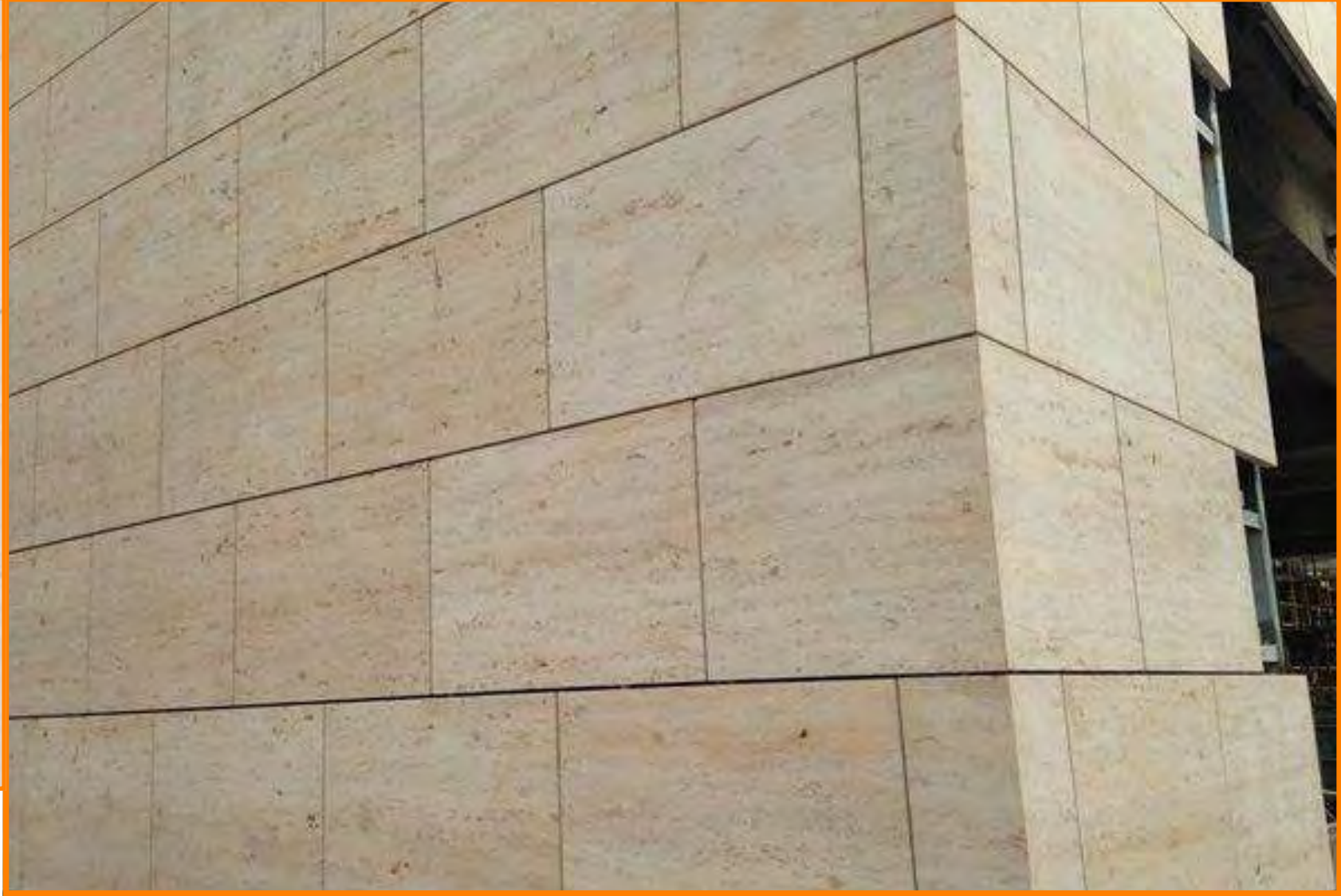
STONE PANELS ON ECO-CLAD FRAMING SYSTEM
