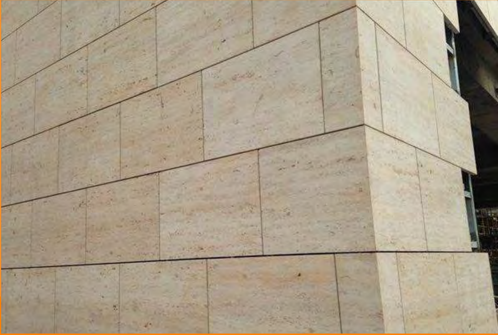
STONE PANELS ON ECO-CLAD FRAMING SYSTEM
