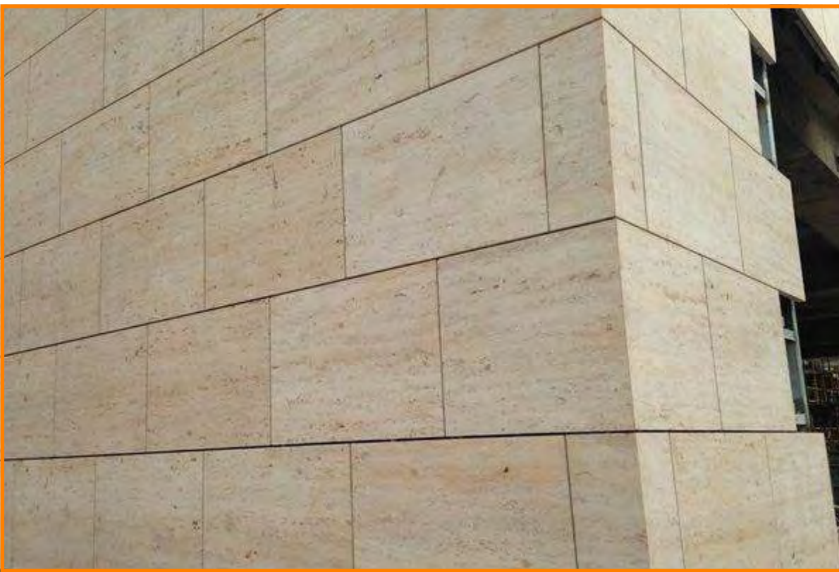
STONE PANELS ON ECO-CLAD FRAMING SYSTEM
