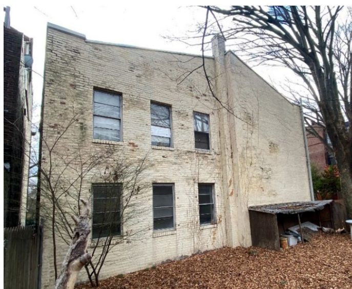
Figure 12: North elevation of the residence, looking southwest from Lawrence Court Walk. The jog in this wall matches the plan of the building as seen in the 1916 and 1950 Sanborn maps ( Figures 17 and 18 ), indicating that this portion of the building pre-dates the Church.
