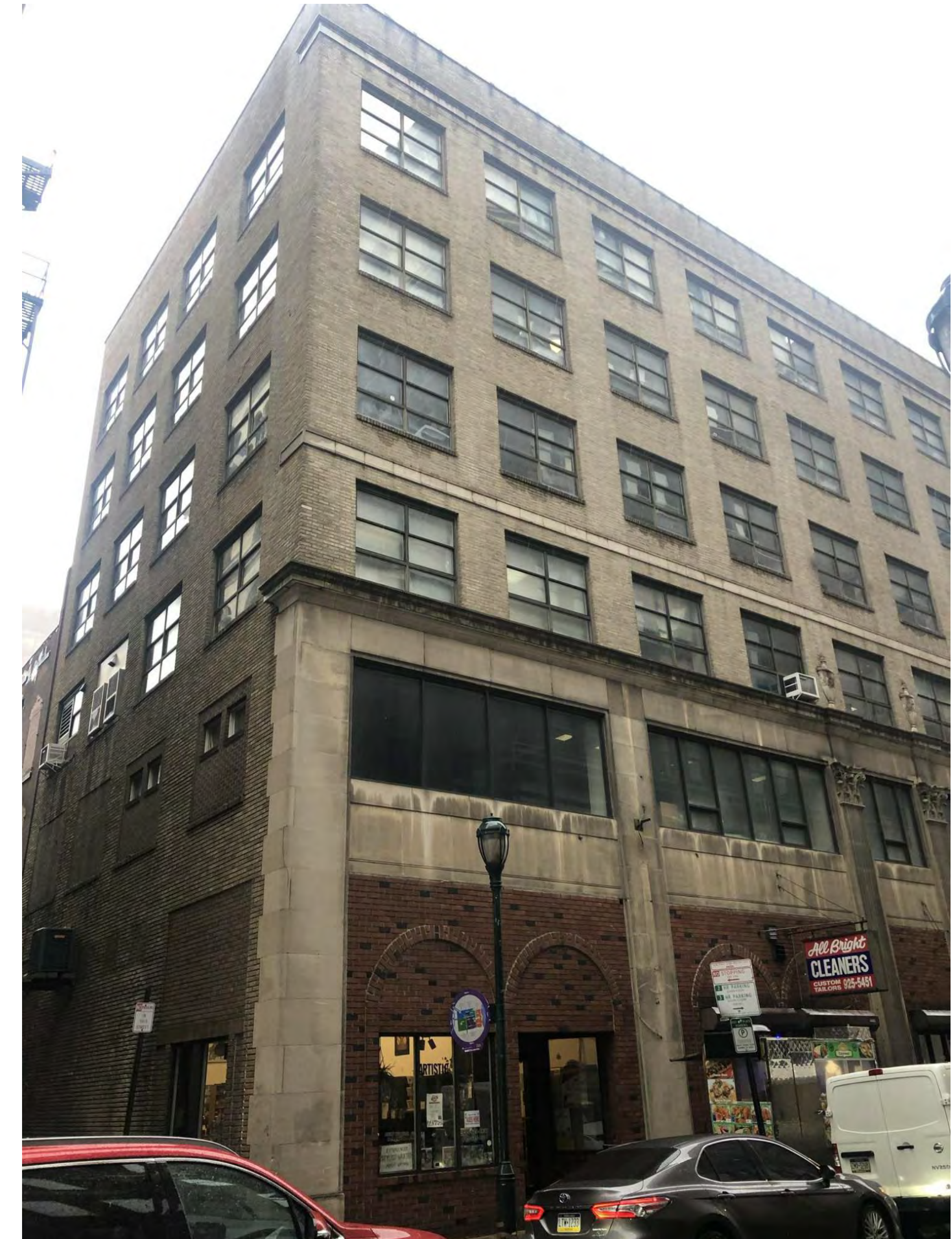
3 VIEW OF 700 CHESTNUT AT IONIC STREET
