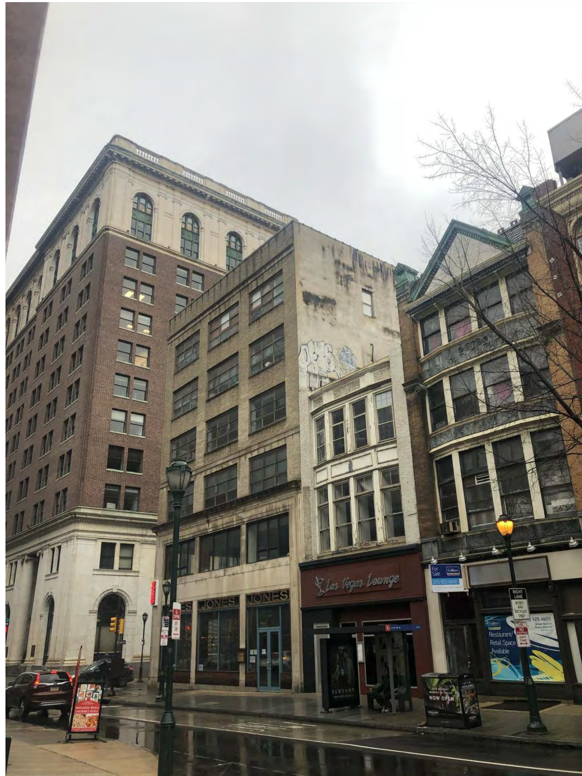
1 VIEW OF 700 CHESTNUT LOOKING SOUTH
