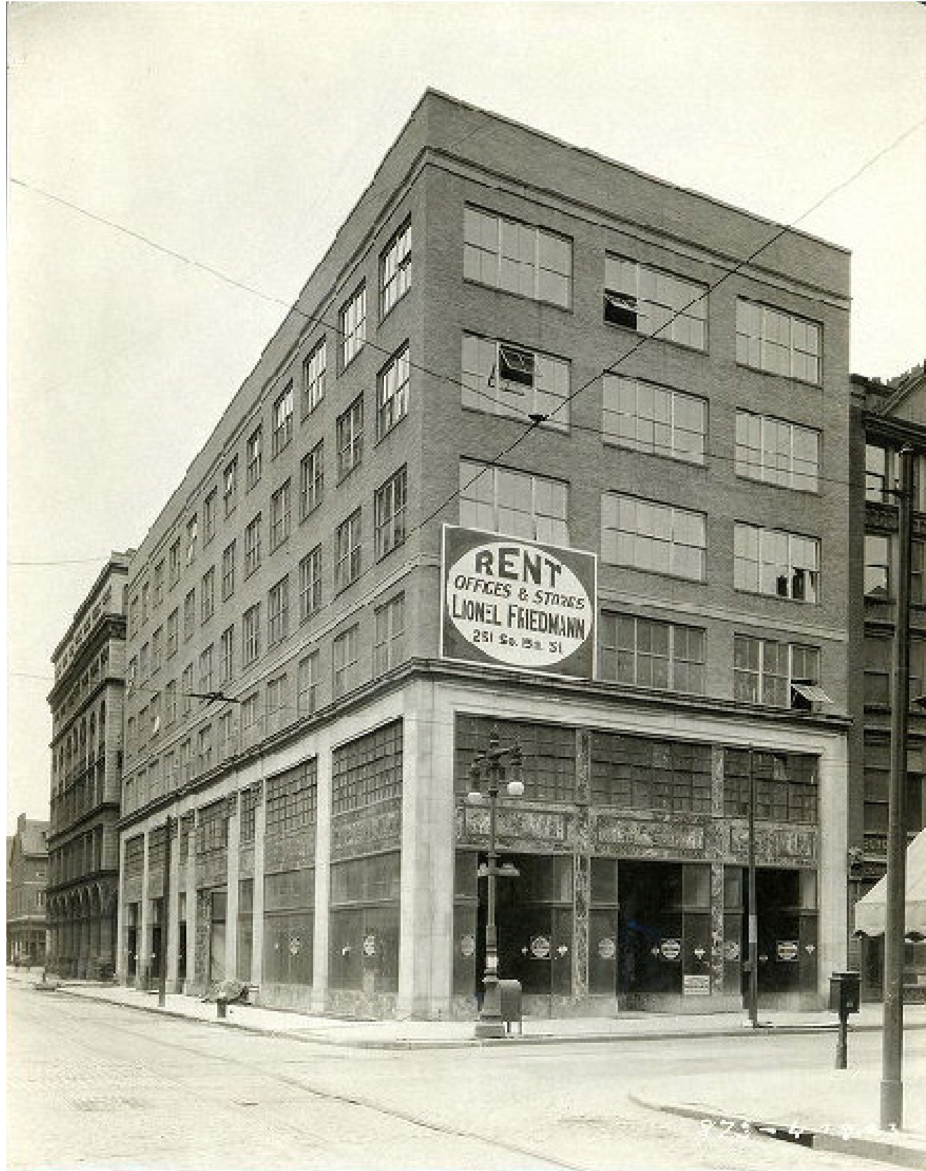
CA 1923, WASHINGTON SQUARE BUILDING
