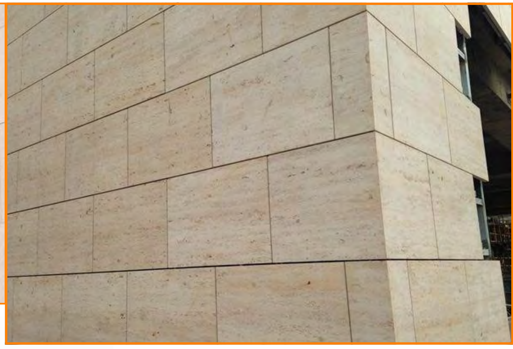
STONE PANELS ON ECO-CLAD FRAMING SYSTEM
