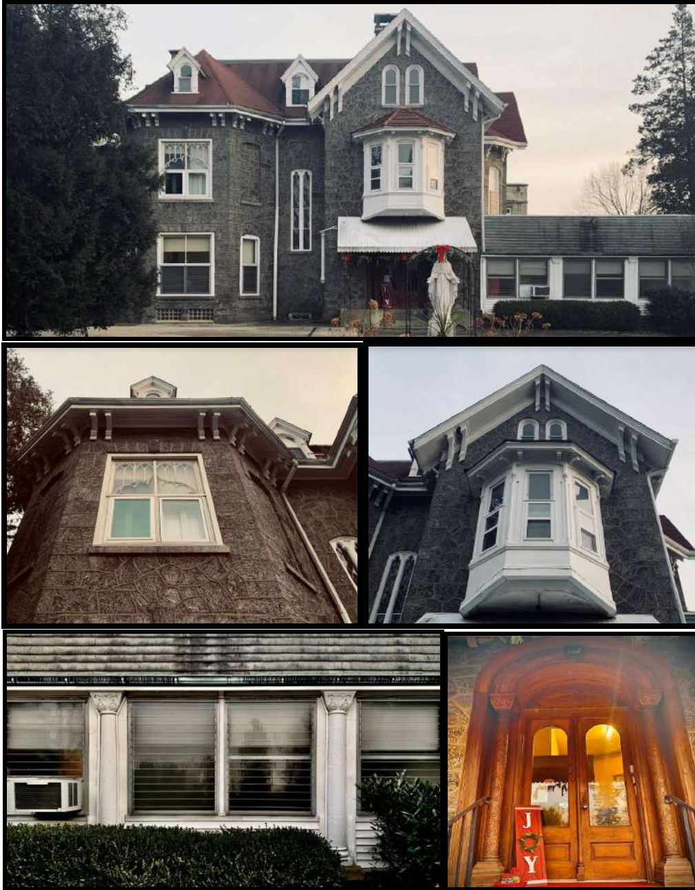
Figure 47. Top: The primary (northwest) elevation of the Main Block. Figure 48. Middle left and Figure 49. right: Details of the primary (northwest) elevation of the Main Block. Source: Oscar Beisert, 2019. Figure 50. Bottom left: The primary (northwest) elevation of the Porch Addition to the Main Block, showing the columns and cushion capitals with Norman architectural details of the porch addition. Figure 51. Bottom right: The primary entrance within the primary (northwest) elevation of the Main Block, showing similar columns and cushion capitals with Norman architectural details to the porch. Source: Oscar Beisert, 2019.
