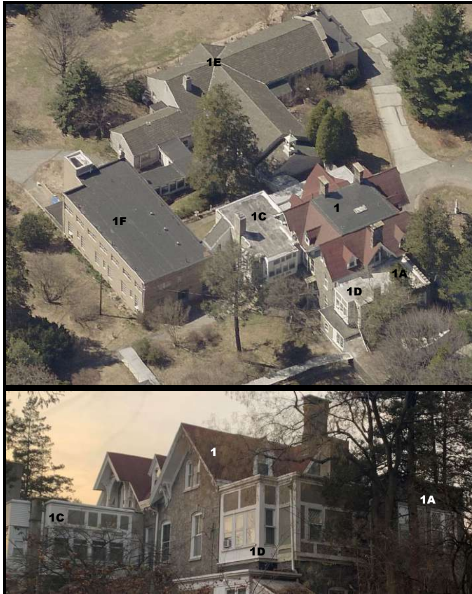
Figure 54. Top: Looking northwest at the Main Block and 1a. Arcade Addition, 1b. Porch Addition, 1c. East Addition, 1d. South Addition, 1e. Chapel Addition, and 1f. Dormitory. Source: Pictometry, Atlas, City of Philadelphia, 2019. Figure 55. Bottom: The rear (southeast) and side (northeast) elevations of the Main Block with 1c. East Addition, 1d. South Addition, and 1a. Arcade Addition also in view. Source: Oscar Beisert, 2019.
