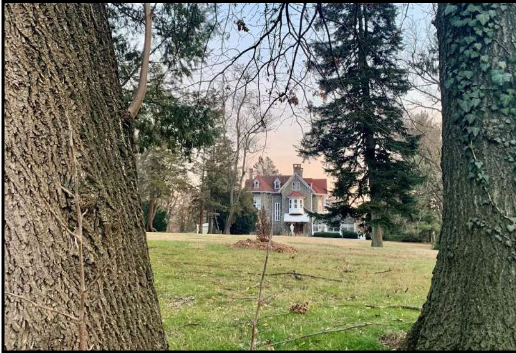
Figure 1. Looking southeast at the primary (northwest) elevation of the Main Block of the Mansion House. Source: Oscar Beisert, 2019.
