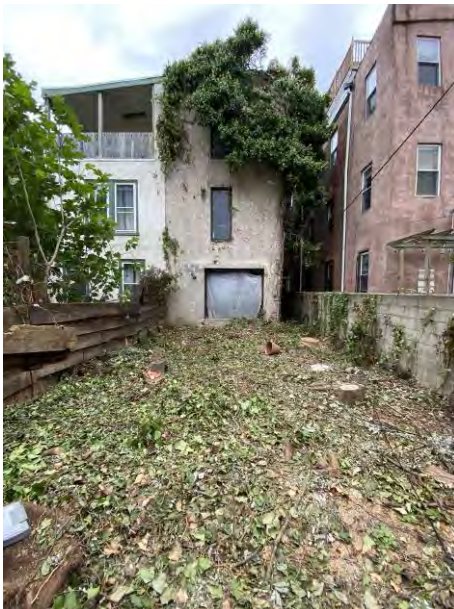
Photo 3: Existing Rear Yard (Future Addition above existing rear portion (walls to remain, rear roof to be demolished). New extension from rear wall to limits in plan.
