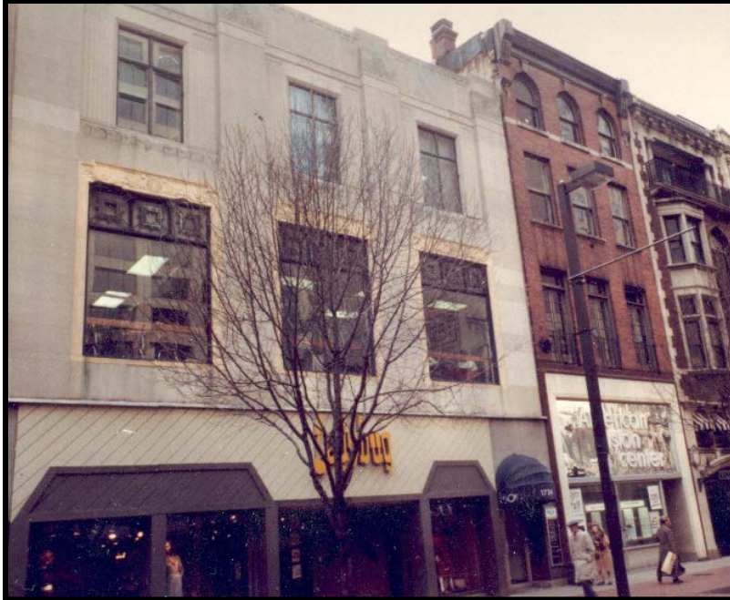
Figure 6. The primary (north) elevation in 1983. Source: Jefferson Moak, Philadelphia Historical Commission.
