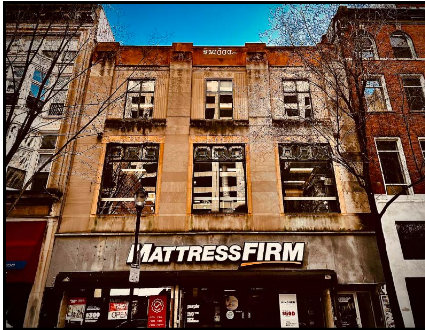
Figure 1. The primary (north) elevation of the subject property. Source: Oscar Beisert, 2022.
