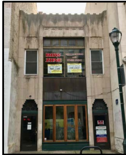
Figure 21. The Durham & Co. Radio Showroom, Philadelphia W3XM Radio Station, 2006 Chestnut Street. Source: Oscar Beisert. Philadelphia Register of Historic Places Nomination: The Durham & Co. Radio Showroom, Philadelphia W3XM Radio Station, 2006 Chestnut Street (1928) . (Philadelphia: The Keeping Society, 2020).
