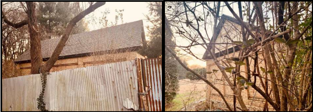
Figure 81. Left: The northeast elevation of the Garage/Storage Building. Source: Oscar Beisert, 2019. Figure 82. Right: The southeast elevation of the Garage/Storage Building. Source: Oscar Beisert, 2019.
