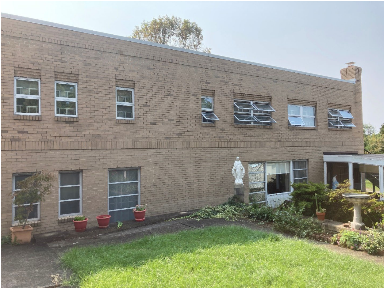
Figure 15: September 2022 photograph showing the dormitory addition to the mansion house. The dormitory addition is a visual intrusion when compared with the remainder of the main house. The addition eliminated the historic bucolic viewshed from the main house. View looking south.
