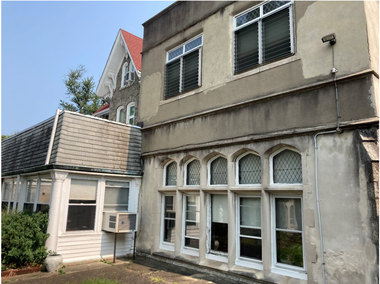
Figure 12: September 2022 photograph showing the east addition, which is situated at center of the mansion house. View looking east.
