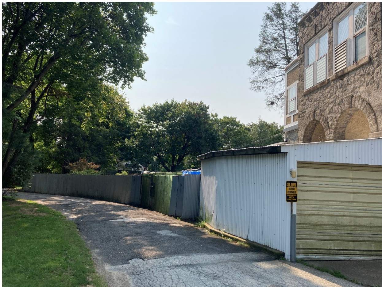
Figure 7: September 2022 photograph showing the current driveway configuration at the east end of the main house. No circular drives remain at this section of the Property.
