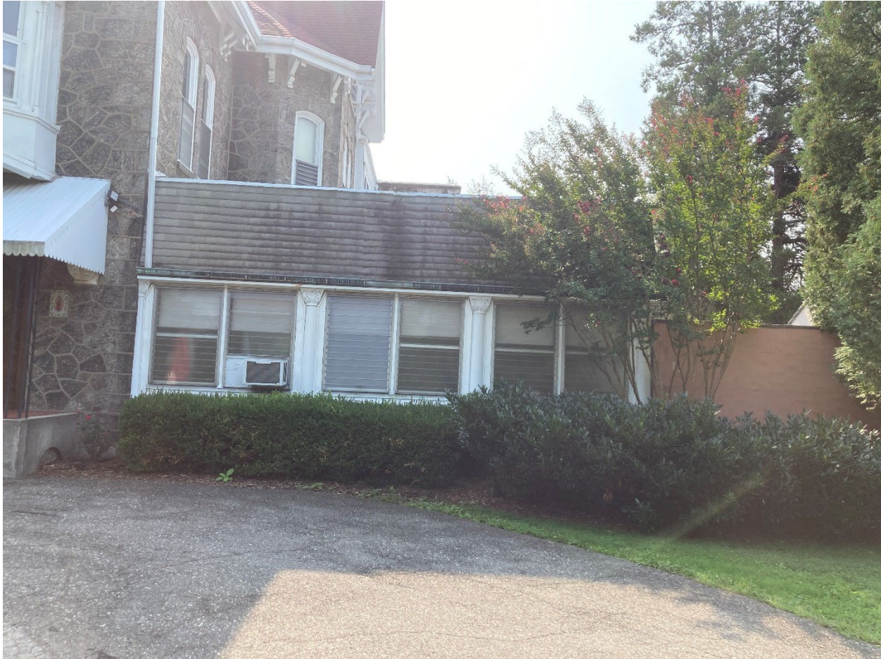
Figure 11: September 2022 photograph showing the porch addition of the mansion house. The nomination dates this building segment to c. 1900-1910. Later alterations to the porch, however, have significantly diminished its ability to convey its date/period of construction and today reads as a mid-century addition. The historic porch, which was a character-defining feature of the 19 th century country estate, no longer exists. View looking west.
