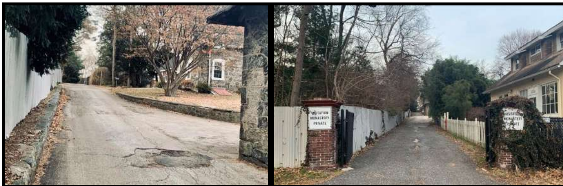
Figure 15. Left: Looking northwest from the rear of the subject property at the Rear Driveway with the Carriage House & Stable and Gardener's Cottage on right. Figure 16. Right: Looking northwest from the rear of the subject property at the Driveway, showing the brick posts on each side and the Gardener's Cottage on right. Source: Oscar Beisert, 2019.
