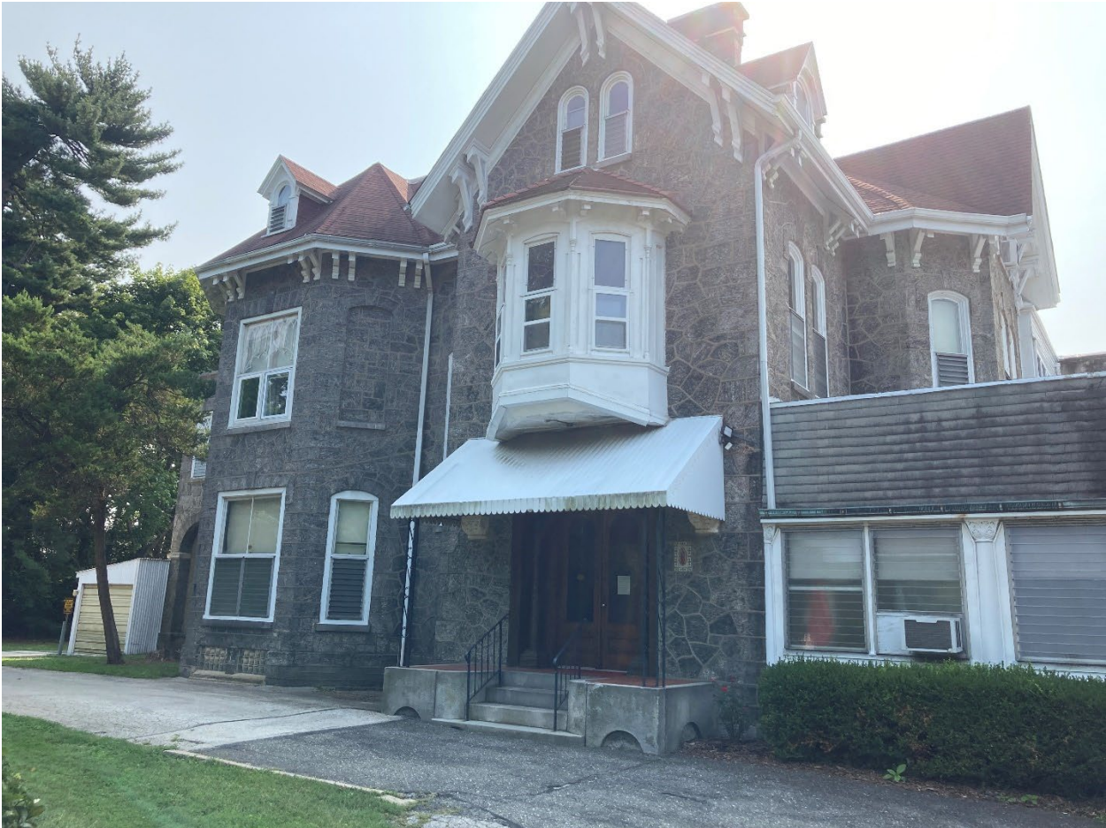
Figure 9: September 2022 photograph showing the main block of the mansion house, which is the oldest portion of the building. View looking southeast.
