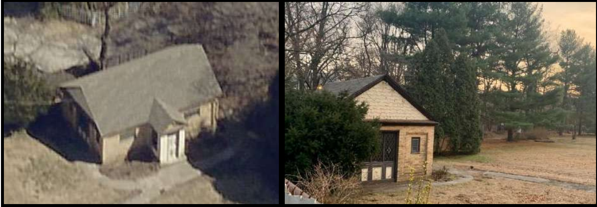
Figure 79. Left: The southwest elevation of the Garage/Storage Building. Source: Pictometry, Atlas, City of Philadelphia, 2019. Figure 80. Right: The northwest elevation of the Garage/Storage Building. Source: Oscar Beisert, 2019.
