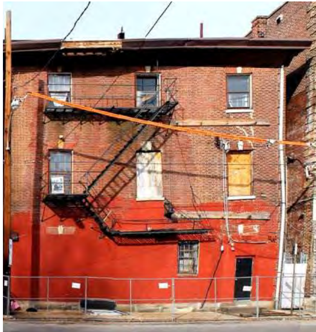
Figure 9: A 2017 photograph of the eastern side of the southeast elevation features the dramatic bend of the structure's east corner that demanded structural remedy, seen below. The foundation may date to the 1870s and is presumed to be a contributing factor to the structural instability. (Photo by Sara Stratte.)
