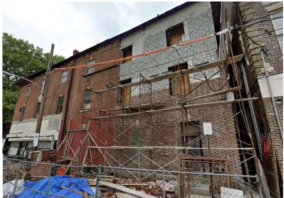
Figure 10: This photo from Google Streetview shows the stabilization and reconstruction efforts underway in 2019. The rebuilt portion uses concrete masonry units clad in brick.
