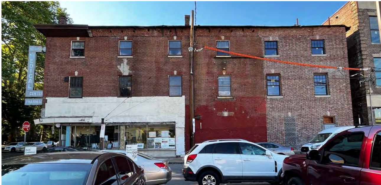
Figure 8: Price Street (Southeast) elevation of 5801-03 Germantown Ave. Photo by Nika Faulkner. Note the new matching windows, Flemish bond brick veneer that differs in color, and lack of cornice.
