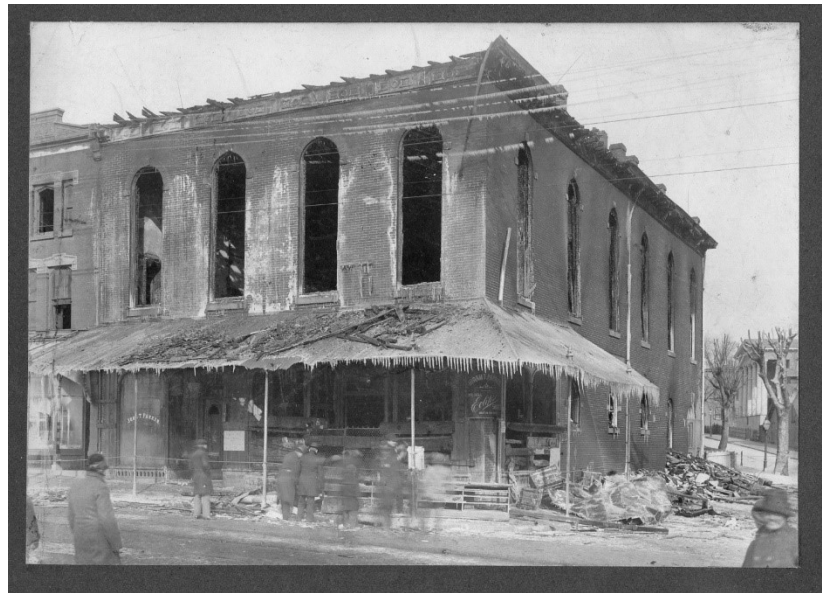
Figure 21: Parker's Hall after a fire that gutted the building, ultimately leading to its demolition and the reconstruction of a new building on the remaining foundation (the building which stands today.) "Parker Hall fire," erroneously dated 1899. Germantown Historical Society. https://germantownhistory.catalogaccess.com/photos/8815 .
