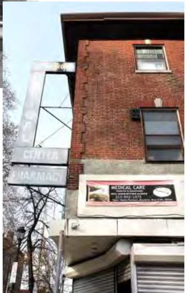
Figure 7: The southern corner of the building shows layers of modifications, including the mid-century sign and stucco covering up scars from the cornice which once ran along the first floor.
