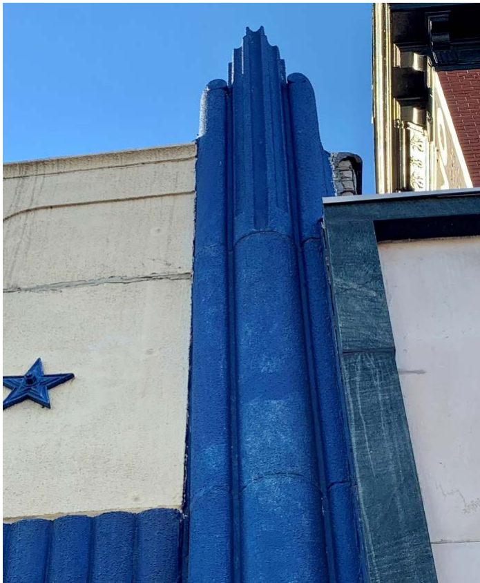
Figure 8. Close-up view of piers and texture of painted concrete "cast stone" panels, December 2022.
