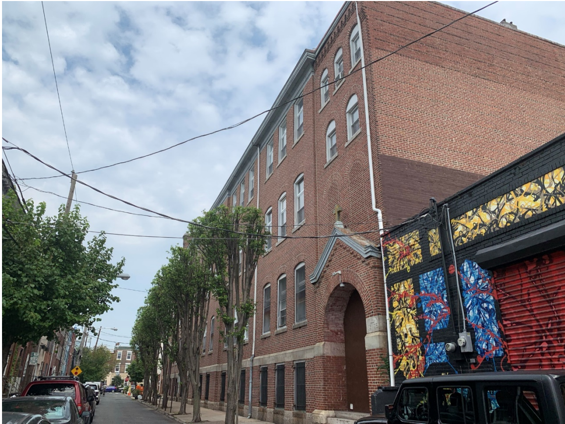
Figure 1. The Montrose Street façade of the 1905 St. Paul's Parochial School, looking west. July 2021.
