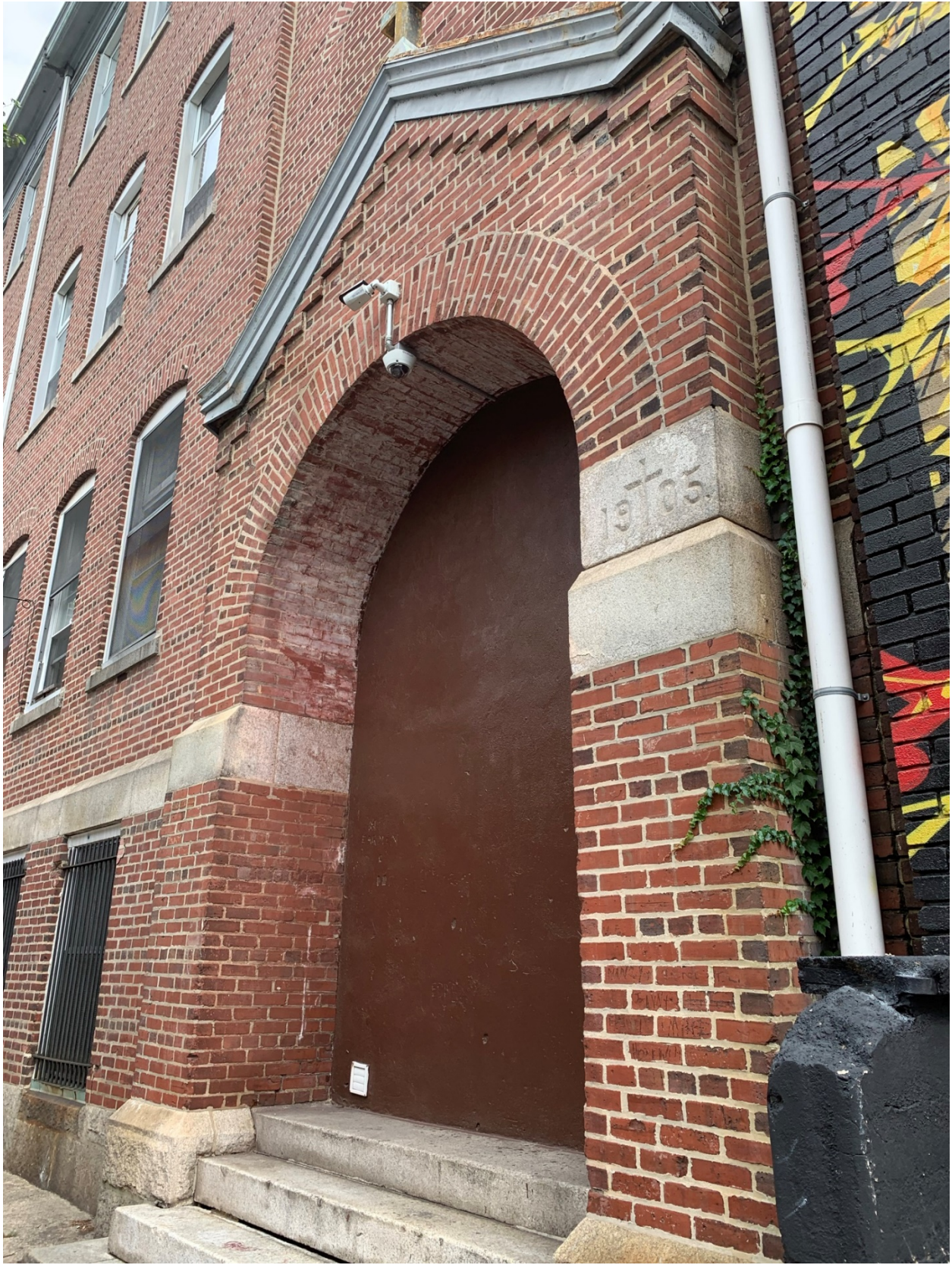
Figure 3. Eastern entrance on the Montrose Street façade with 1905 cornerstone. July 2021.
