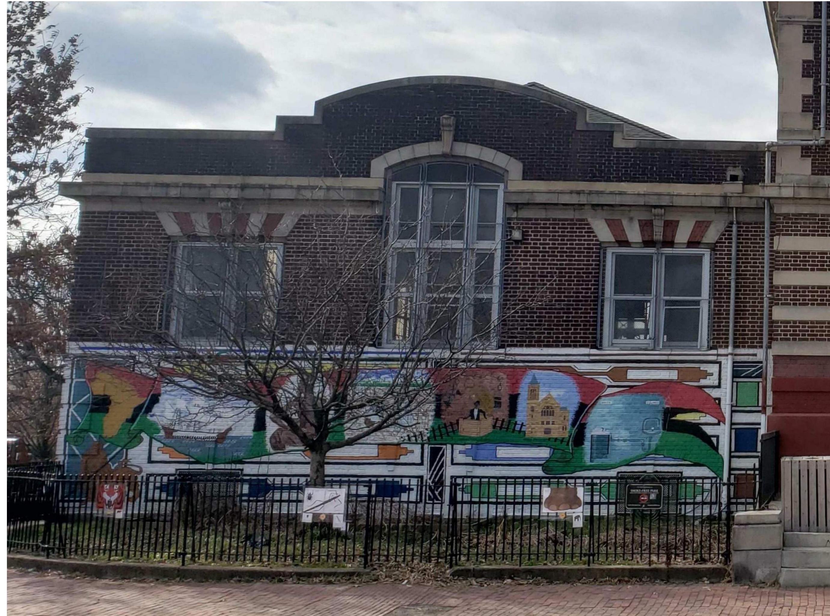
MAIN ENTRY - EAST ELEVATION (PLAZA, SOUTH)
