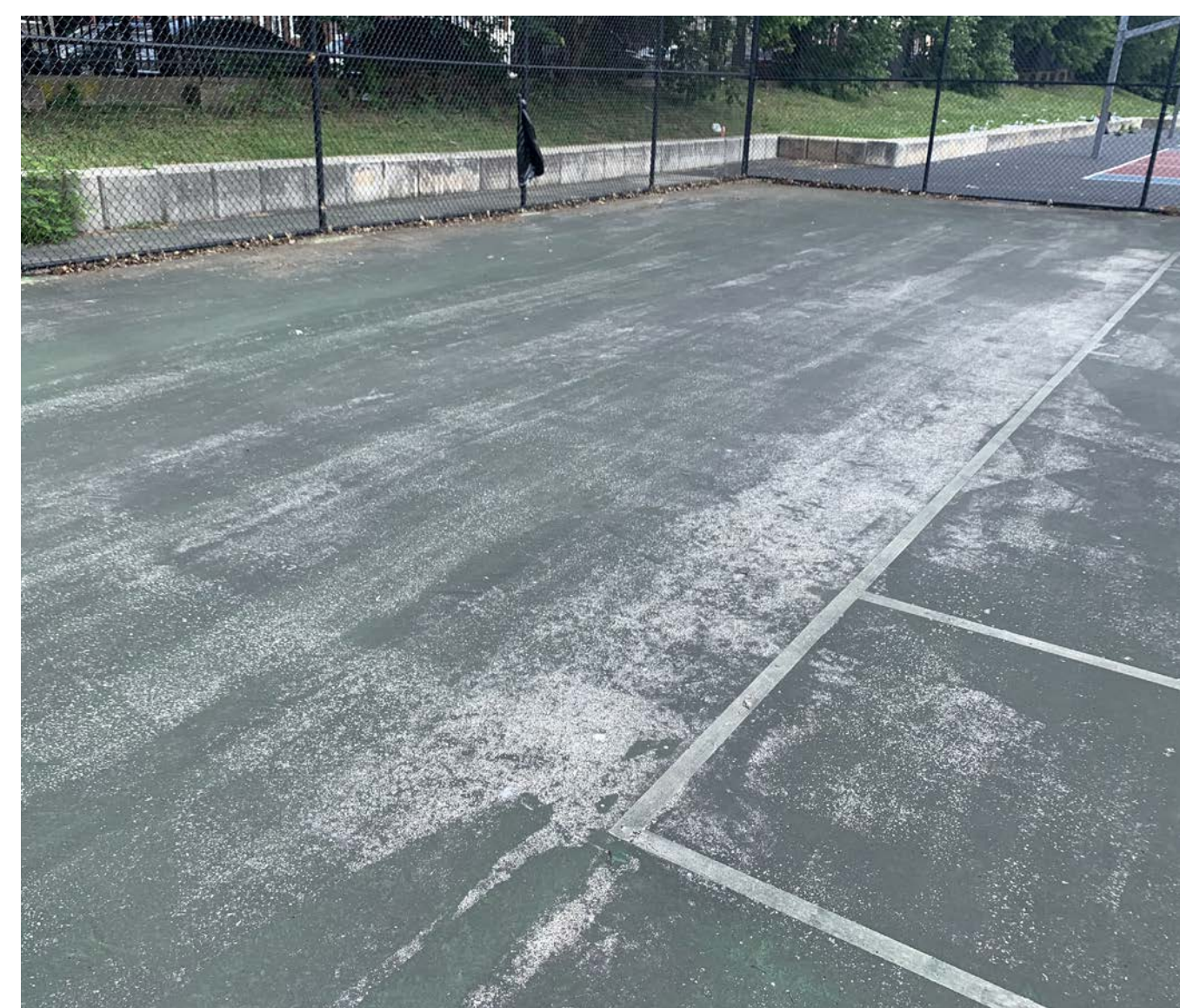
8 EXISTING TENNIS COURT SURFACING
