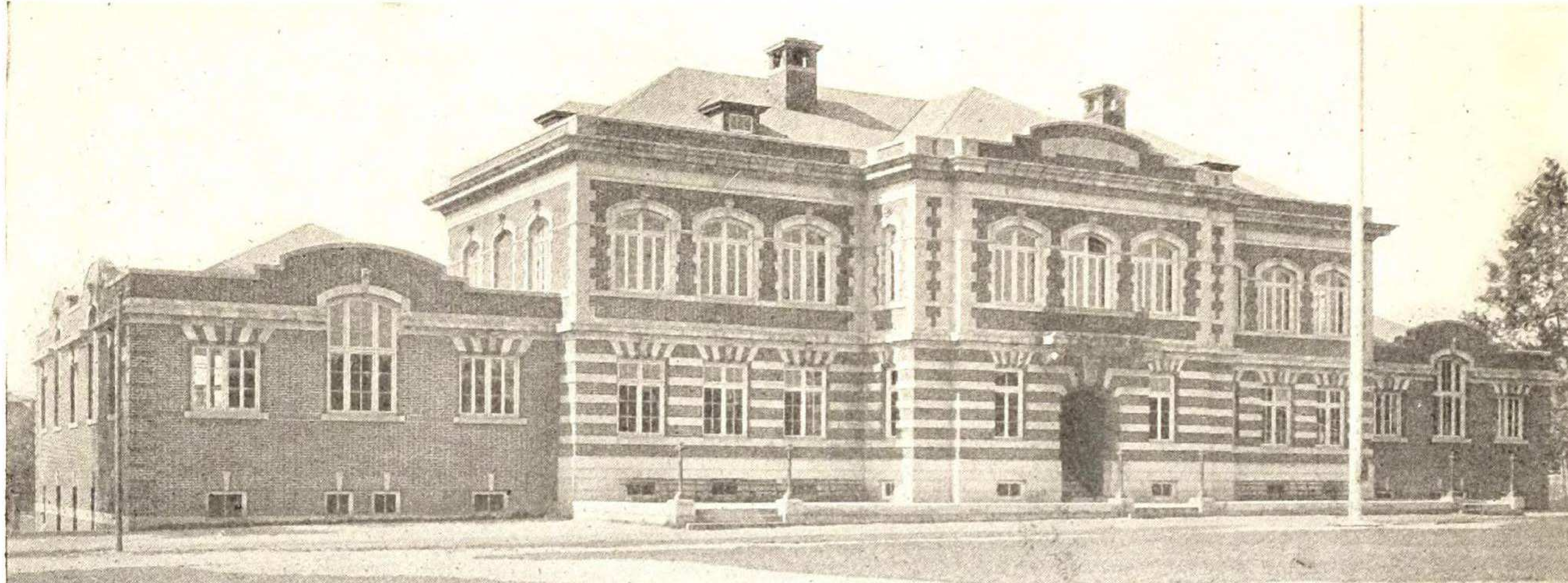
EAST ELEVATION - JULY 1923
