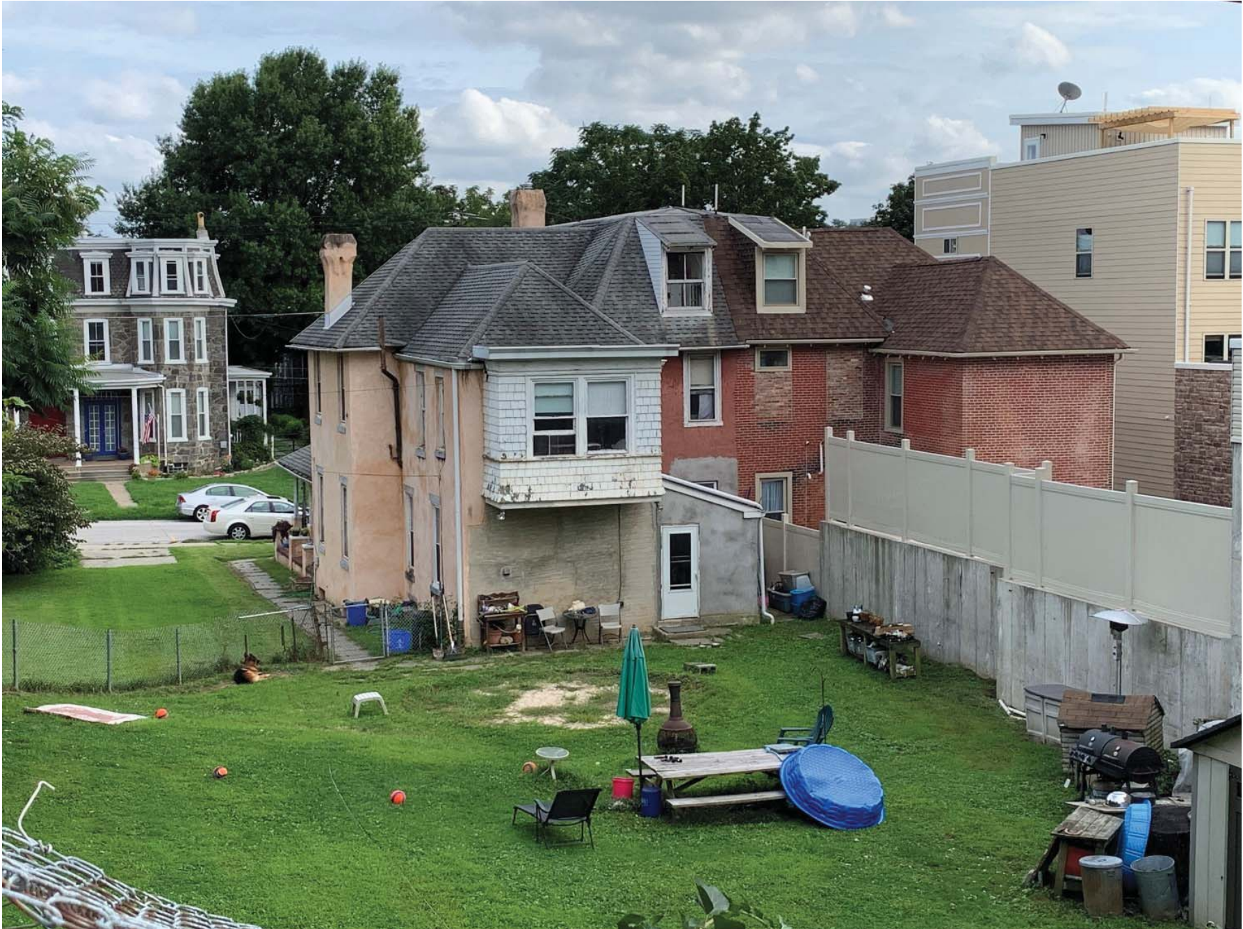
Rear of 145 Sumac Street (right) and 147 Sumac Street (left). View from Kalos Street. July 2019.
