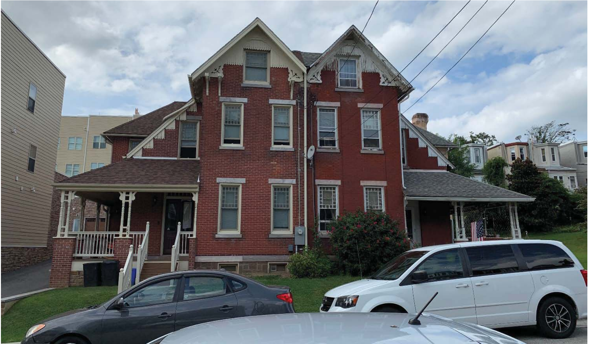
145 Sumac Street (left) and 147 Sumac Street (right). Primary facades fronting Sumac Street. July 2019.
