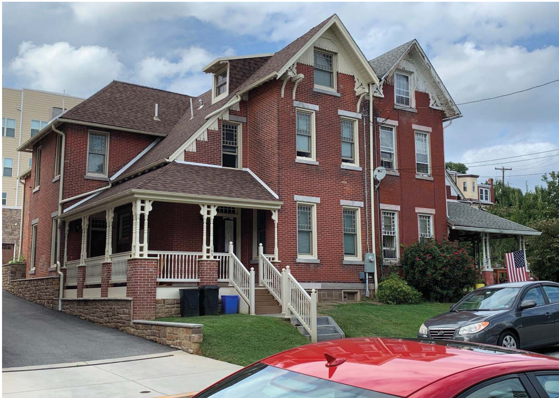
145 Sumac Street (left) and 147 Sumac Street (right). Primary facades fronting Sumac Street, and side of 145 Sumac Street. July 2019.
