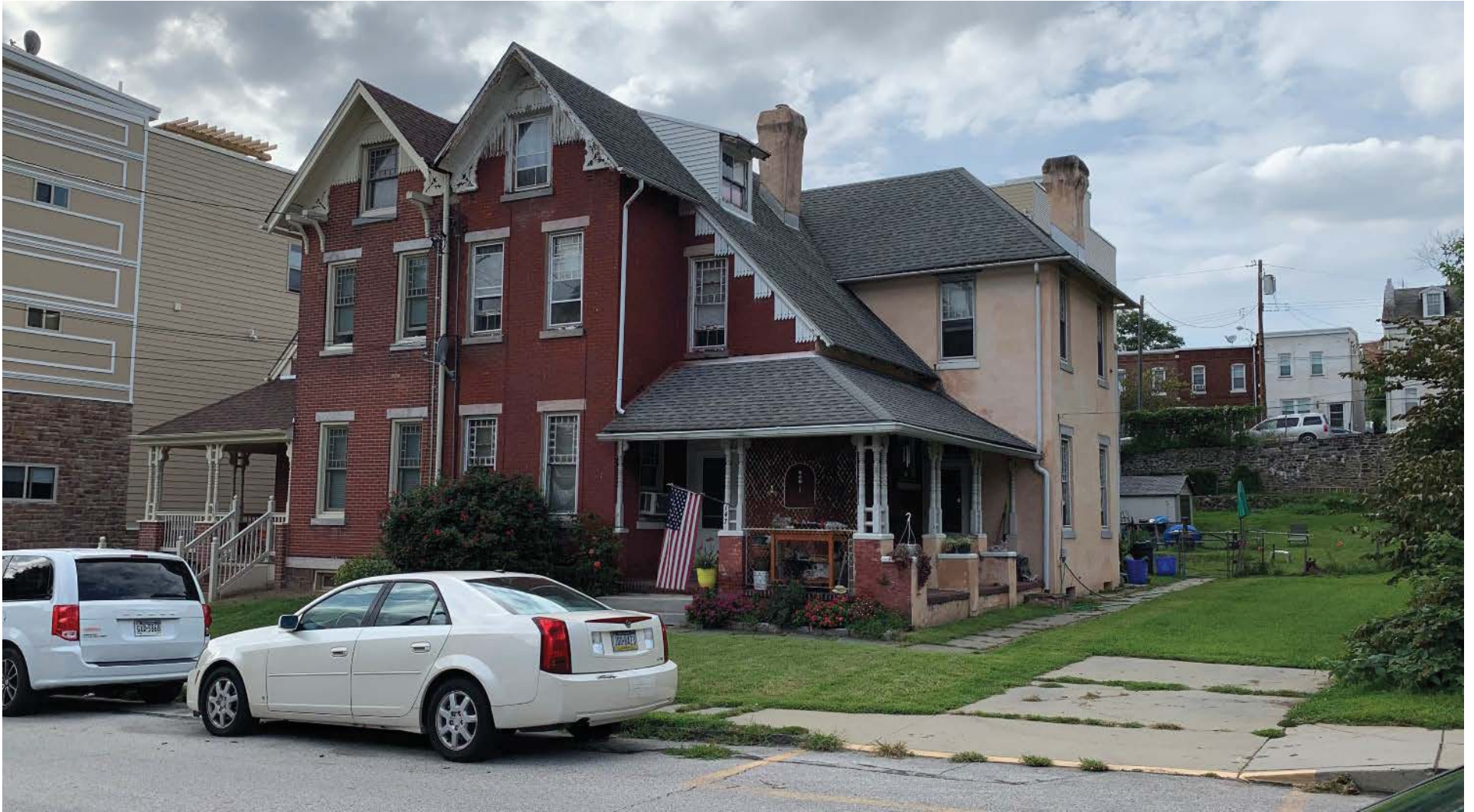
145 Sumac Street (left) and 147 Sumac Street (right). Primary facades fronting Sumac Street, and side of 147 Sumac Street. July 2019.
