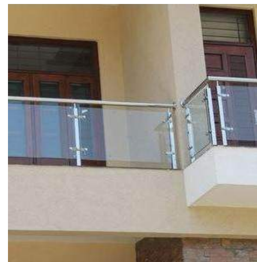
10- Aluminum and Glass Railing
