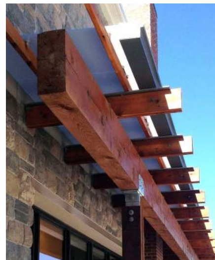
11- Exposed Cedar Roof Framing
