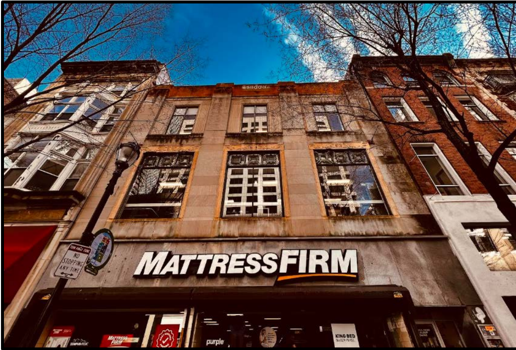
Figure 3. The primary (north) elevation of the subject property. Source: Oscar Beisert, 2022.
