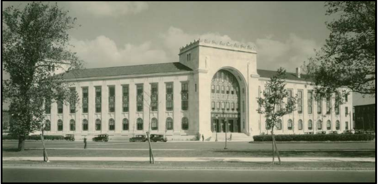
Figure 15. Fidelity Mutual Life Insurance Company Building, 1926, Zantsinger, Borie, & Medary, 26 th and Fairmont Avenue. Source: Building a Nation: Limestone Photograph Collection, Indiana University Bloomington.
