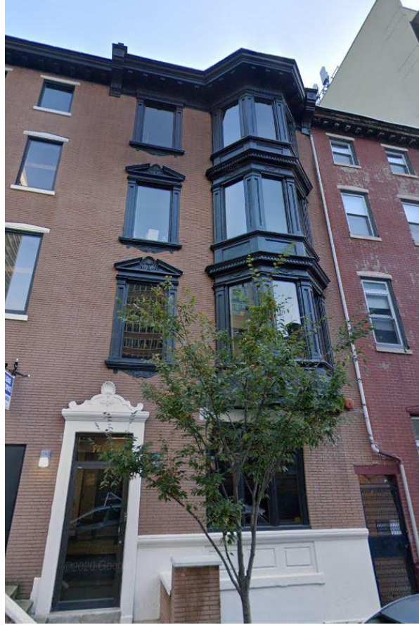
Figure 7 - 1706 Race Street, north elevation (facing Race Street).
