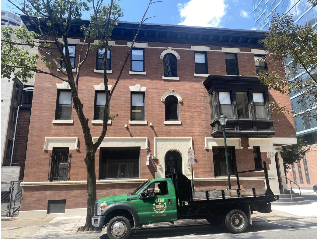
Figure 4 - 1700-02 Race Street, east elevation (facing 17th Street).
