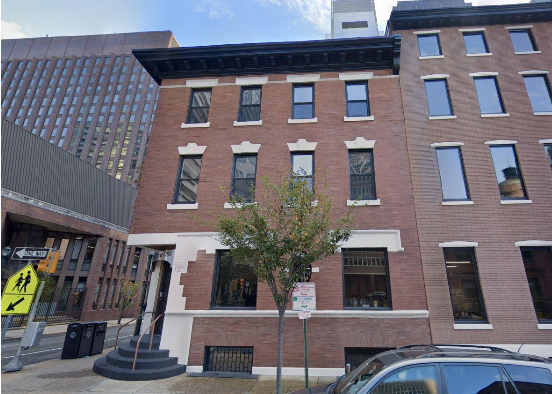
Figure 3 - 1700-02 Race Street, north elevation (facing Race Street).
