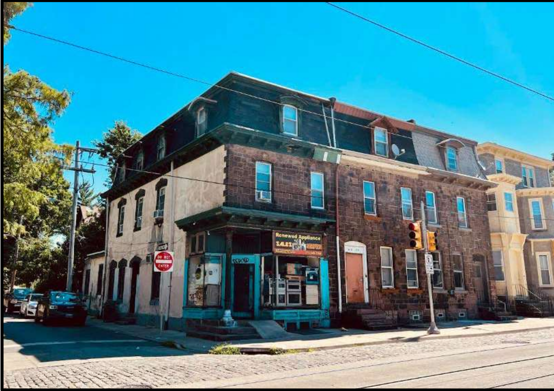
Figure 3. Top: The primary elevation (southwest) and side (northwest) elevations of 4841 Germantown Avenue. Source: Keeping Society of Philadelphia, 2022.
