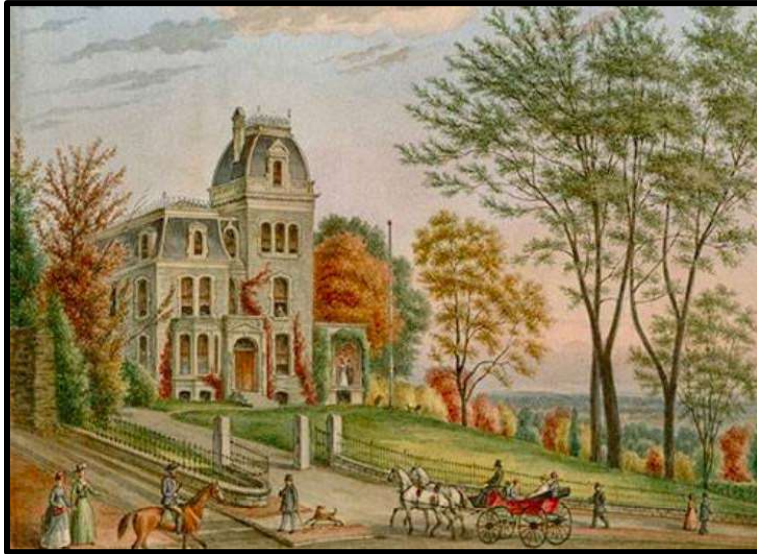
Figure 17. Bottom: The William Adamson Mansion, 4811 Germantown Avenue, Germantown, Pa., ca. 1920s. Source: The Germantown Historical Society.
