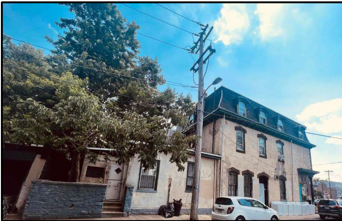
Figure 9. The side (northwest) elevation. Source: Keeping Society of Philadelphia, 2022.
