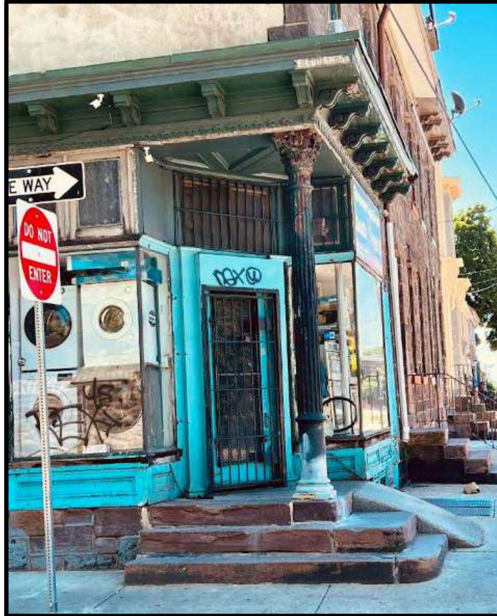
Figure 6. Top: The primary (southwest) and side (northwest) elevations at the corner of Germantown Avenue and East Logan Street. Figure 7. Bottom: The corner storefront. Source: Keeping Society of Philadelphia, 2022.
