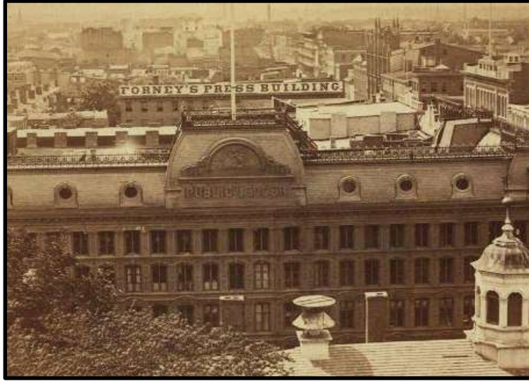
Figure 21. Public Ledger Building, Philadelphia, Pennsylvania, ca. 1867. Source: The Library Company of Philadelphia.
