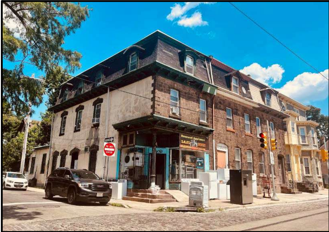
Figure 1. The side (northwest) and primary (southwest) elevations of the subject property. Source: Keeping Society of Philadelphia, 2022.
