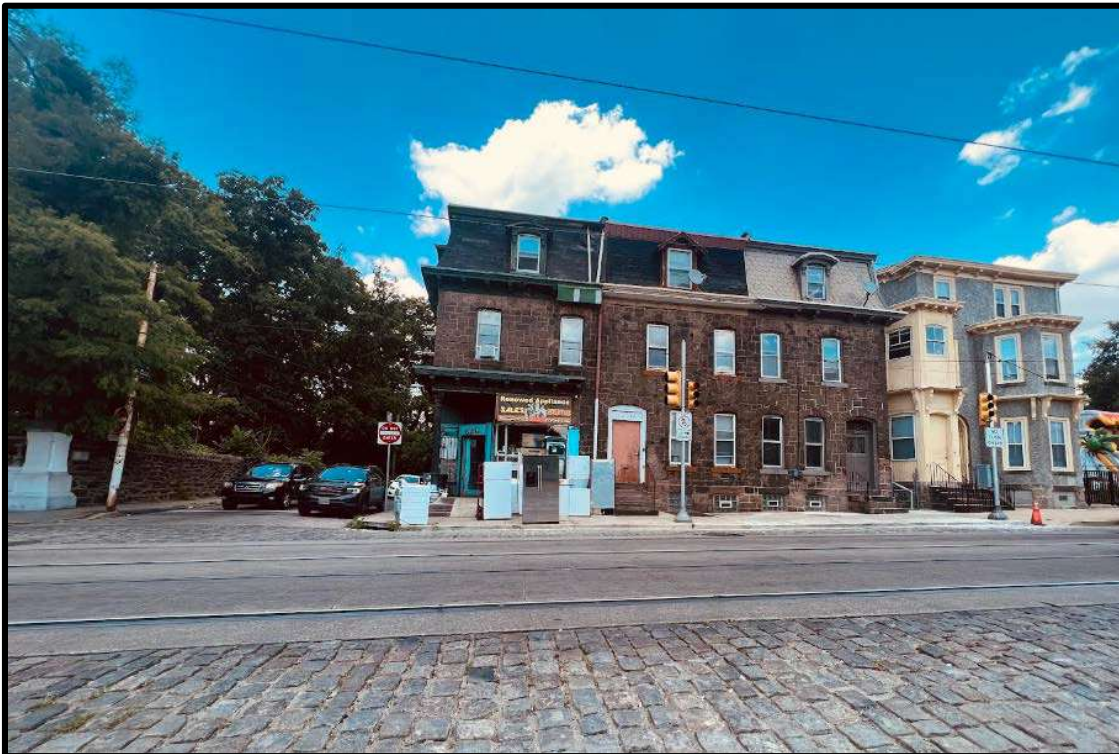
Figure 4. The primary (southwest) elevation of the subject property in context. Source: Keeping Society of Philadelphia, 2022.
