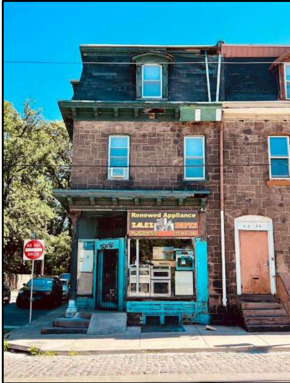
Figure 5. The primary (southwest) elevation. Source: Keeping Society of Philadelphia, 2022.
