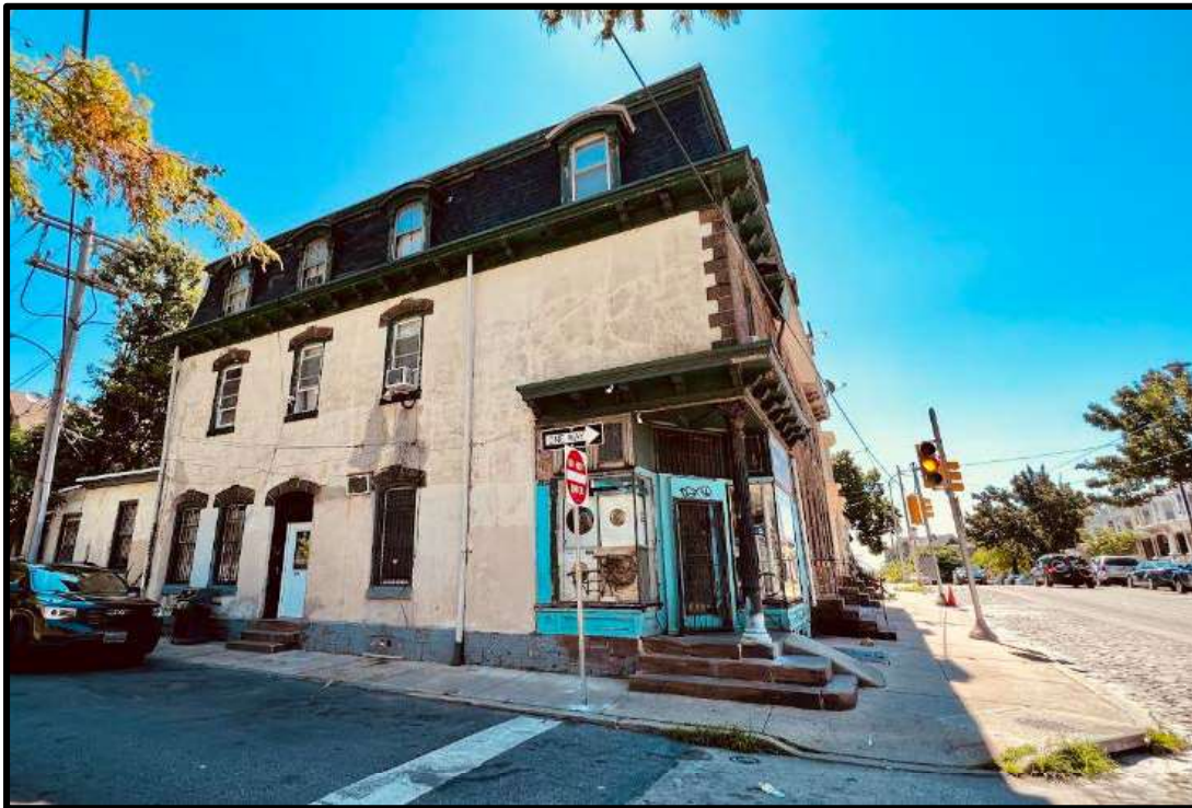
Figure 8. The side (northwest) elevation. Source: Keeping Society of Philadelphia, 2022.
