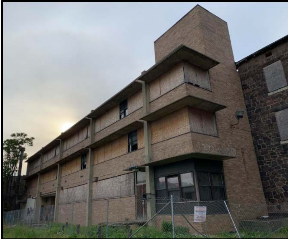
Figure 13. The south and east elevations of the Infirmary Addition. Source: Oscar Beisert, 2021.
