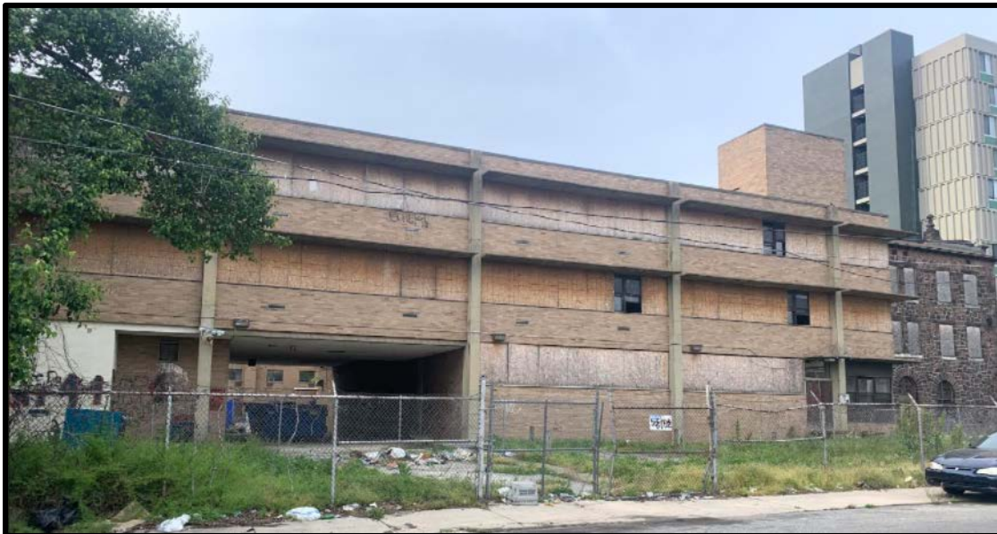
Figure 12. The south elevation of the Infirmary Addition. Source: Oscar Beisert, 2021.
