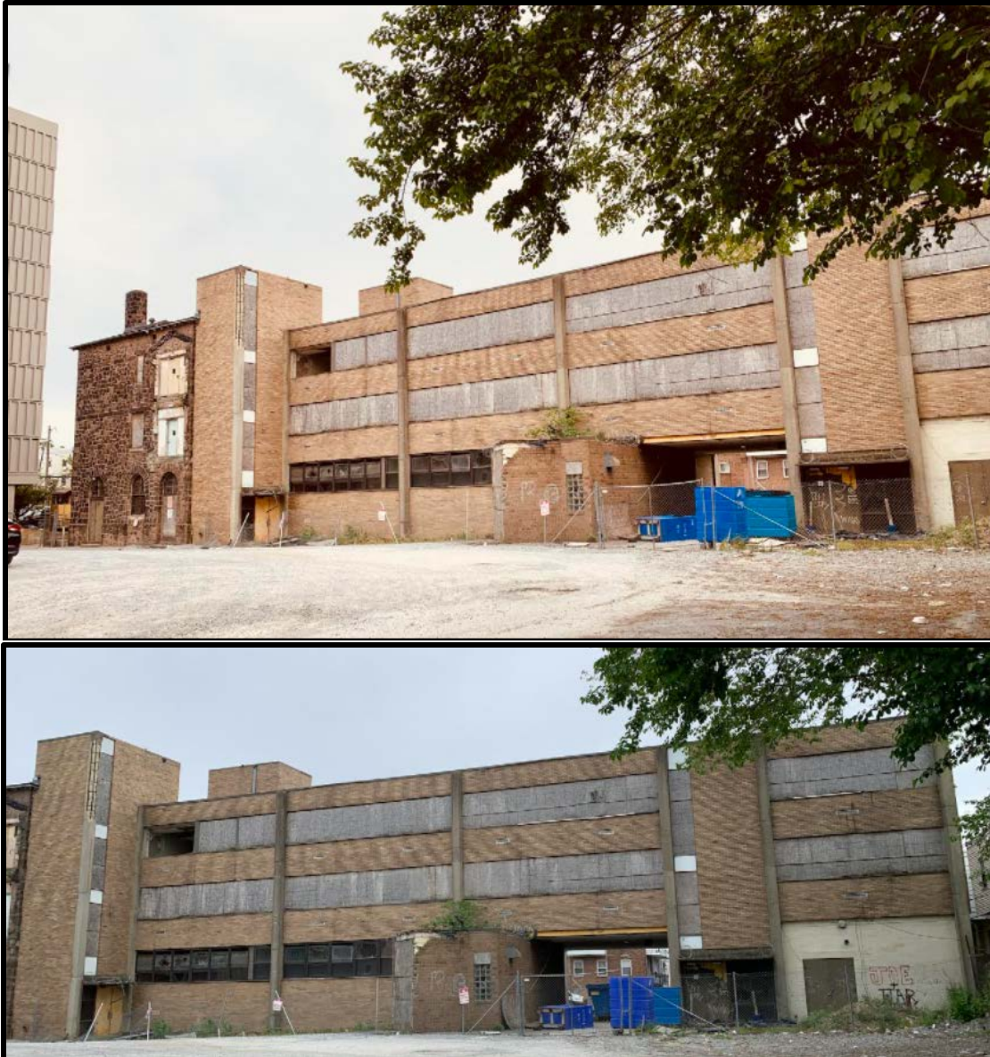
Figure 10. Top: The north elevations of the Infirmary and the Infirmary Addition. Source: Oscar Beisert, 2021. Figure 11. Bottom: The north elevation of the Infirmary Addition. Source: Oscar Beisert, 2021.
