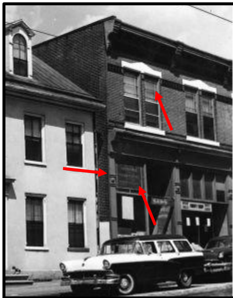
Figure 23. The subject building in 1957, showing the Queen Anne windows and the original storefront details. Source: The Philadelphia Historical Commission, 1957.
