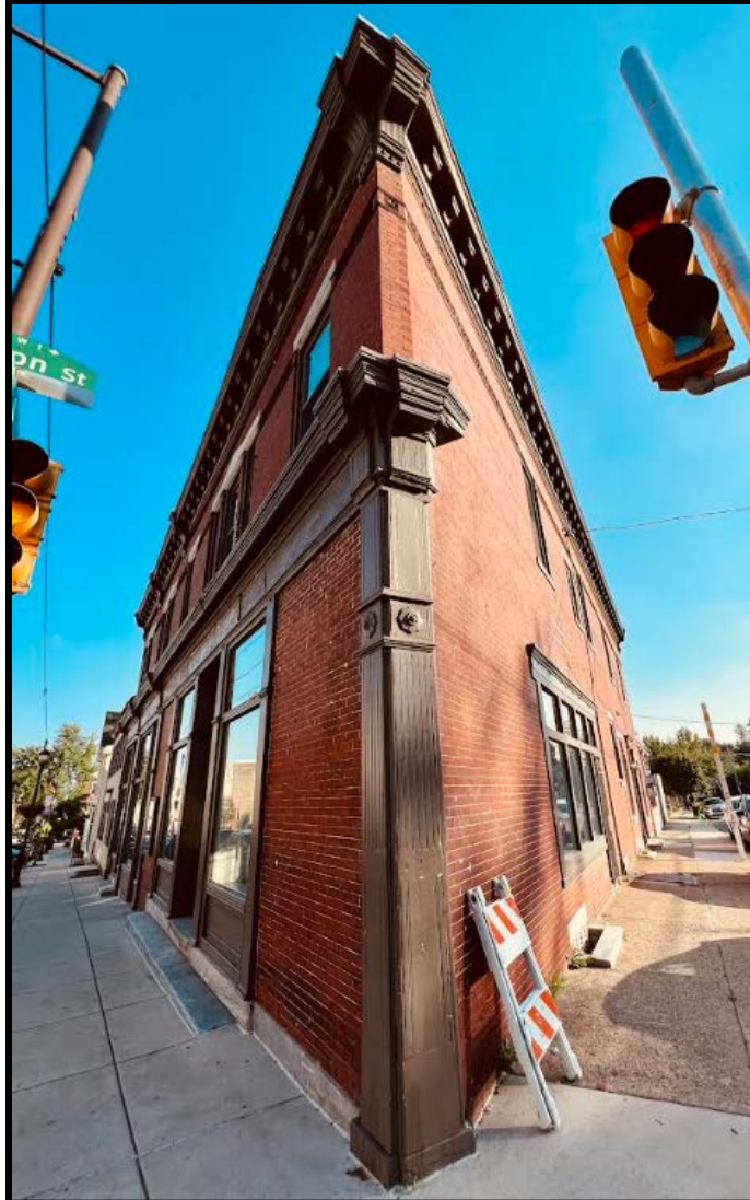
Figure 5. The primary (northeast) and side (northwest) elevations of the subject property. Source: Oscar Beisert, 2022.
