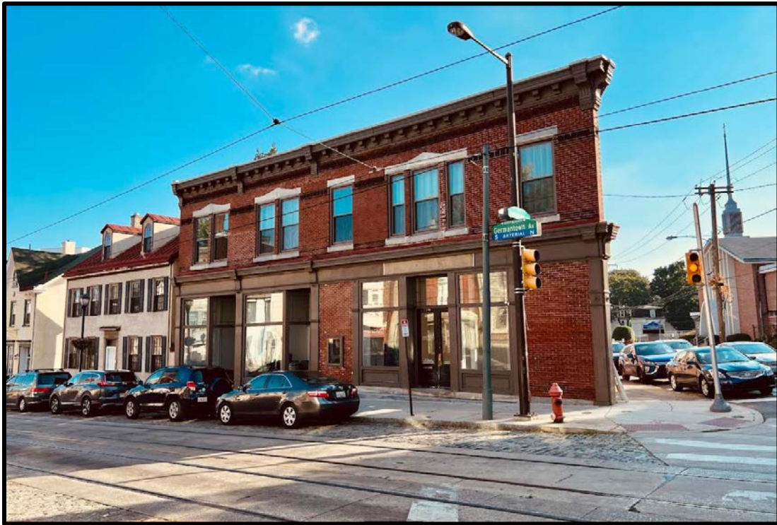
Figure 1. The primary (north) elevation of the subject property. Source: Oscar Beisert, 2022.
