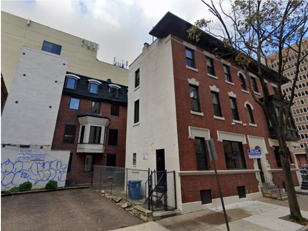
Figure 5 - 1700-02 Race Street, south and east elevations. The rear ell of 1704 Race Street is seen at far left.
