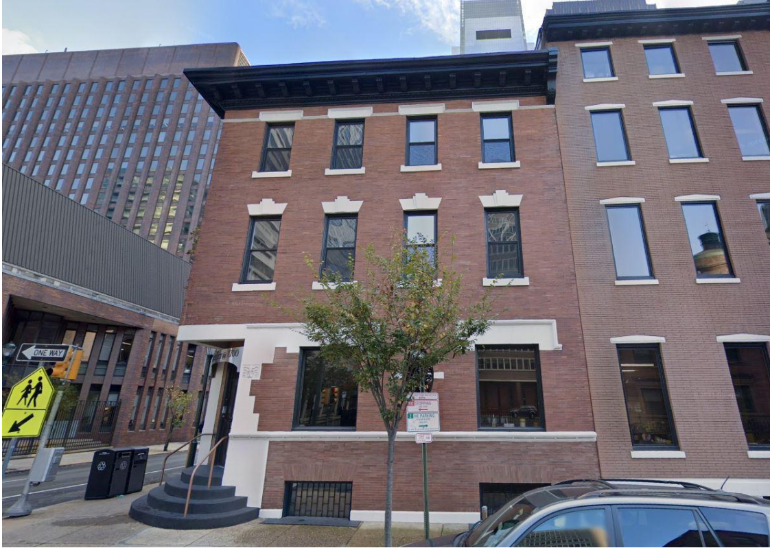
Figure 3 - 1700-02 Race Street, north elevation (facing Race Street).
