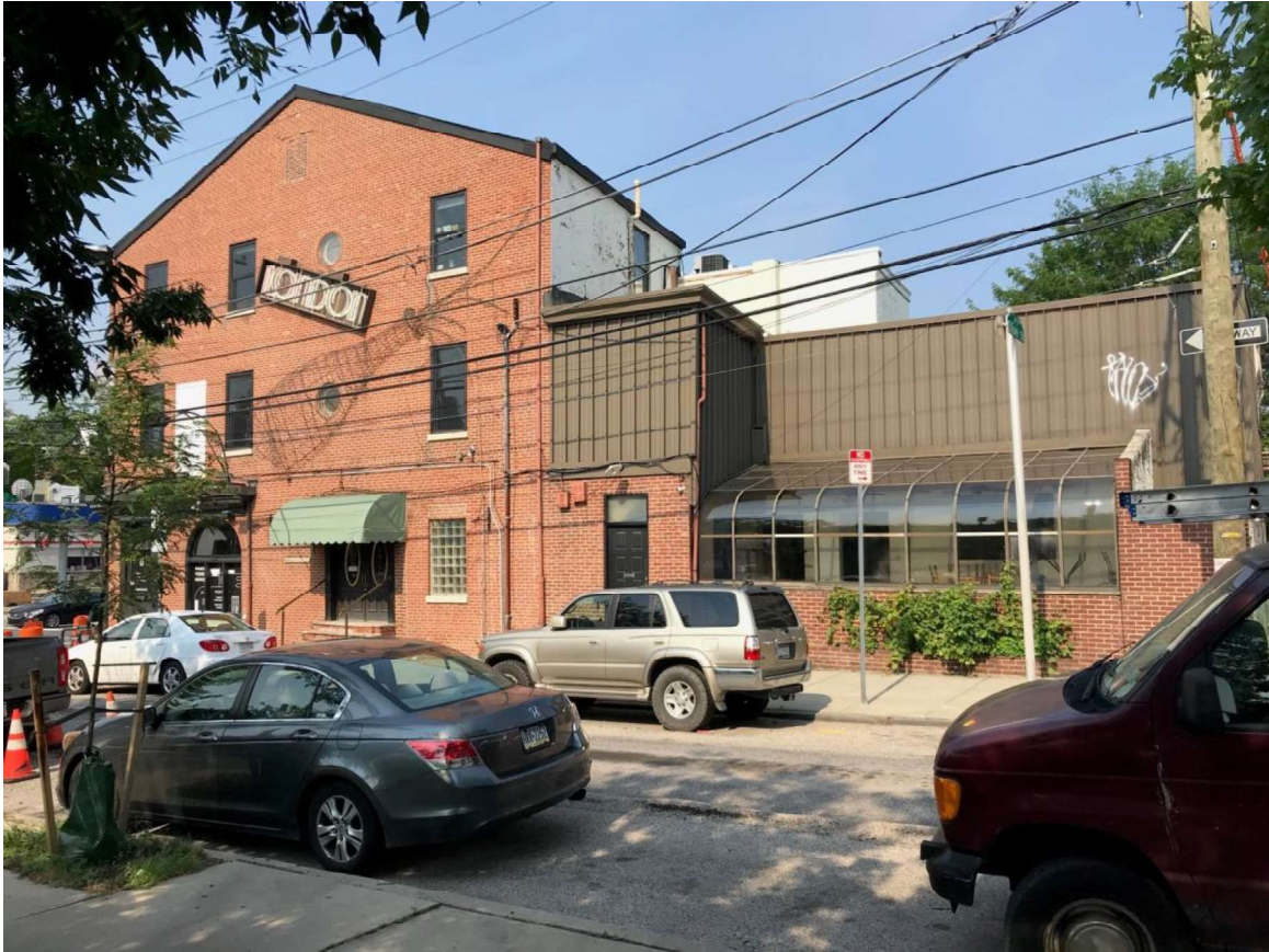
Figure 5 – East elevation, looking southwest from 23 rd Street.
