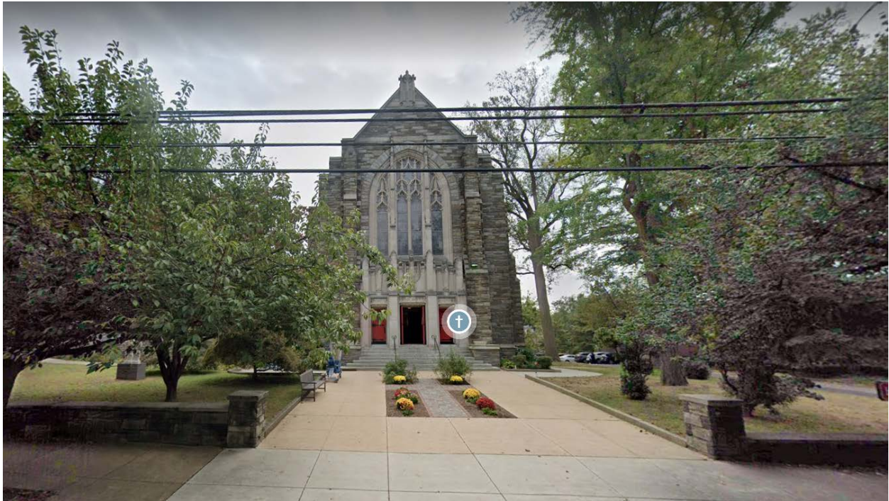
Front façade of the church building at 148-54 E. Mt. Airy Ave. (Source: Google StreetView, October 2019)
