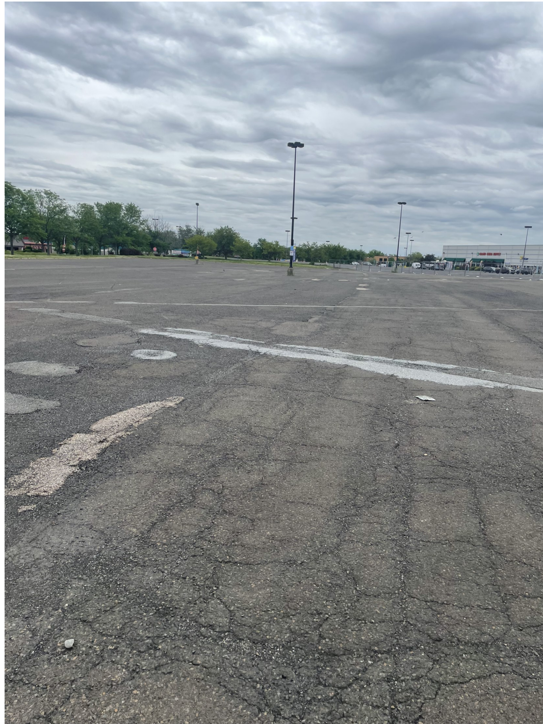
Photograph 7 – View looking south from within the existing parking lot.
