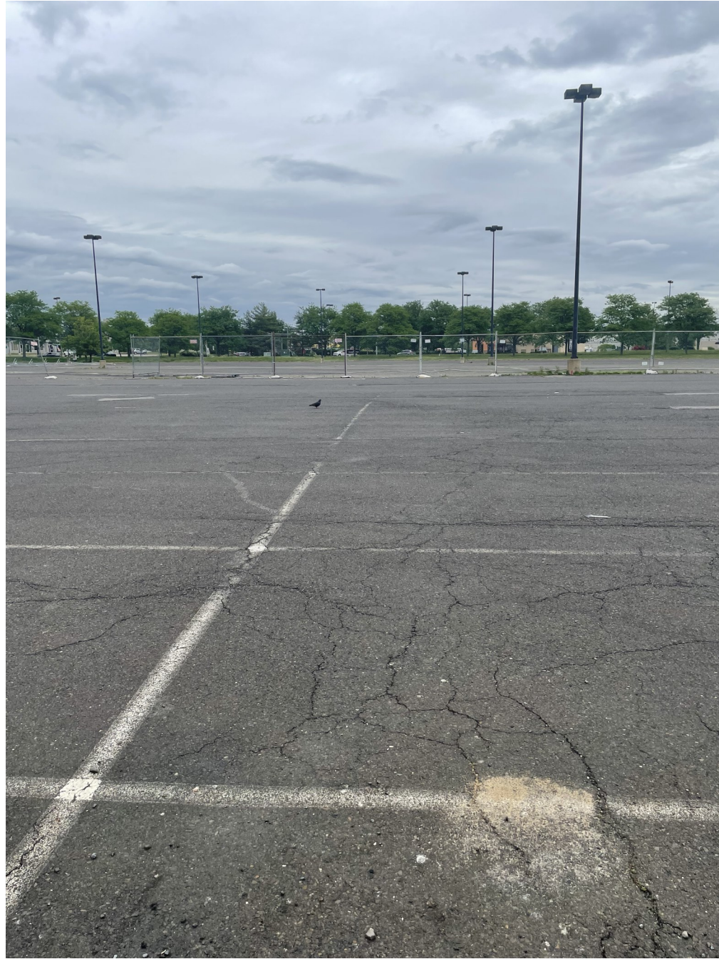
Photograph 4 - View looking northeast at the location of the proposed building into the site.
