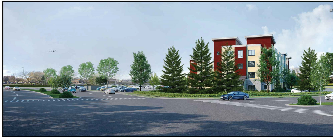
LIBERTY BELL BOULEVARD & FRANKLIN MILLS BOULEVARD STREET VIEW LOOKING NORTH
