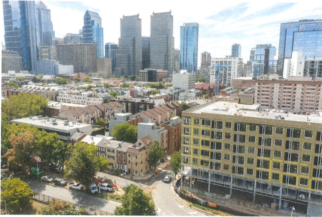
North elevation – building to left
