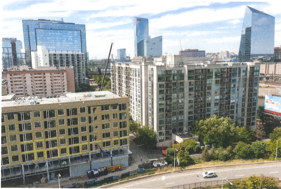
North elevation – building to right
