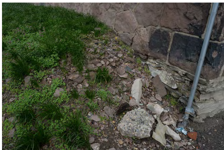
Removed bridge, unrepaired masonry where bridge removed, north façade; deterioration of brownstone, south façade.
