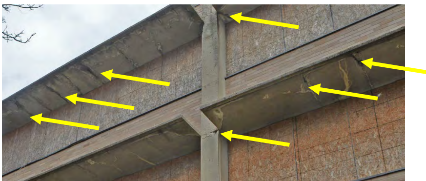
Dark lines where canopies are cracking with rebar rust and expansion; cracking of pier surfaces at floor level
