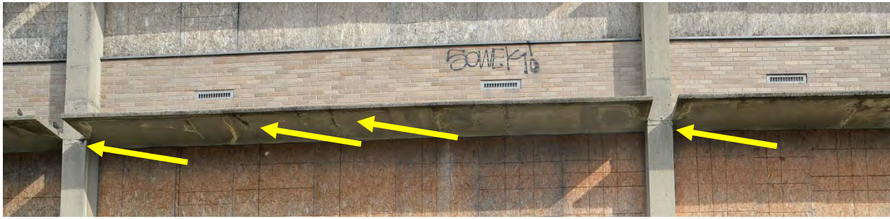
Additional rebar damage in canopies, cracking at floor levels in piers. Graffiti from interior access.
