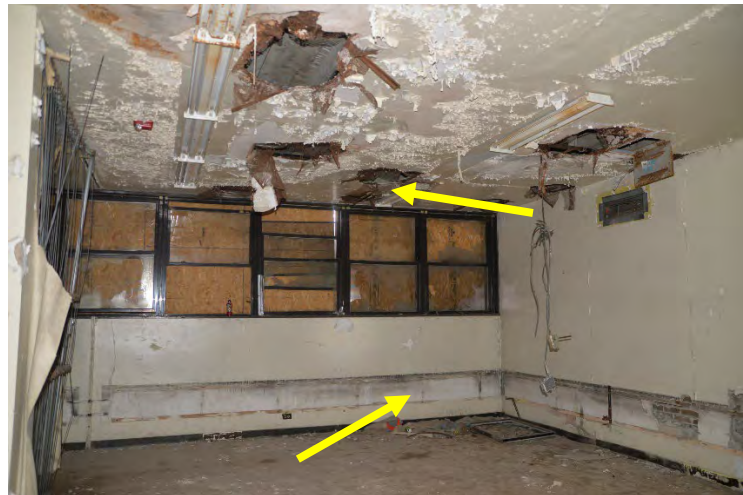
Interior water damage; rusted-out metal lath that would require the replacement of all of the interior wall and ceiling finishes; inoperable copper fin-tube radiators removed, all interior surfaces beyond repair
