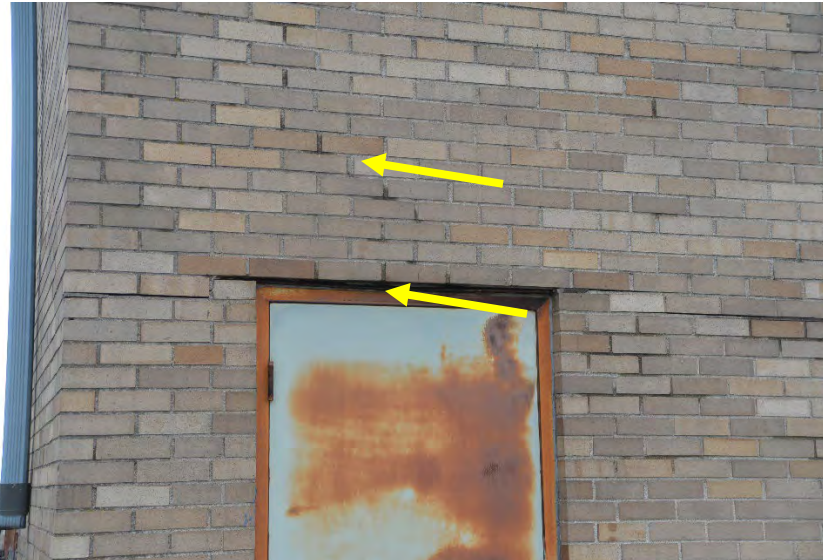
Rebar expansion from rust in concrete; lintel expansion with resultant masonry step-cracking above attic door
