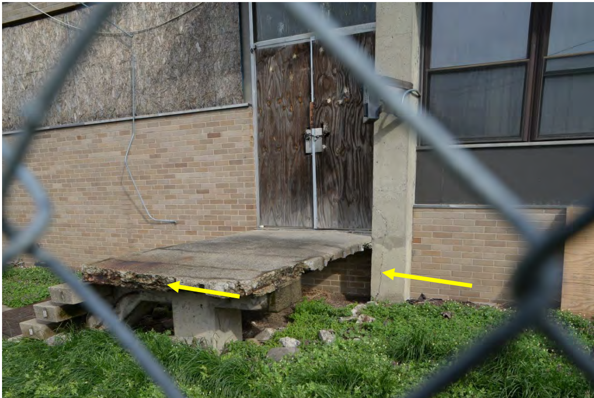
Significant rust jacking and destruction of rear platform suggestive of incipient failure in other unprotected concrete surfaces; pier cracking at ground.
