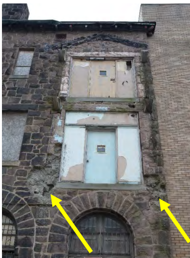
Removed bridge, unrepaired masonry where bridge removed, north façade; deterioration of brownstone, south façade.
