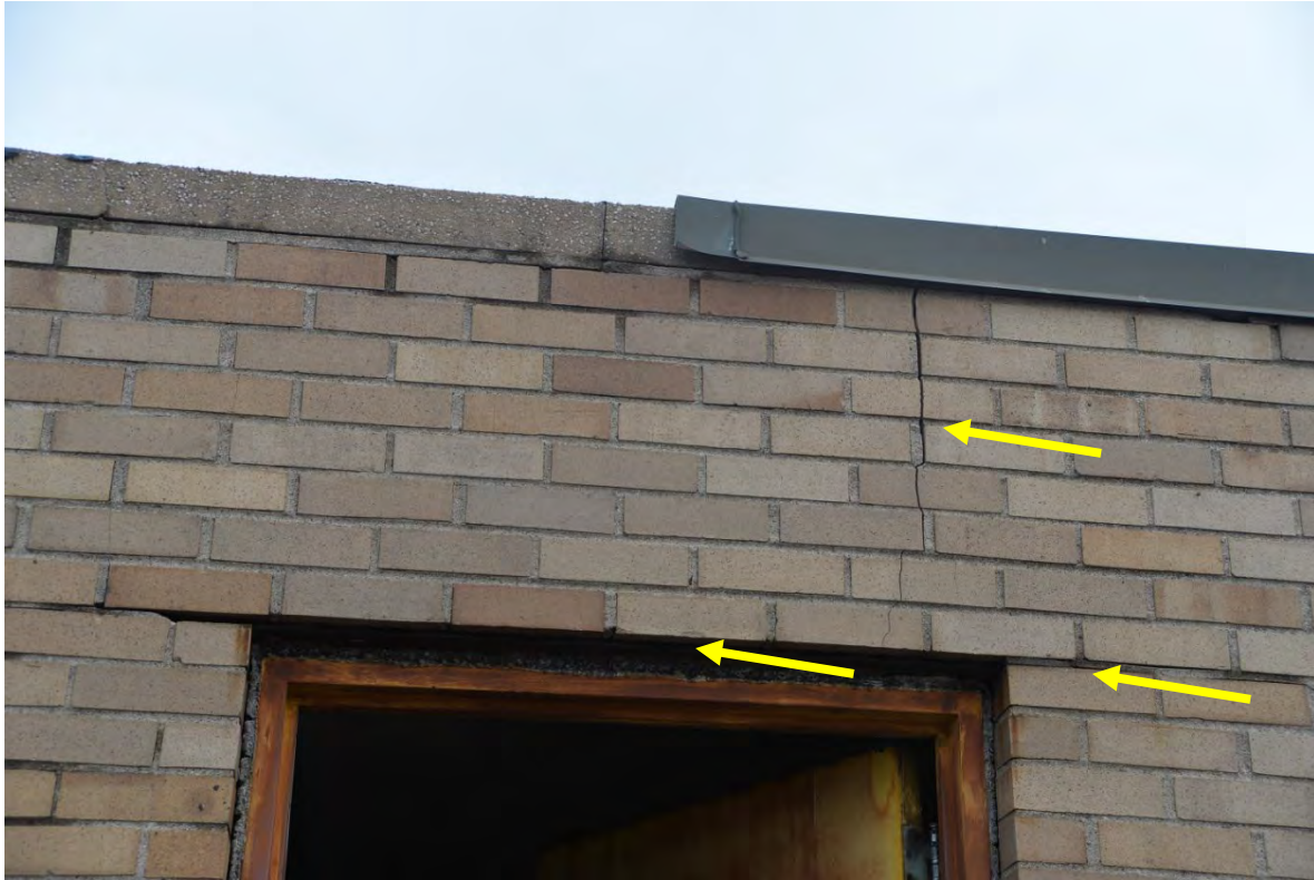
Rust jacking of lintel cracking bricks above with cast stone coping permitting water access into masonry
