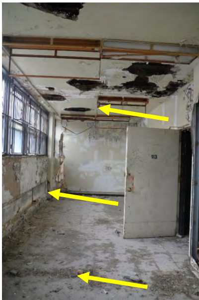
Interior water damage; rusted-out metal lath that would require the replacement of all of the interior wall and ceiling finishes; inoperable copper fin-tube radiators removed, all interior surfaces beyond repair
