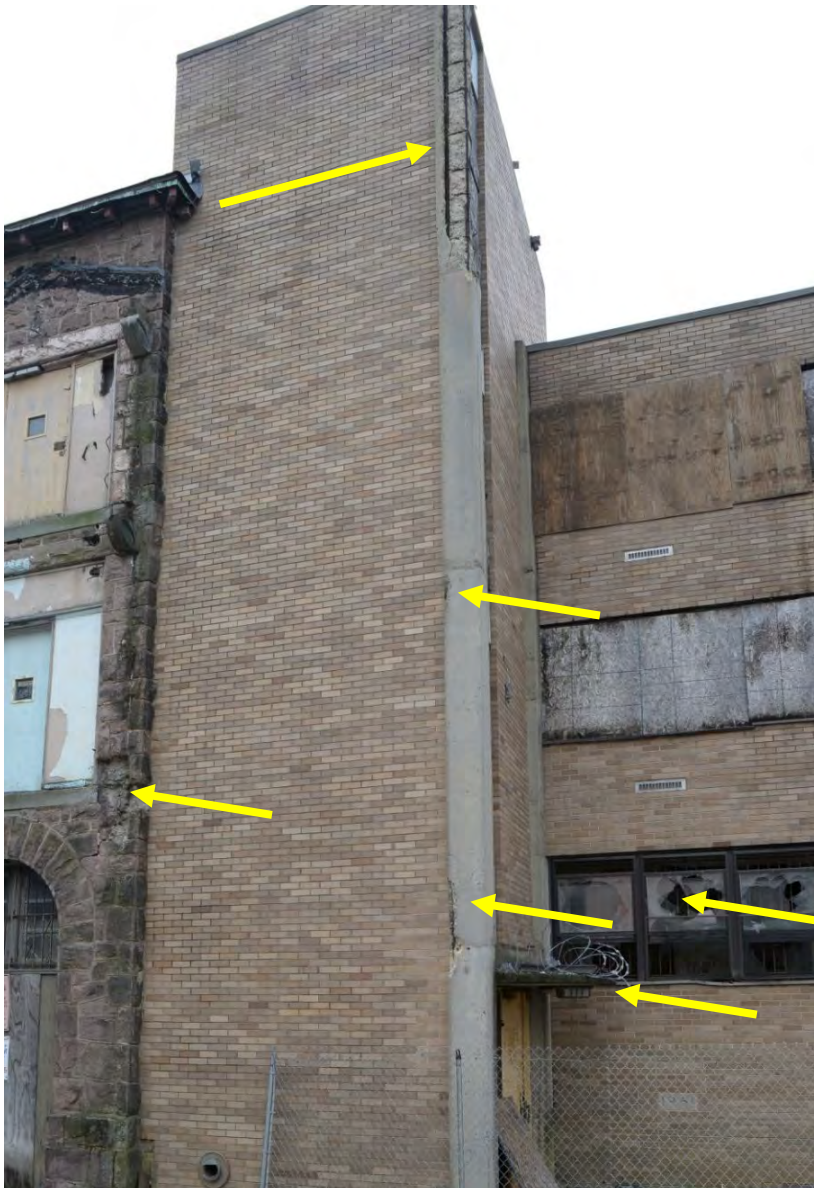
North side stair tower, rebar exposure, slenderness of canopy slab and water damage in canopy above doorway, modern replacement windows with smashed glazing; rust jacking at window heads; brutal removal of bridges from brownstone building with no attempt to repair the damage suggesting that reuse was never contemplated.
