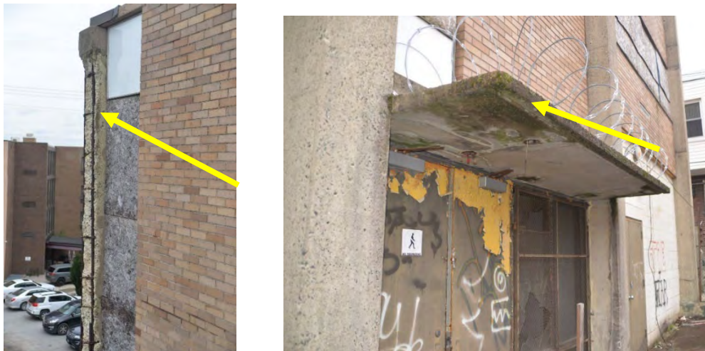
Rebar damage in stair tower and water penetration through cantilevered door canopy
