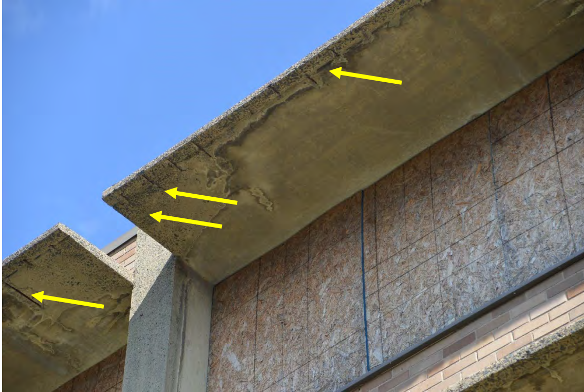
Detail sunscreens, water erosion of surface cement, rust damage to rebar
