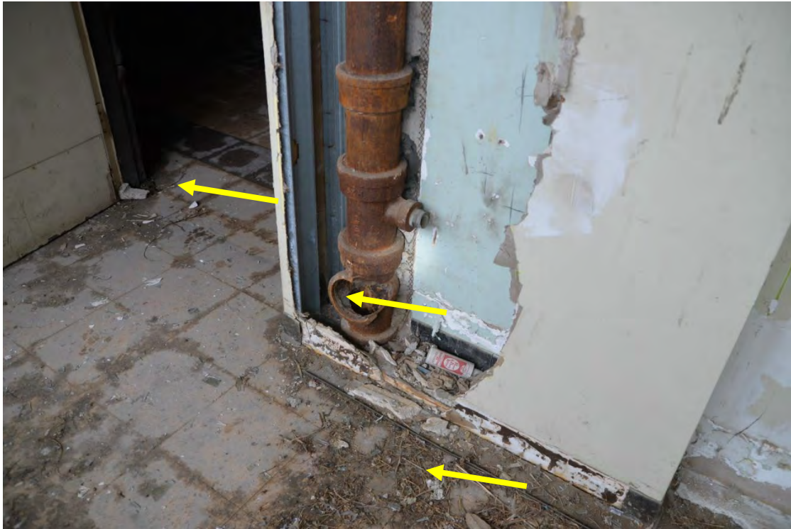
Interior vandalism, soil stacks smashed by vandals; evidence of water damage throughout building
