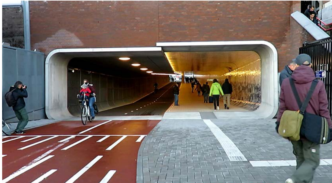
Bike Path Overhead Lighting
