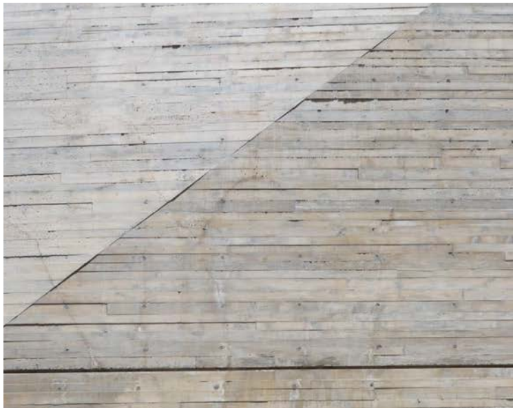
Abutment Wall Treatment: Board Formed Concrete Finish
