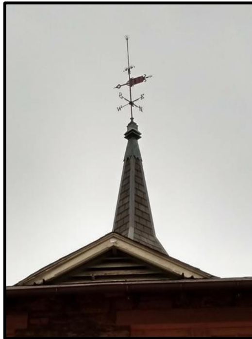
Figure 10: The ornamented spirelet of the taller of the two ventilation appliances
