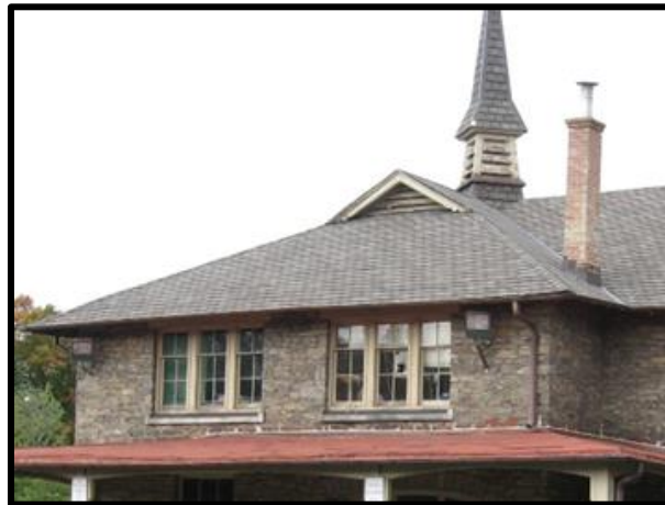
Figure 17. Showing similar gablet and hipped roof of the subject building.
