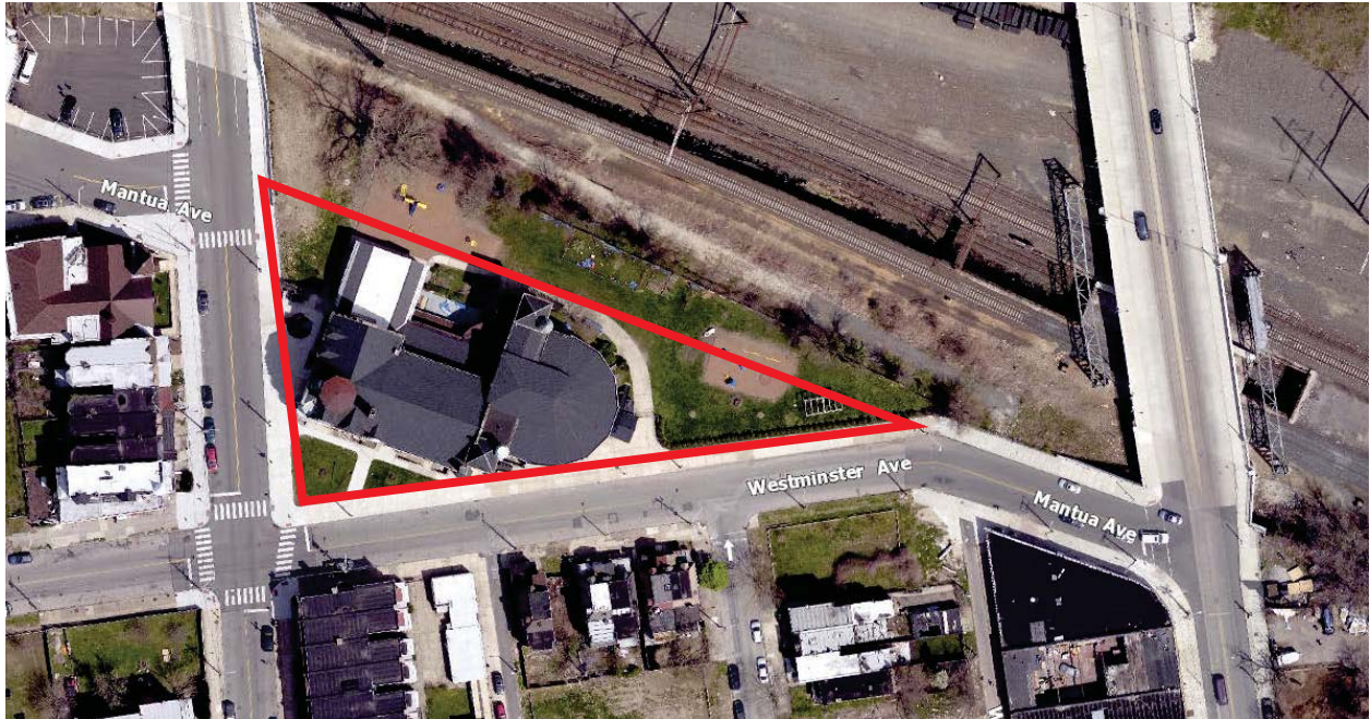
Figure 22: Aerial view of 40125-4069 Westminister Avenue. Source: City of Philadelphia Department of Records, CityGeo.
