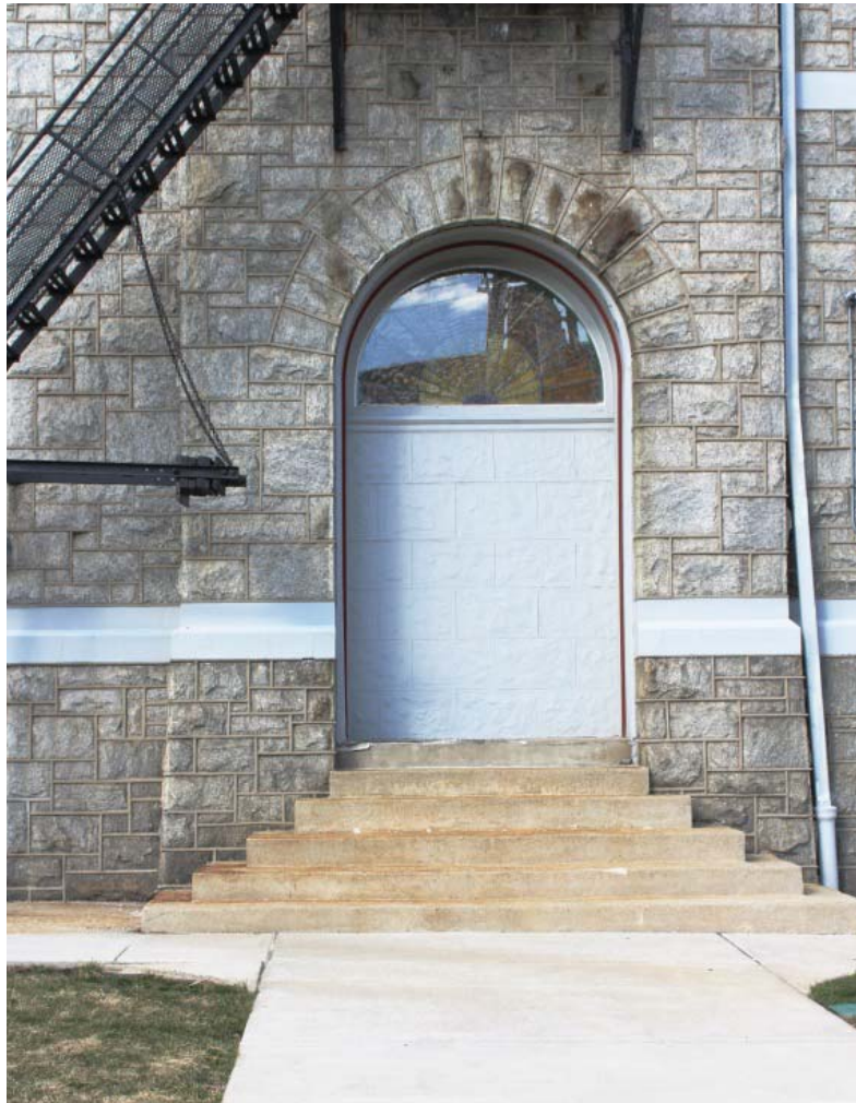
Figure 8: Infilled entry and transom. Source: Photo by Amanda Stevens, March 19, 2019.
