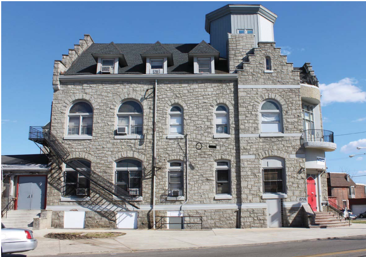
Figure 11: West façade of 4025-69 Westminster. Source: Photo by Amanda Stevens, March 19, 2019.
