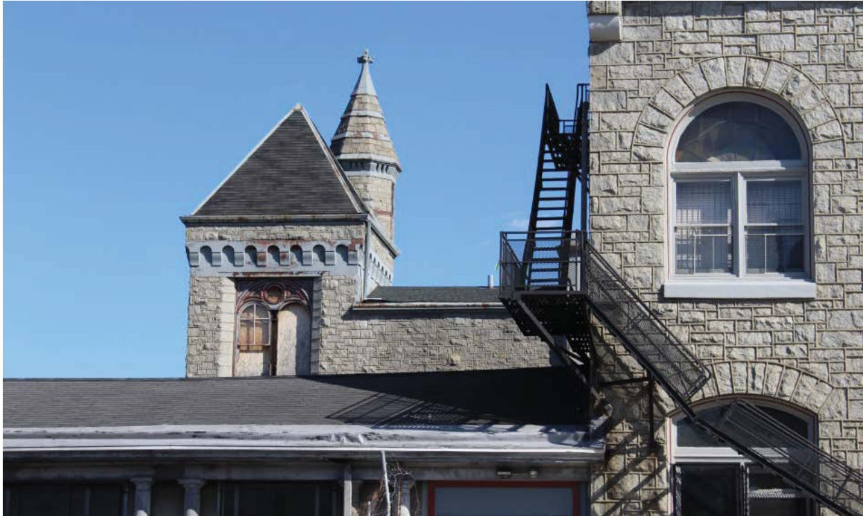
Figure 13: View of north towers. Source: Photo by Amanda Stevens, March 19, 2019.
