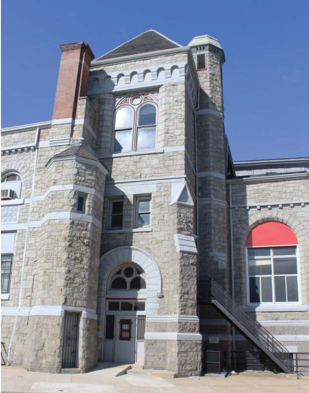
Figure 10: Multiple tower structures on the south elevation. Source: Photo by Amanda Stevens, March 19, 2019.
