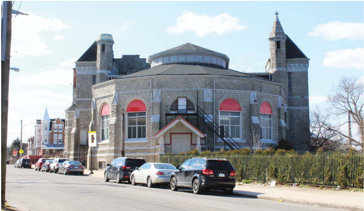
Figure 14: View looking west at auditorium. Source: Photo by Amanda Stevens, March 19, 2019.
