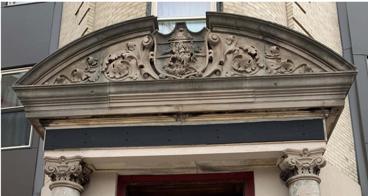
Main entrance at the corner of 638 Christian Street, February 2019. The carved cartouche above the doorway has floral motifs alongside the coat of arms for the Region of Calabria. Saint George on horseback, slaying a long-tailed dragon, identifies the southern-most region of Italy, Calabria.
