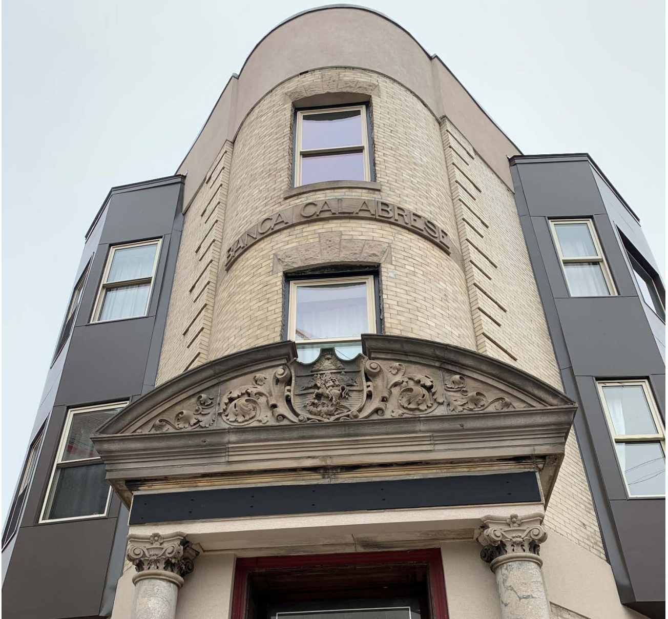
“Banca Calabrese” is legible on the mounted stone band, which follows the contour of the rounded corner, February 2019.
