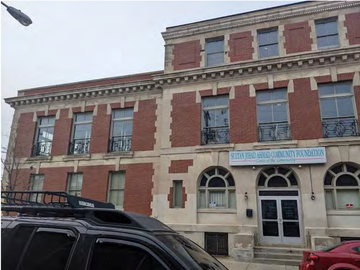
Figure 3. Photograph of the front-façade of the structure facing east across 19 th Street, north of W. Oxford. Note the brick and stone masonry, the modillions lining uniformly above the structure’s second floor, the double sash windows, and the symmetry of the windows on the third floor above the center of the structure. Photographs are attributable to the author unless otherwise specified.
