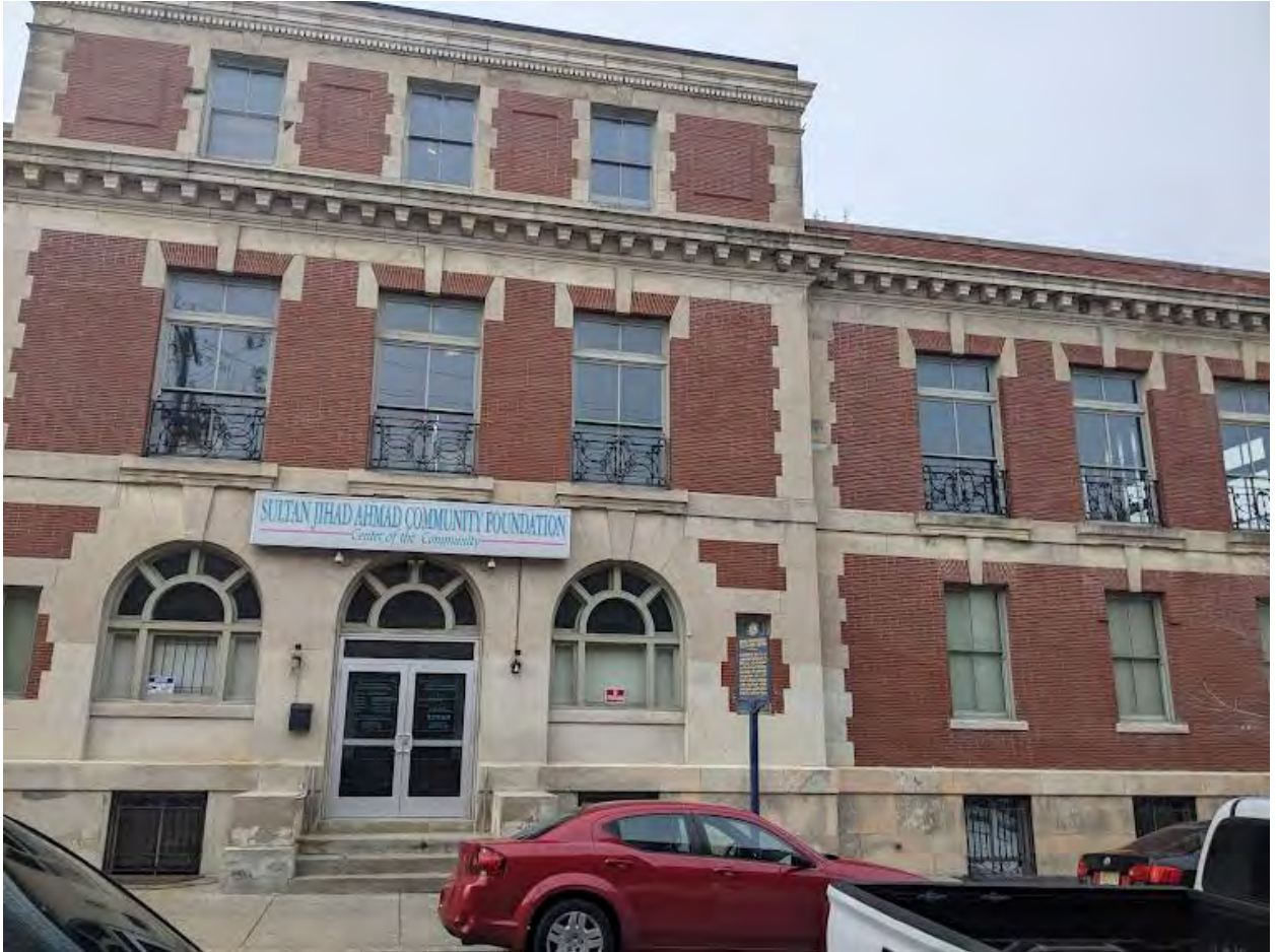
Figure 4. Photograph of the structure at 1901 W. Oxford Street, facing the northern two-thirds of the structure along 19 th Street, north of W. Oxford Street. Note the contrast in the cornices above the second and third floors; above the second floor is lined with modillions beneath the cornice, and beneath the cornice above the third floor are more tightly packed dentils.
