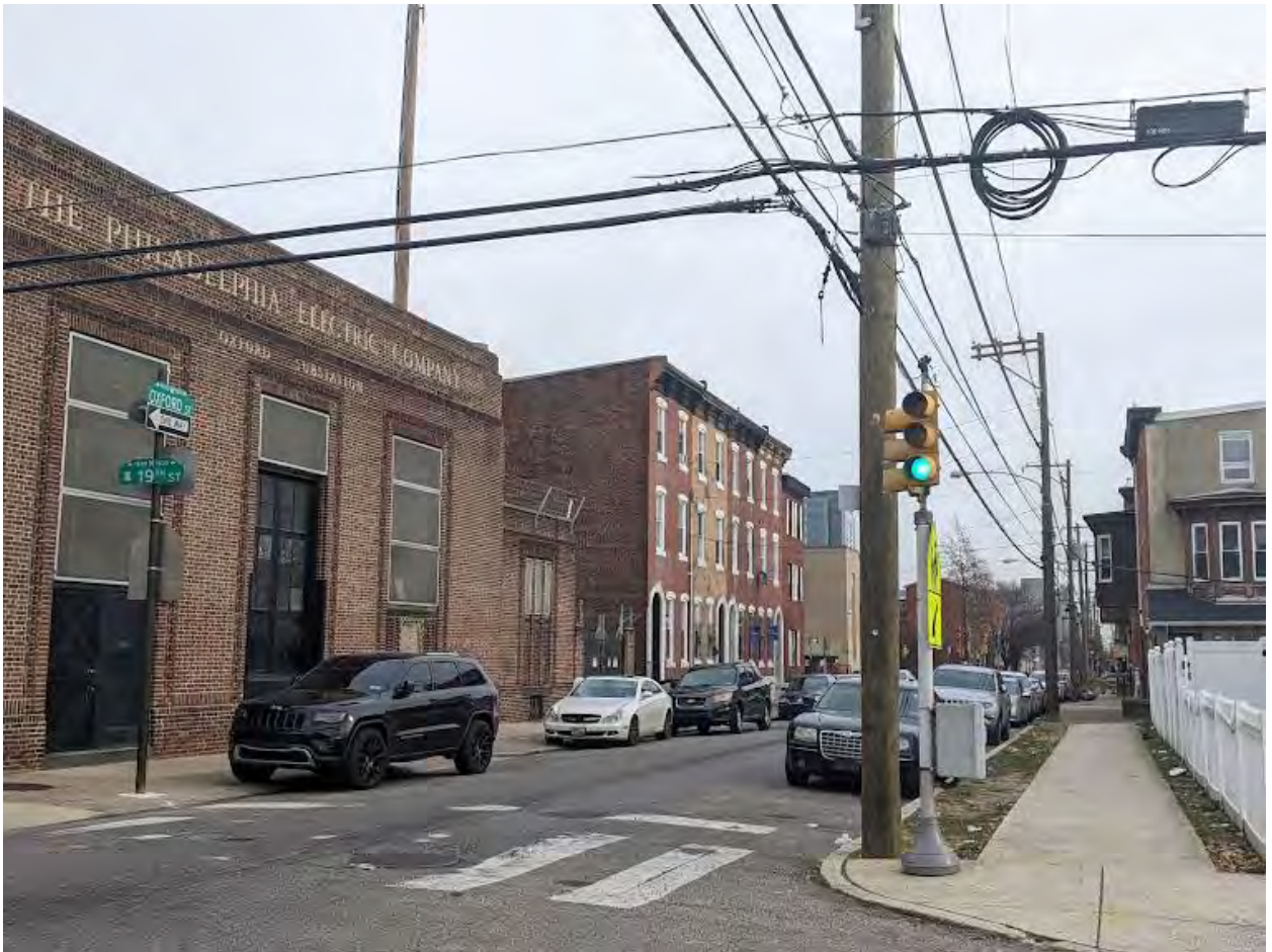
Figure 8. Photograph of the Philadelphia Electric Company’s substation at 19 th and W. Oxford Street, facing east from the southwest corner of 19 th and W. Oxford Street. The substation here was constructed as the city’s neighborhoods required increased access to electricity c. 1926. The row-homes visible beyond exhibit similar characteristics of Colonial Revival style, further contributing to 1901 W. Oxford Street’s connection to the setting.
