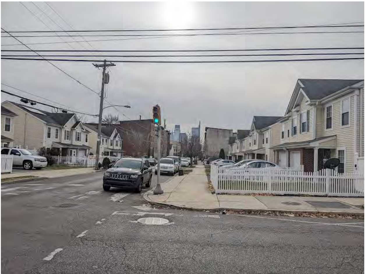
Figure 6. Photograph from the southern end of the structure at 1901 W. Oxford Street, facing south from the northwest corner of 19 th and W. Oxford Streets. Although the neighborhood was first developed residentially in the nineteenth and early twentieth
