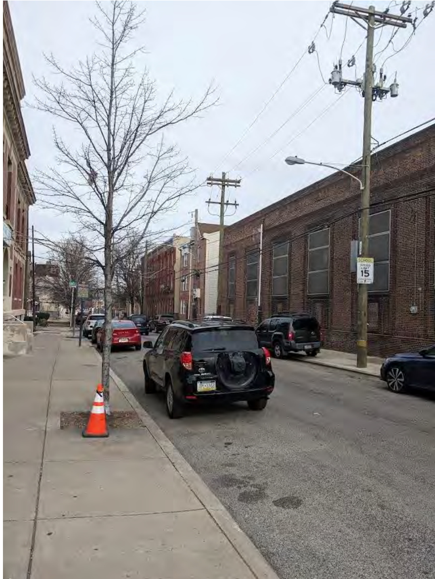
Figure 13. Photograph facing north along 19 th Street with 1901 W. Oxford Street at left and the Philadelphia Electrical Company Substation at right. Further down the street additional Colonial Revival, brick and masonry rowhomes are visible, further solidifying
