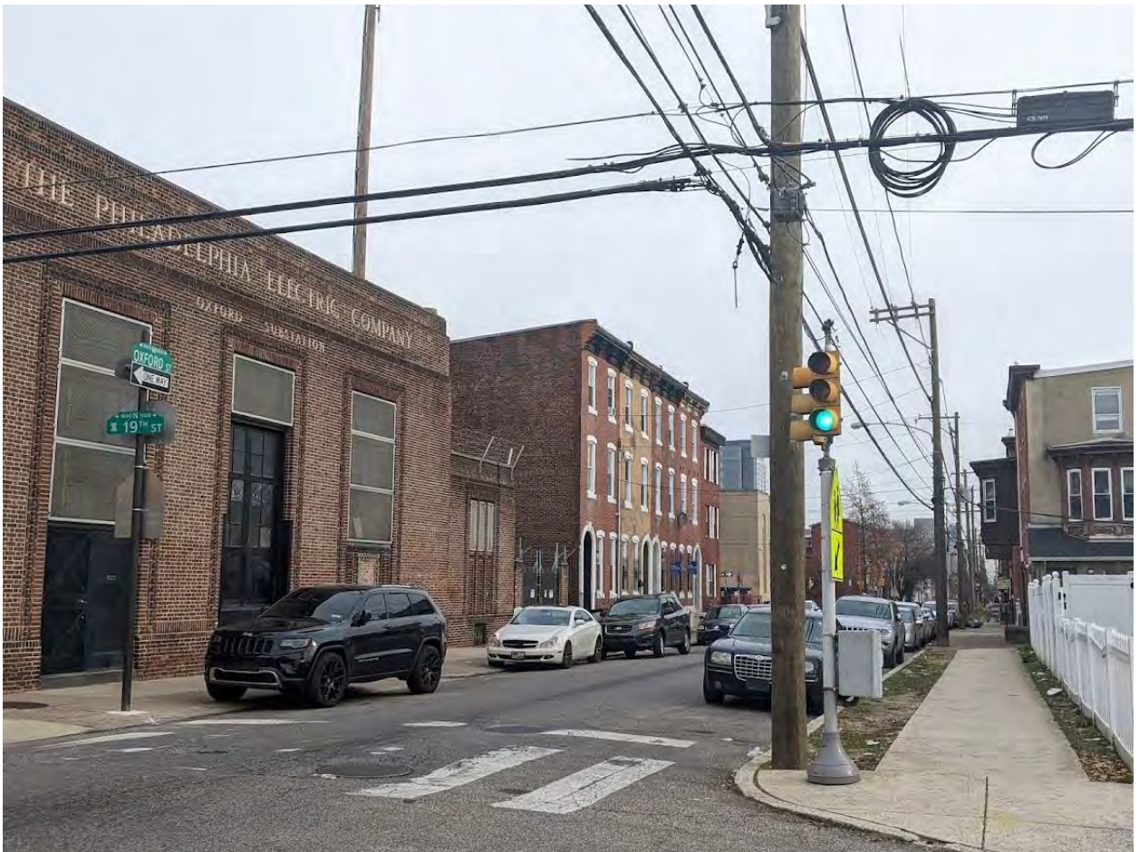
Figure 14. Photograph featuring the aforementioned 19 th and W. Oxford Sts. Power Station of the Philadelphia Electrical Company, and additional Colonial Revival rowhouses east of 1901 W. Oxford Street along W. Oxford Street, further situating the structure's style within a compatible setting.
