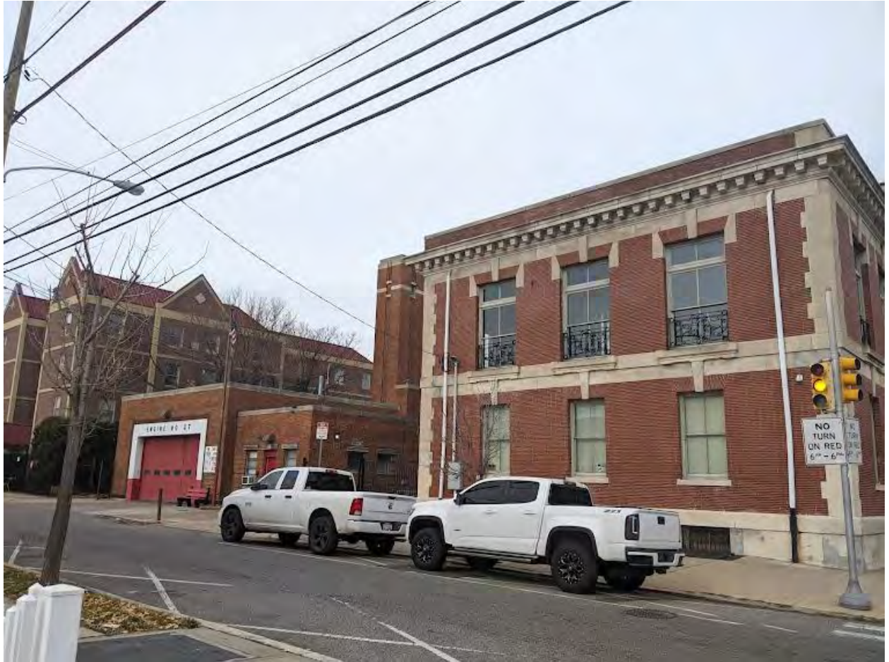
Figure 7. Photograph of the structure at 1901 W. Oxford Street (right) and the firehouse (left) facing northwest from the southwest corner of 19 th and W. Oxford Street. In the nineteenth century these two properties sat on the same parcel which served as stables, but were subsequently sold to the city and redeveloped as a firehouse and police station and jailhouse.
