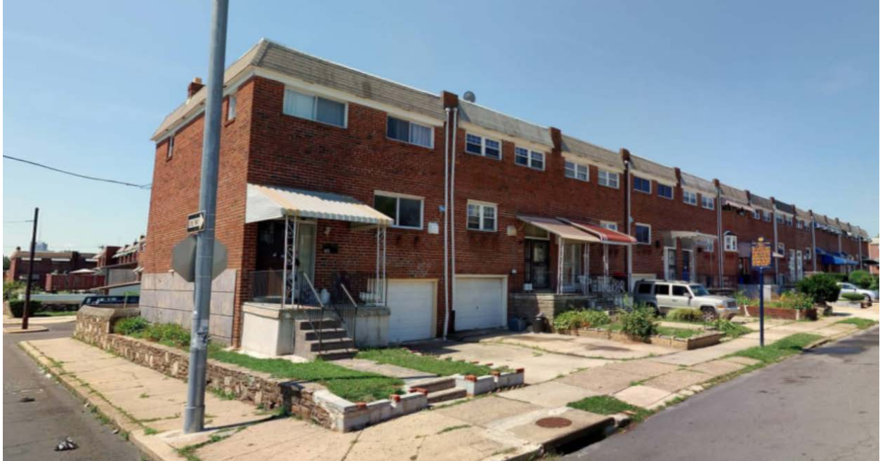
Figure 5. View looking southwest toward the south side of the 1100-block of Master Street, July 16, 2019. Source: Cyclomedia.
