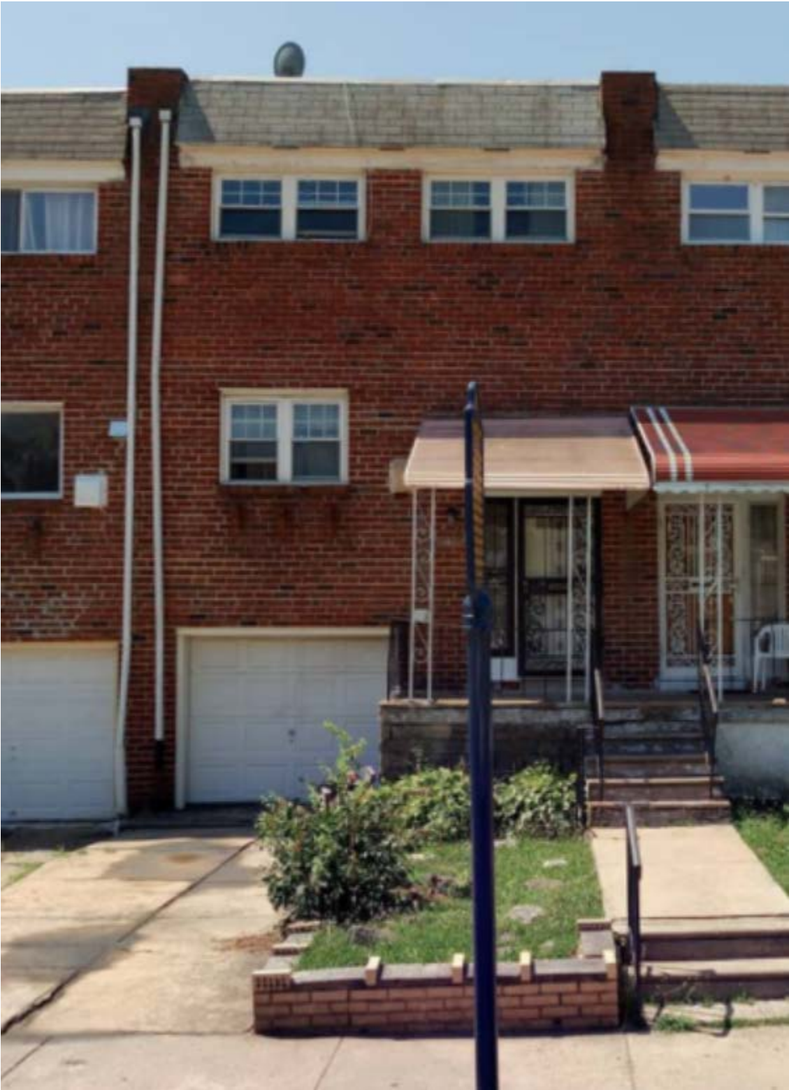
Figure 4. View of front façade at 1102 Master Street, July 16, 2019. Source: Cyclomedia.
