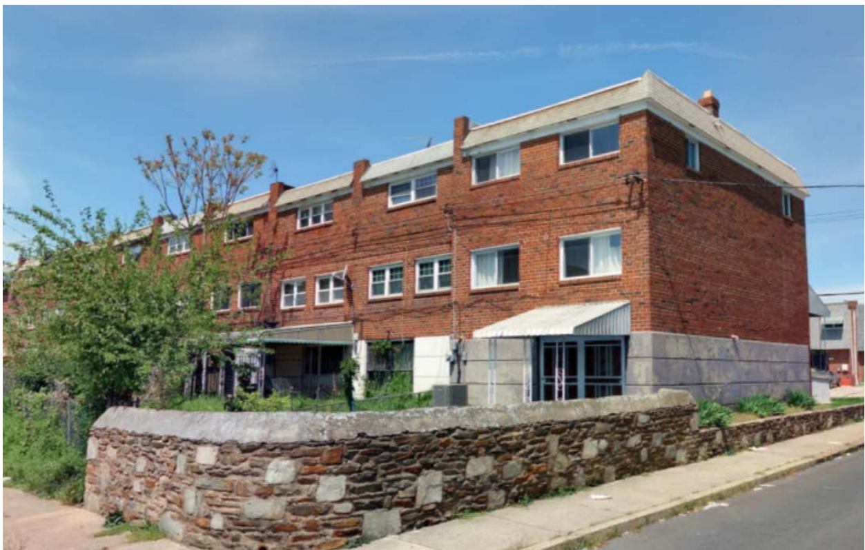
Figure 6. View looking northwest at the rear facades of 1100-block of Master Street, May 2, 2020. Source: Cyclomedia.
