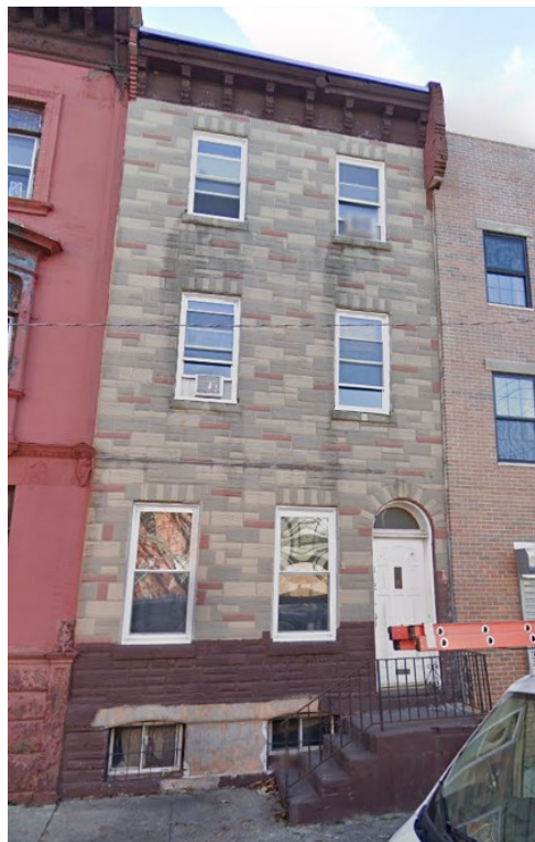
Example of 1.b.ii: The PermaStone veneer at 1842 Christian Street has been attached to the original façade rather than replacing it; the older façade remains underneath.
