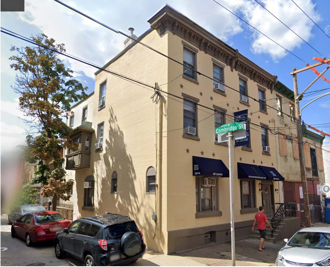
Figure 3: View at the corner of N. 19th St & Cambridge St
