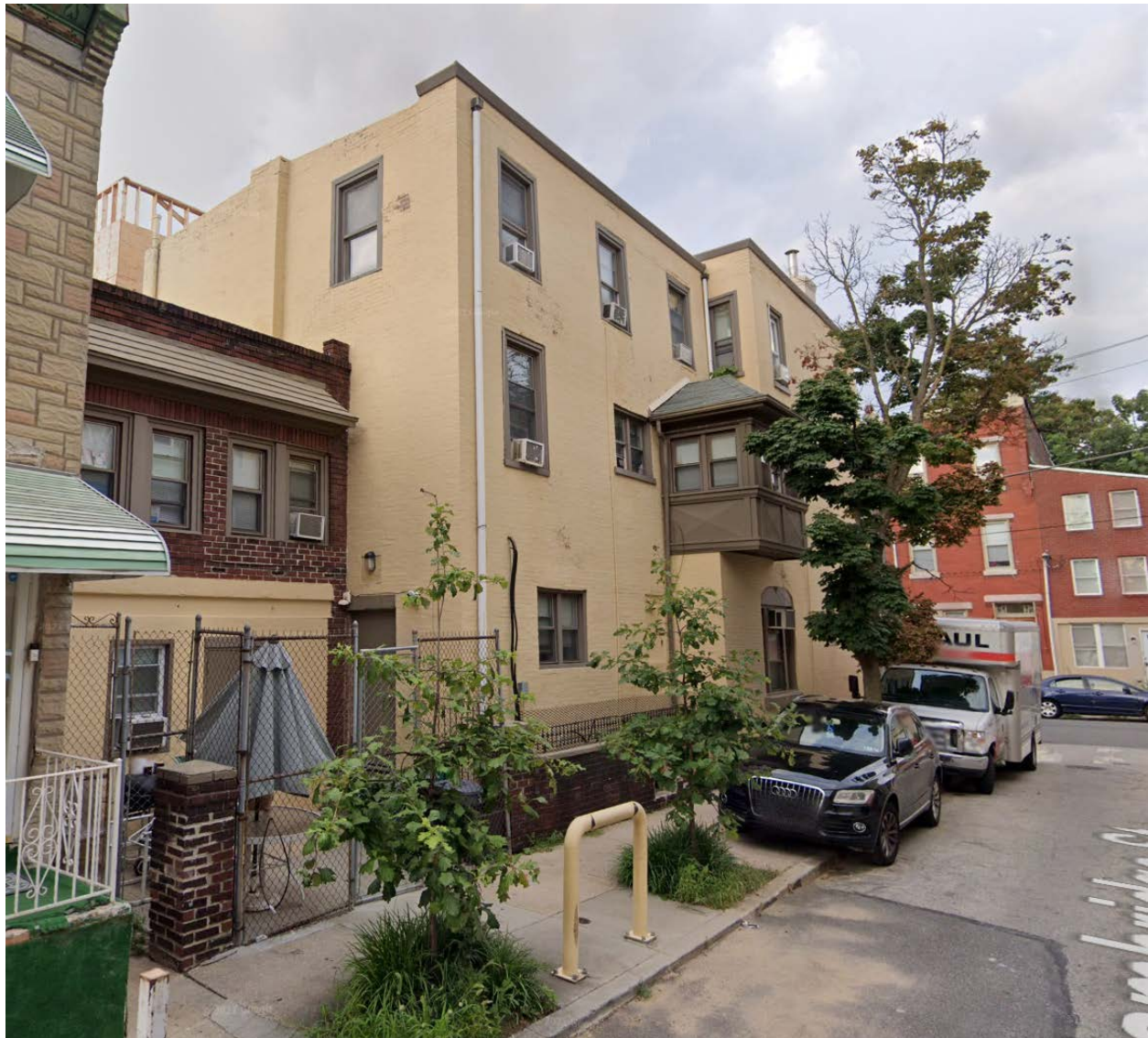
Figure 5: View along Cambridge Street towards N. 19th Street, note the projecting bay window at the second story
