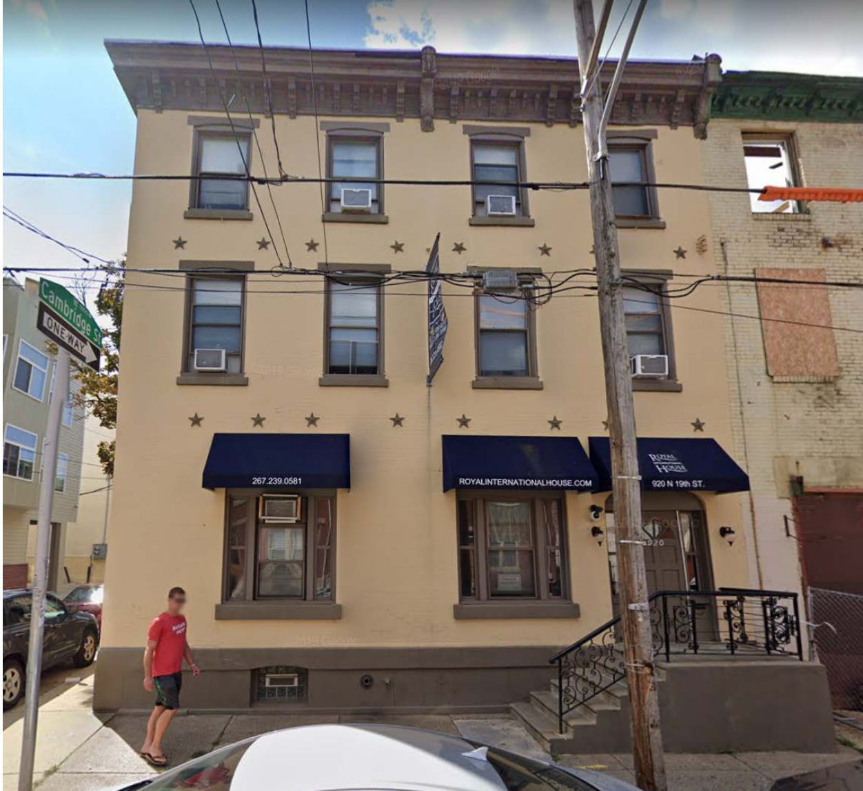
Figure 2: Primary facade along N. 19th St, note the double-wide rowhouse
