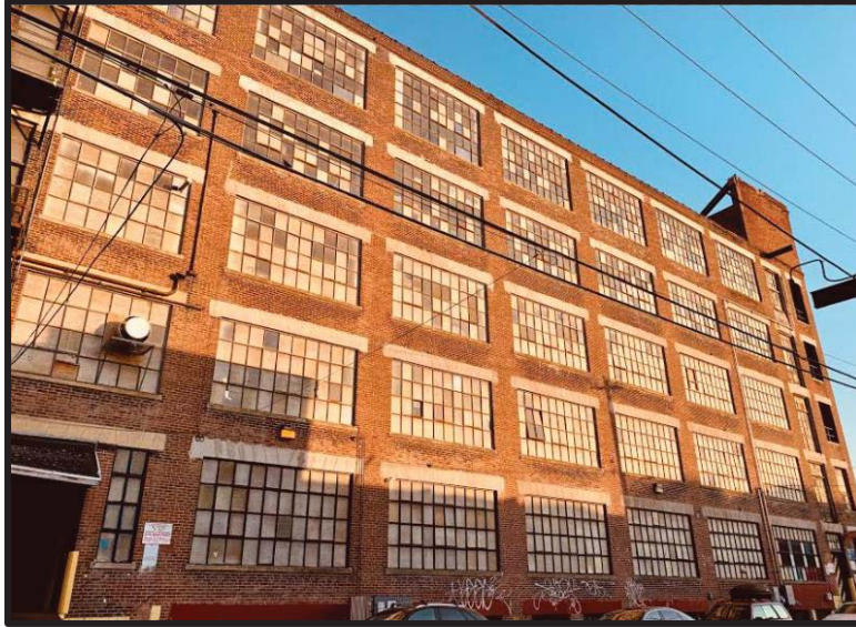
Figure 36. The west elevation of Building 5. Source: Oscar Beisert, 2021.
