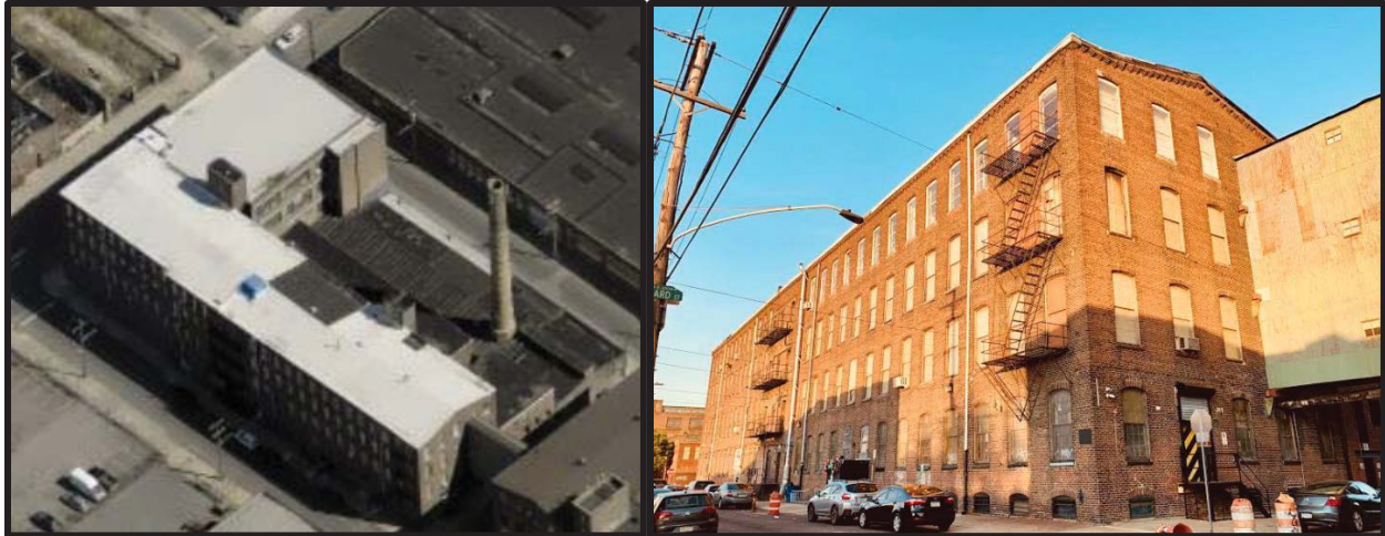
Figure 16. Looking northeast at 2095 E. Willard Street. Source: Pictometry, Atlas, City of Philadelphia. Figure 17. Right: Looking northeast at Buildings 1 and 1a at the northeast corner of Amber and E. Willard Streets. Source: Oscar Beisert, 2021.
