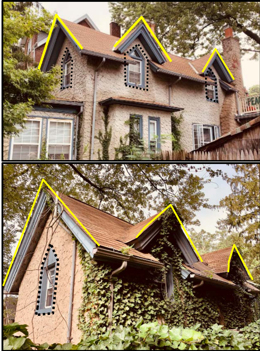
Figures 1 and 8. The above photographs are enhanced to highlight various characteristics of the Gothic Revival style, including yellow outlines on the gable ends and gable front wall dormers, as well as dotted lines on the Gothic Revival style triangular top arched windows. Top: Looking east at the southwest elevation. Source: Oscar Beisert, 2021. Bottom: Looking northwest at the southeast and northeast elevations. Source: Oscar Beisert, 2021.
