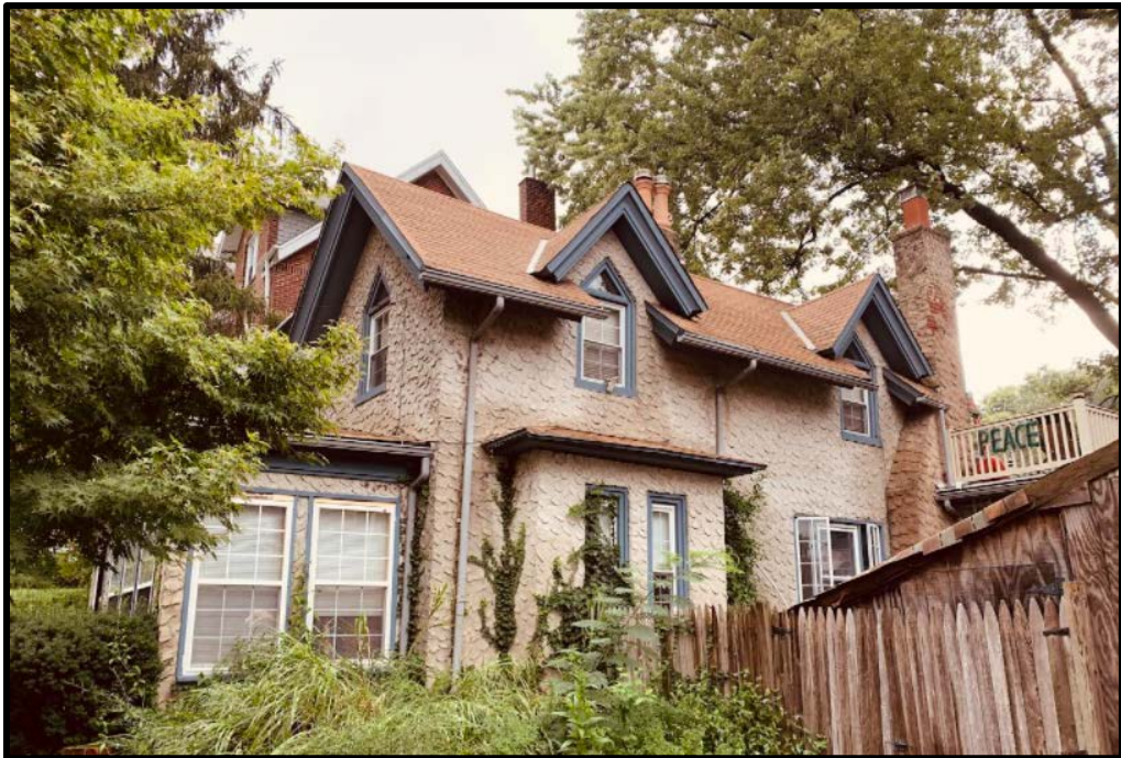
Figure 1. Looking east at the northwest and southwest elevations. Source: Oscar Beisert, 2021.
