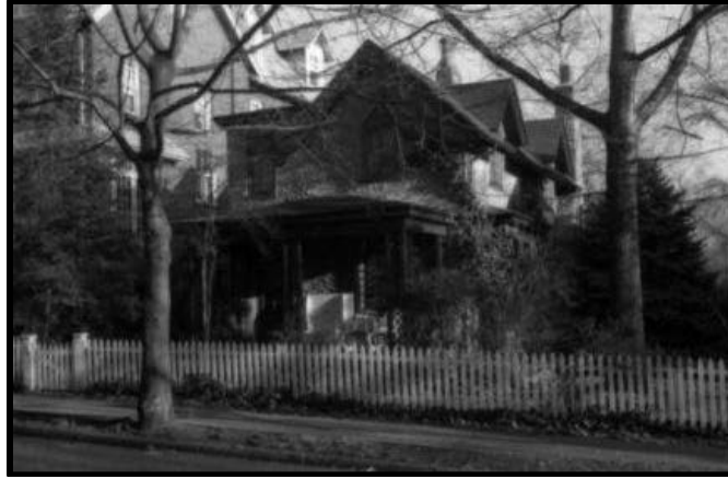
Figure 13. The northwest elevation, ca.1960s. Source: Philadelphia Historical Commission via PhillyHistory.org.
