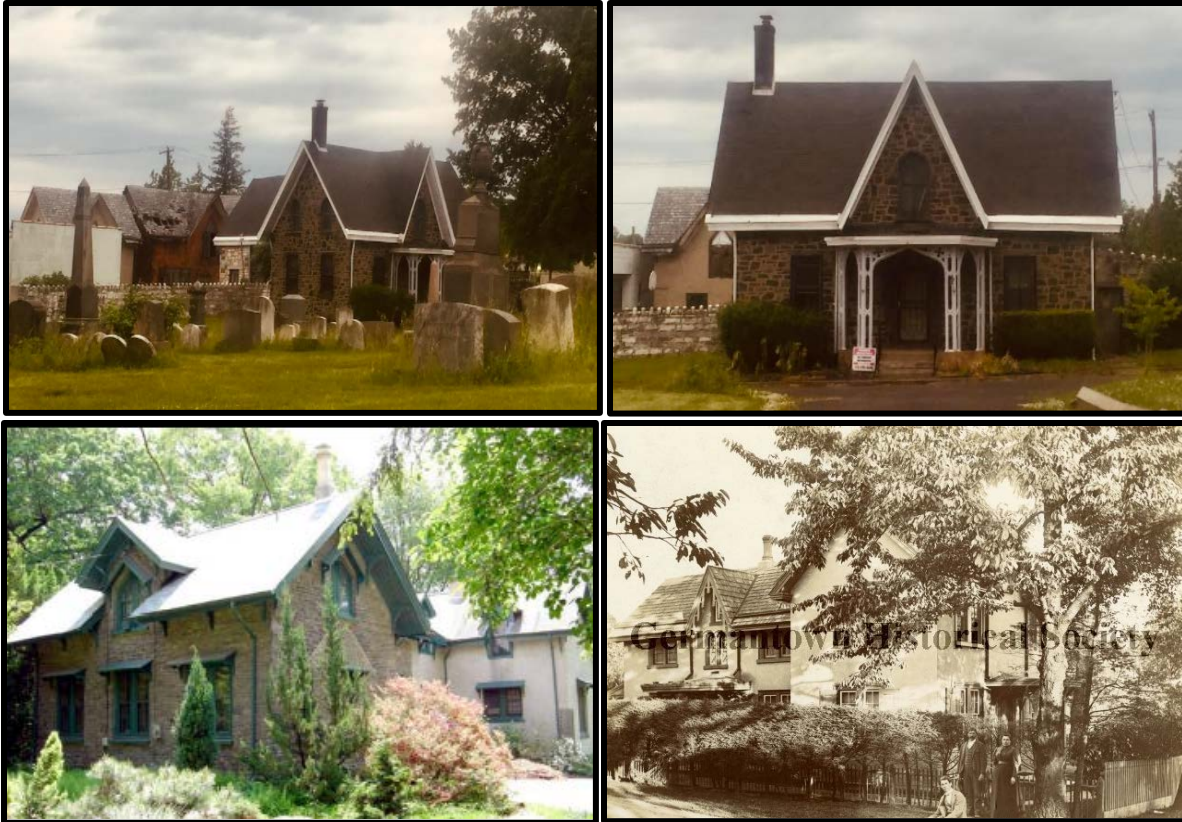
Figures 22. and 23. Top left and right: Keeper's Cottage at North Cedar Hill Cemetery in the Frankford neighborhood of Philadelphia. Source: Oscar Beisert, 2021. Figure 24. Bottom left: Awbury Servant's House (1852) at 6190 Ardleigh Street, East Germantown. Source: Awbury Historic District Nomination. Figure 25. Bottom right: Gardener's Cottage at Ravenhill, showing John McCleary, the gardener and his family. Source: Germantown Historical Society.
