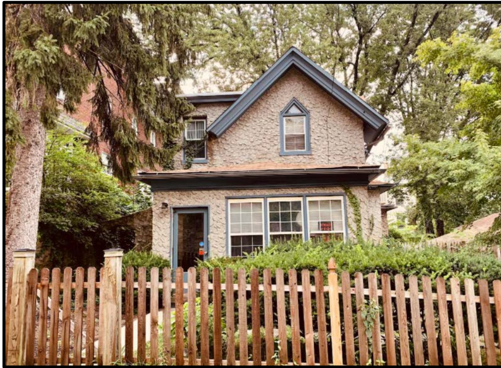
Figure 7. The northwest elevation. Source: Oscar Beisert, 2021.
