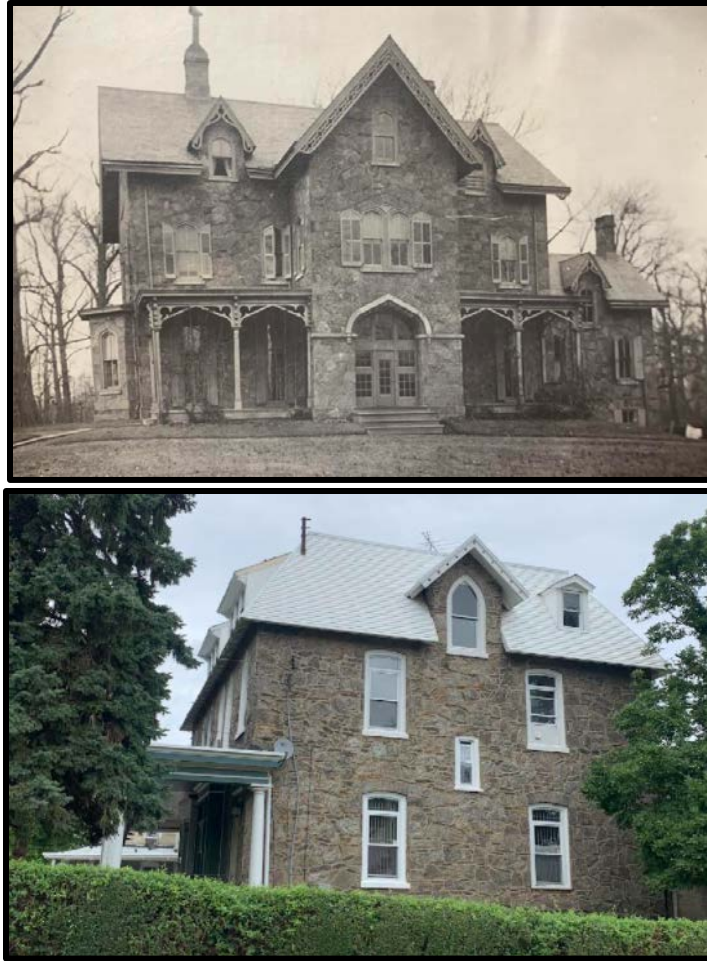
Figure 20. Top: A Gothic Revival house in Germantown, featuring a central gable, a Gothic Revival style doorway, and gable front wall dormers with barge board. Source: Germantown Historical Society. Figure 21. Bottom: The Thomas A. Gummey Twin at the southeast corner of High and Morton Streets in Germantown, featuring a gable front wall dormer, featuring a pointed arched opening. Source: Oscar Beisert, 2021.
