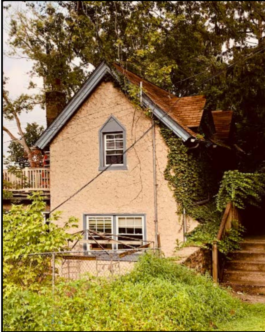
Figure 10. Looking northwest at the southeast elevation. Source: Oscar Beisert, 2021.
