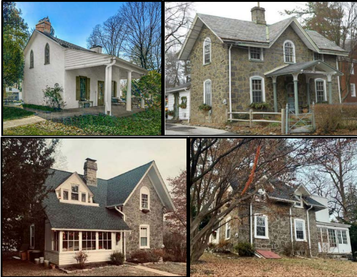
Similar examples of the Gothic Revival style employed in cottages that served larger estates in Philadelphia. Figure 26. Top left: A Keeper's Cottage (ca.1790, 1837, and 1880) of the Roxboro Estate, School House Lane, East Falls/Germantown. Source: www.estate.com . Figure 27. Top right: Stone Gothic Cottage (ca.1848-50) on Cherry Lane, officially 3000 W. School House Lane, East Falls/Germantown. Source: Nancy Pontone. Philadelphia Register of Historic Places Nomination: Stone Gothic Cottage on Cherry Lane, 3000 W. School House Lane . (Philadelphia: East Falls Historical Society, 2020). Figures 28. and 29. Bottom left and right: Views of the Gardner's Cottage at The Chestnuts aka Leighton Place, The Country Seat of David Scull, Jr. at 5848 City Avenue. Source: Oscar Beisert. Philadelphia Register of Historic Places Nomination: The Chestnuts aka Leighton Place, The Country Seat of David Scull, Jr., 5848 City Avenue, Overbrook, Philadelphia . (Philadelphia: Keeping Society of Philadelphia, 2020), 34.
