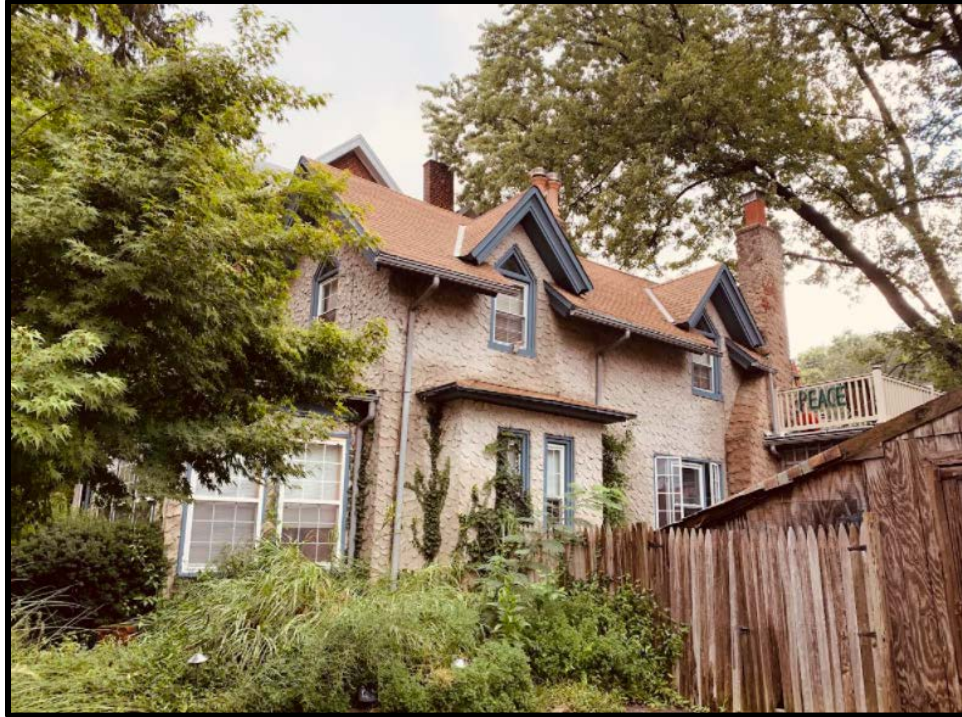
Figure 6. Looking east at the northwest and southwest elevations. Source: Oscar Beisert, 2021.
