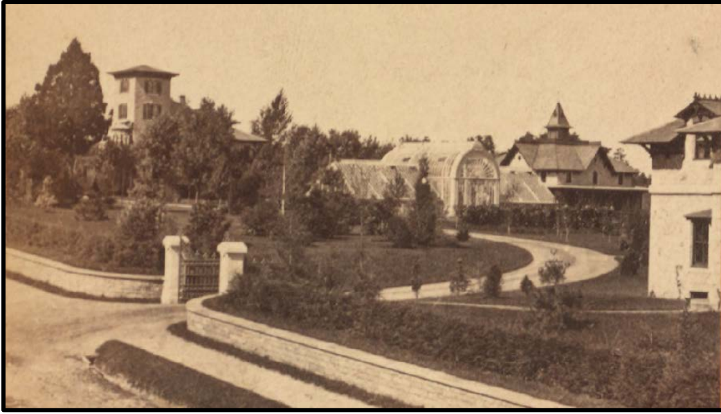
Figure 32. The Edward White Clark Estate at the southeast corner of School House Lane and Wissahickon Avenue, showing the ancillary buildings, which formed a distinctive historic landscape. Source: New York Public Library.
