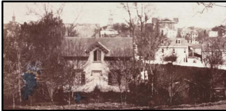
Figure 17. Taken in 1858, looking north, this photograph shows a small Gothic Revival style cottage in the rear of a lot along the east side of Germantown Avenue between E. Penn Street and Church Lane. Source: Philalandmarks.org.
