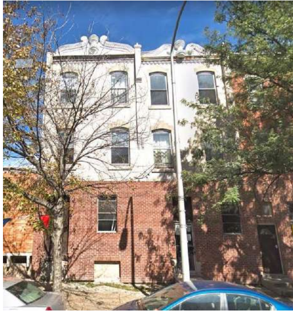
Example of 1.b.i: 1930-32 Christian Street is “Contributing” because the new brick façade occupies less than 50% of the original façade.
