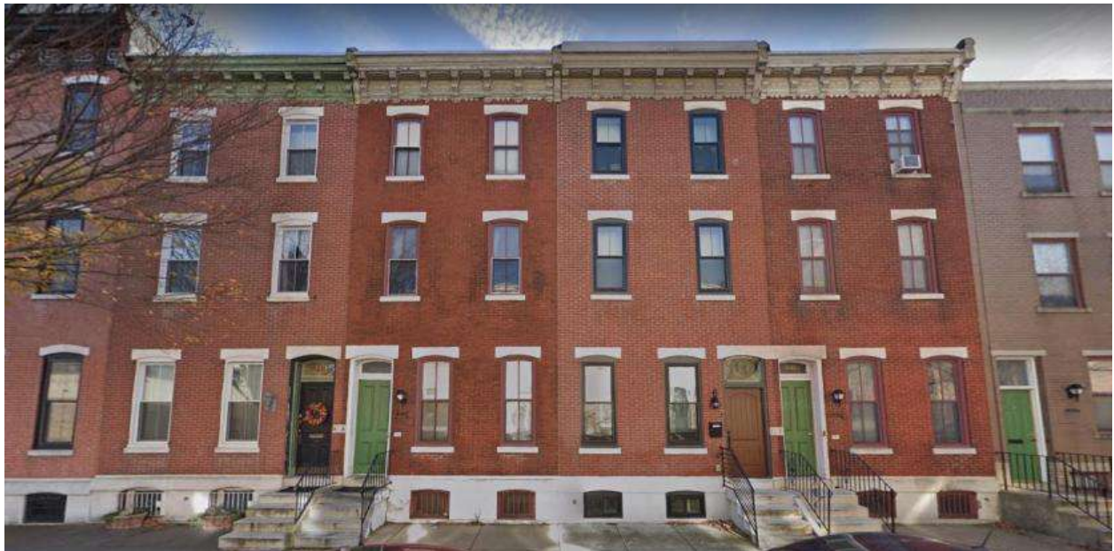
Figure 3. 1428-1434 (right to left) Christian Street. Note ABAB pattern, strong cornice, water table, and eyebrow lintels. 1430 Christian (second from left) retains curved top windows (image by Google Maps).
