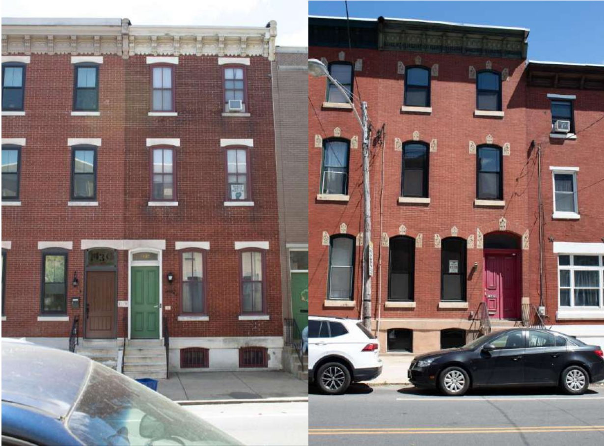
Figure 14b. (L) An example of an Italianate row house at 1432 Christian Street. (R) An example of a Néo-Grec row house at 1609 Christian Street. Both images from the inventory.
