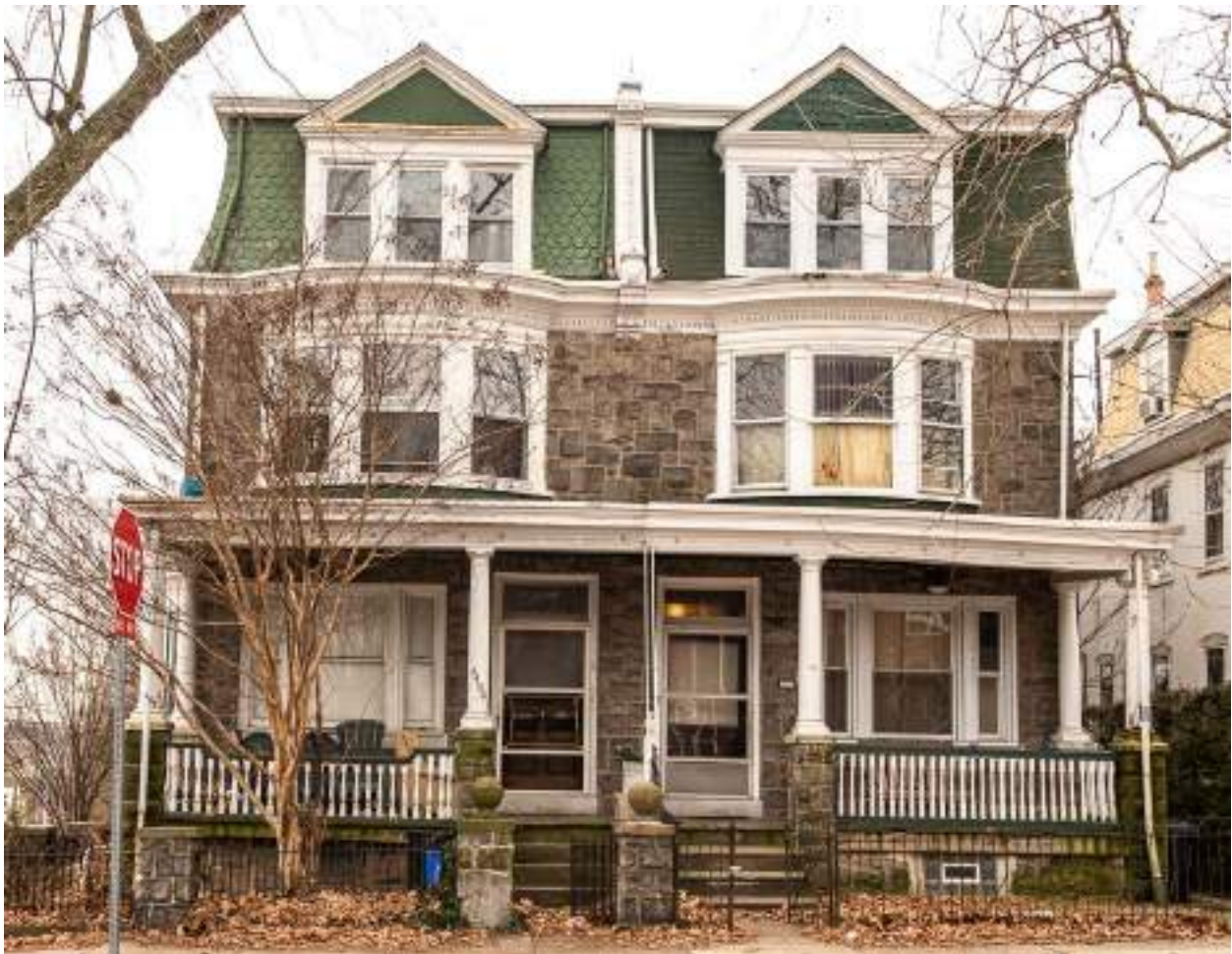
Figure 37: 4400 and 4402 Manayunk Avenue, constructed in 1896 by local contractor Walter Rowland, feature Second Empire mansard roofs but typical Colonial Revival details such as dentiled cornices, columned porches, bay and triple windows.
