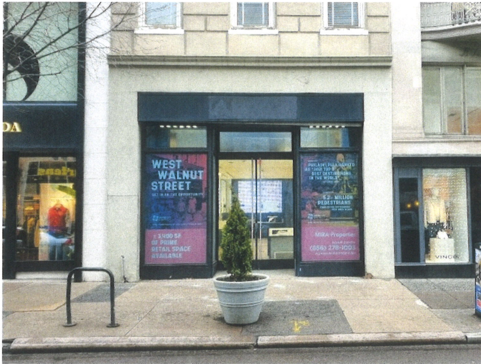
Close-up view of storefront
