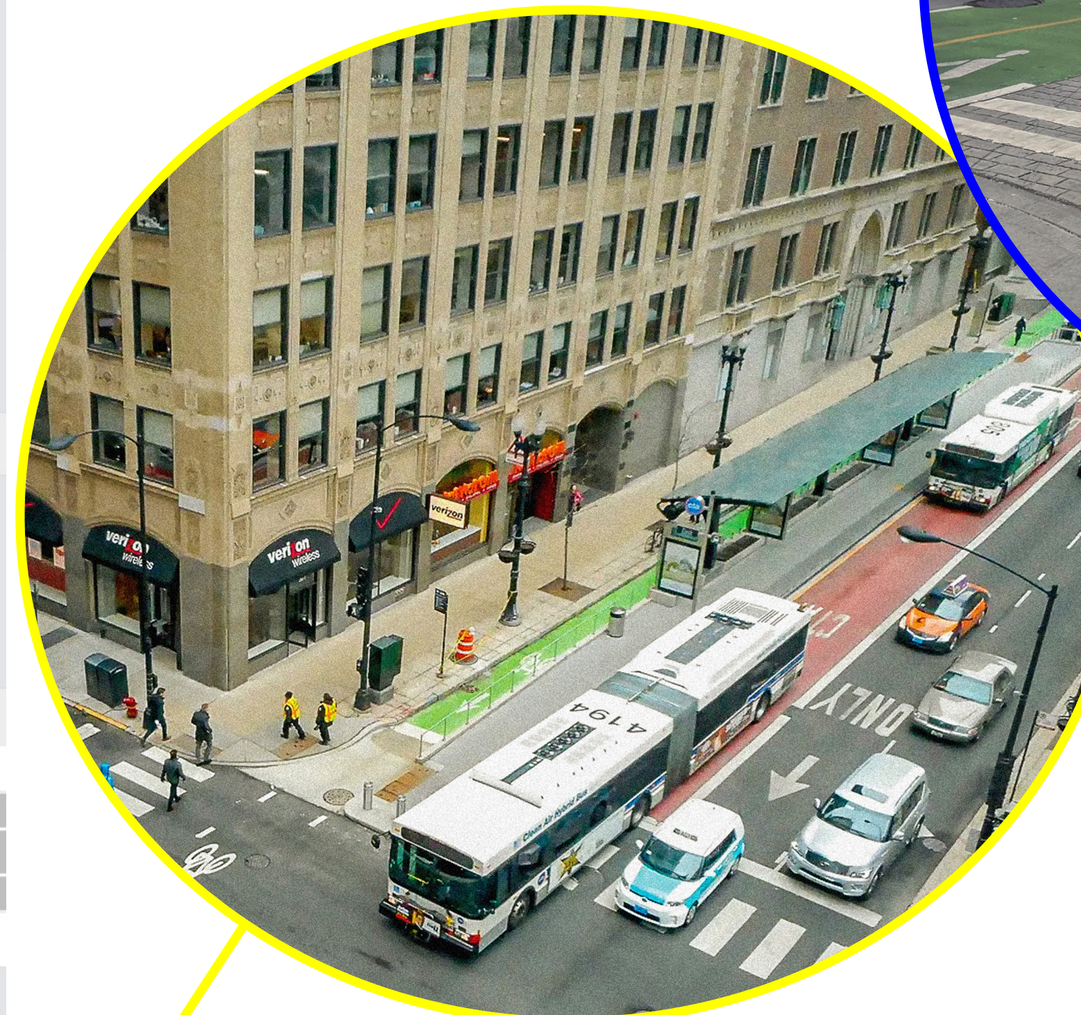
Bus Boarding Island
