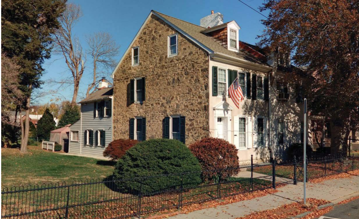
Figure 2: Side elevation of 8110 Frankford Avenue.
