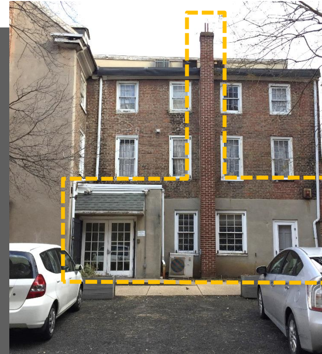
MODERN STUCCO, ENTRANCE BUMPOUT, CHIMNEY – Demolition of rear ell previously approved
