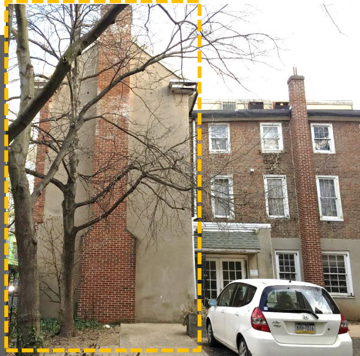
MODERN STUCCO, CHIMNEY (FORMER PARTY WALL) Demolition of c 1973 chimney previously approved
