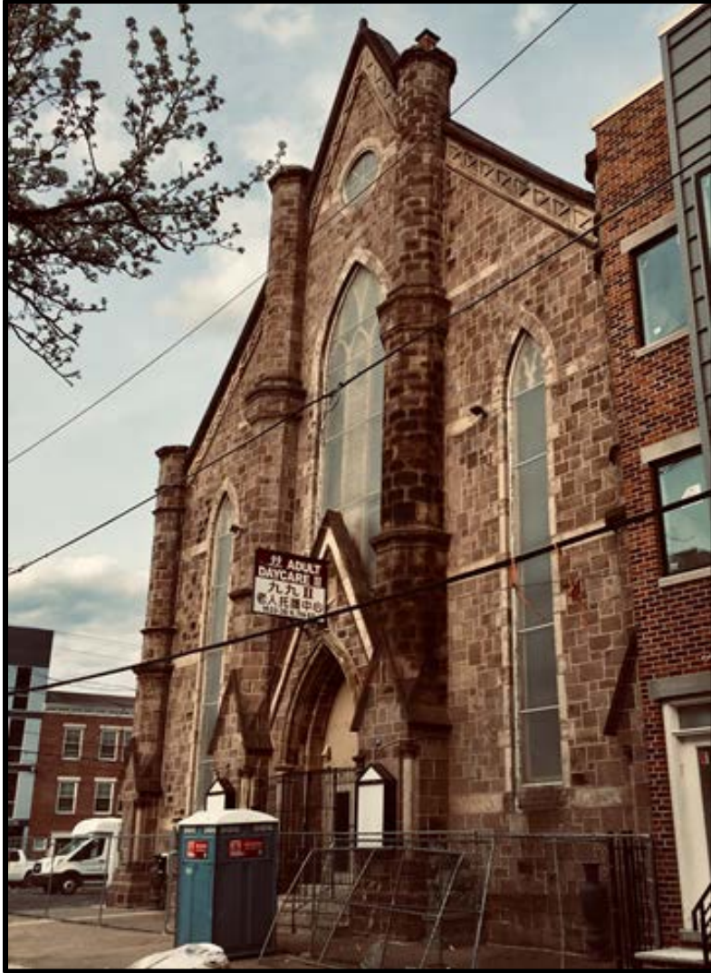
Figure 19. The primary (west) elevation of the subject property. Source: Oscar Beisert, 2019.
