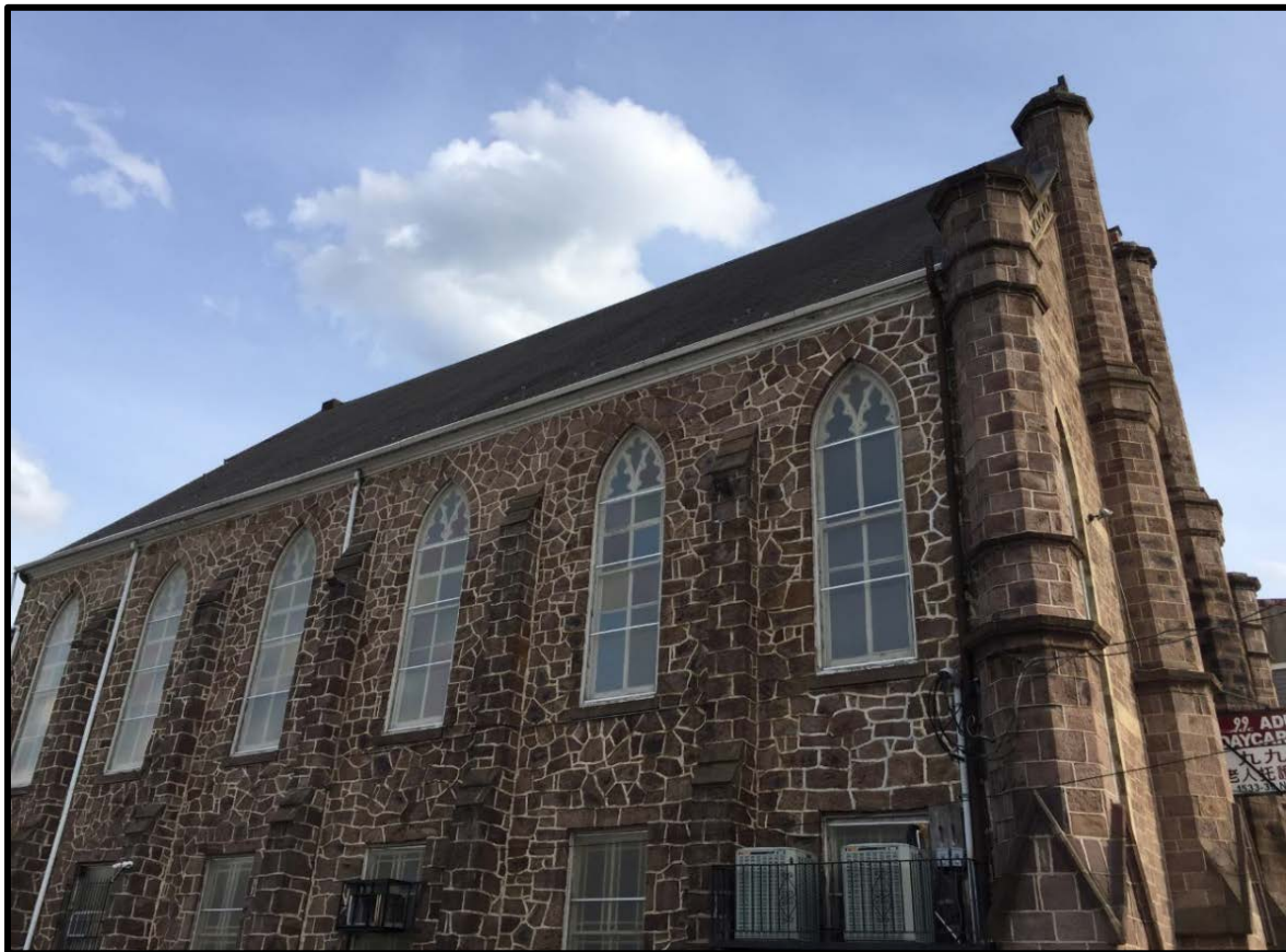
Figure 9. The side (north) elevation of the subject property. Source: Oscar Beisert, 2019.
