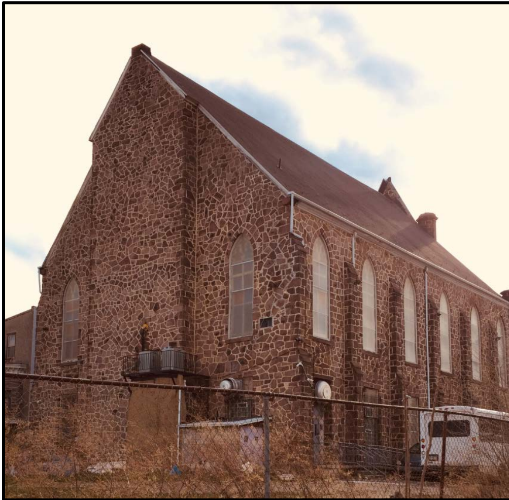
Figure 10. The rear (east) and side (north) elevations of the subject property. Source: Oscar Beisert, 2019.
