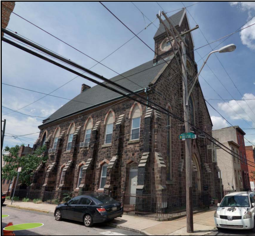
Figure 16. St. John German Evangelical Church located at 516 Wharton Street, designed by Samuel Sloan and constructed in 1873. Source: Cyclomedia, 2018.
