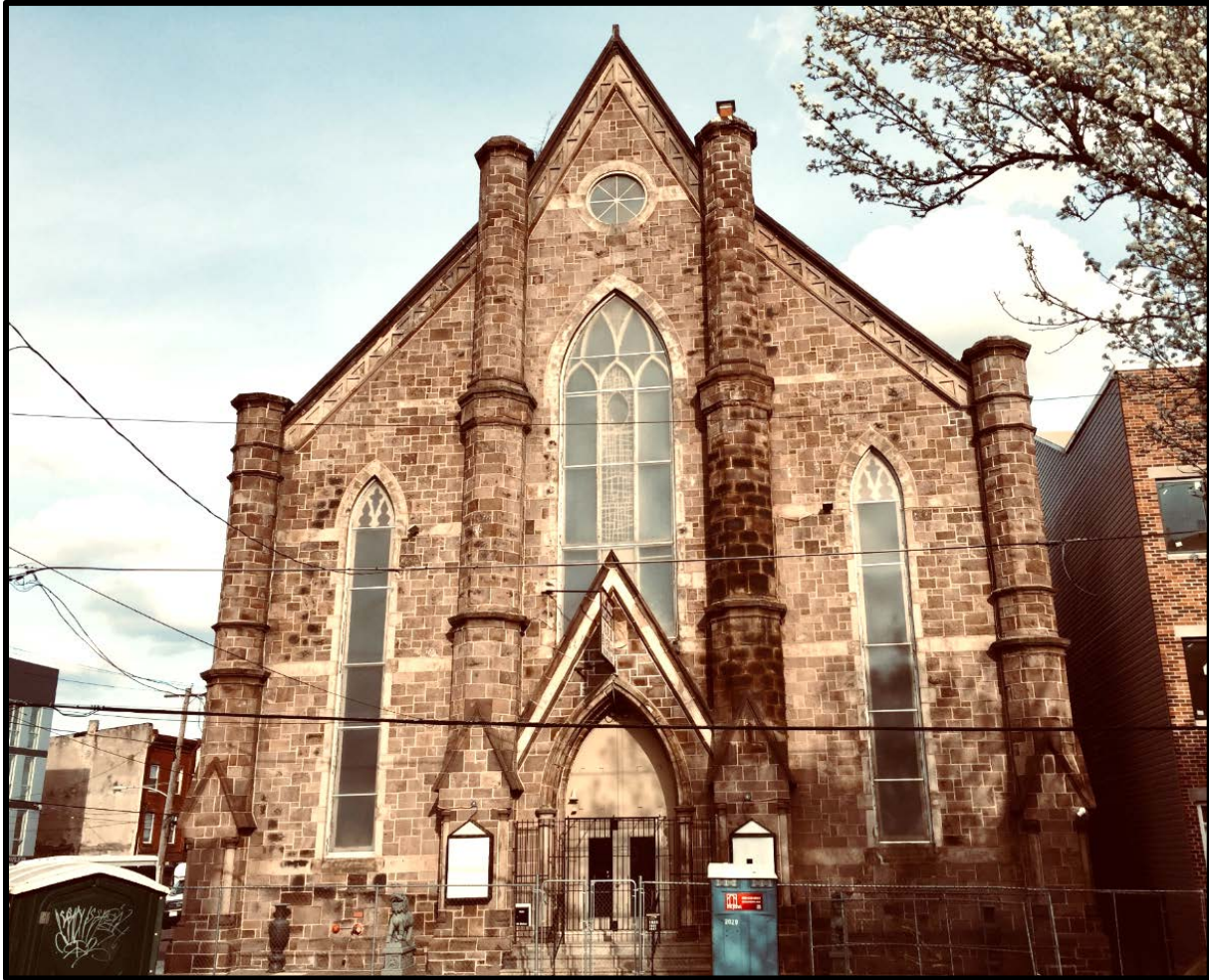
Figure 1. Looking south at the primary (west) elevation of the subject property. Source: Oscar Beisert, 2019.
