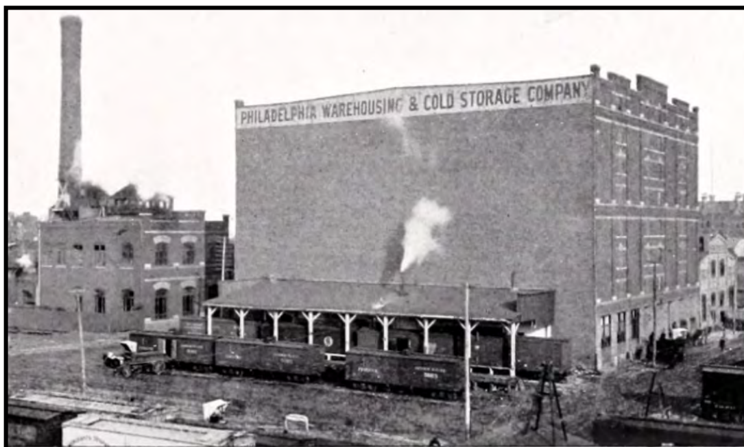
Figure 23. An early photograph of Warehouse A, the Ice Machine House, and the Boiler House and Stack of the Philadelphia Warehousing and Cold Storage Company, as shown in a national book on such facilities. Source: Cold storage and freezing warehouses equipped the Pontifex-Hendrick Refrigeration System. (The Hendrick Manufacturing Co., 1897).
