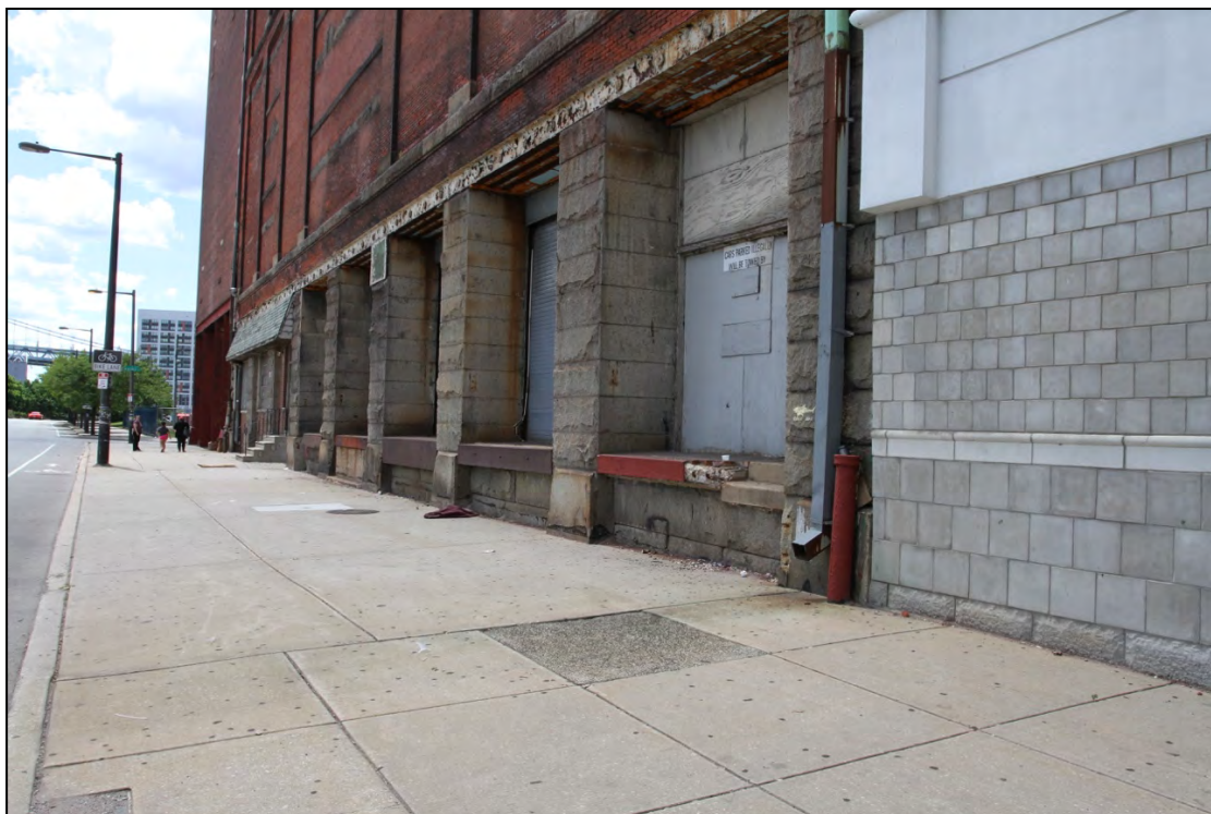
Figure 13. Raking view of the ground floor on the east façade of Warehouse A of the Philadelphia Warehousing & Cold Storage Company industrial complex. Note the ashlar, quarry-faced masonry that anchors the warehouse into its site. Source: Allee Davis, June 2019.
