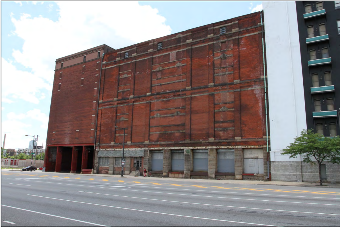
Figure 5. The east façade of both Warehouses A (right) and B (left) of the Philadelphia Warehousing & Cold Storage Company industrial complex. Note the colossal pilasters and stringcourses that organize the symmetrical fenestration patter. Source: Allee Davis, June 2019.
