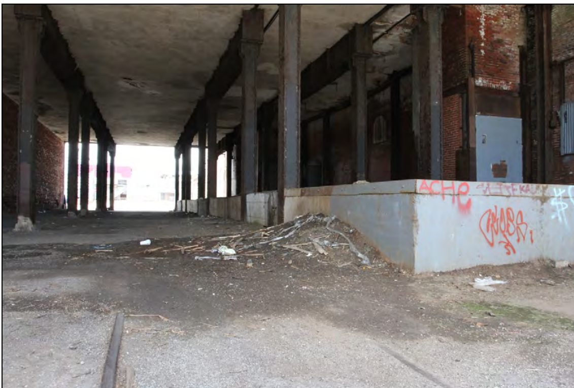
Figure 14. View of the throughway and extant rail siding that historically facilitated the passage of railcars for shipping and receiving in support of the company's operations. Source: Allee Davis, June 2019
