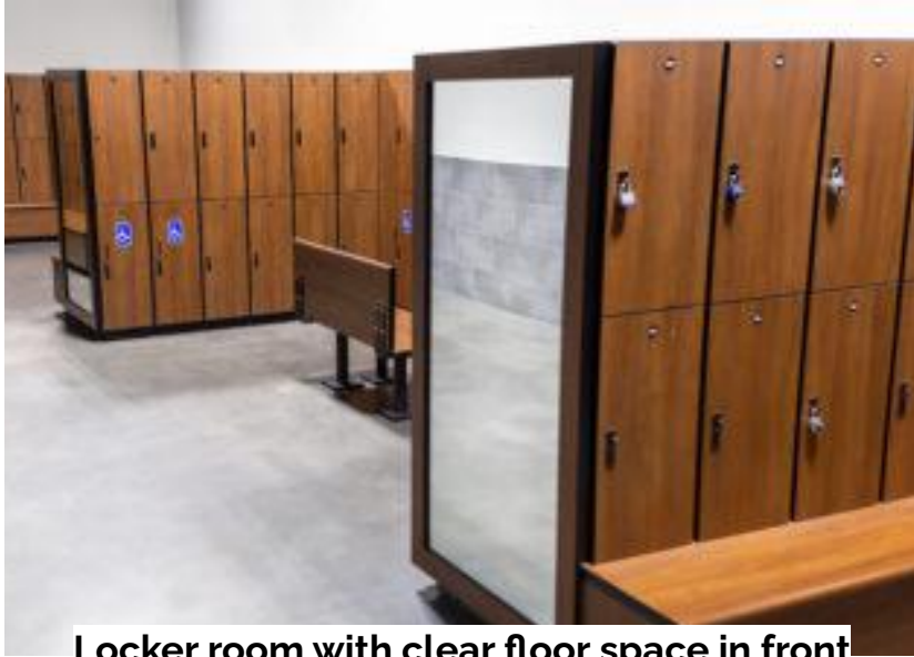
Locker room with clear floor space in front of lockers and back-supporting benches
